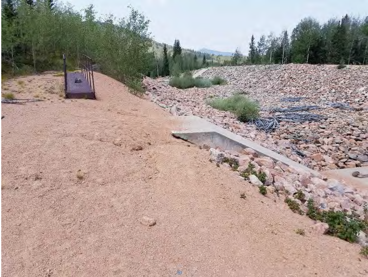
47_Left side spillway control section
