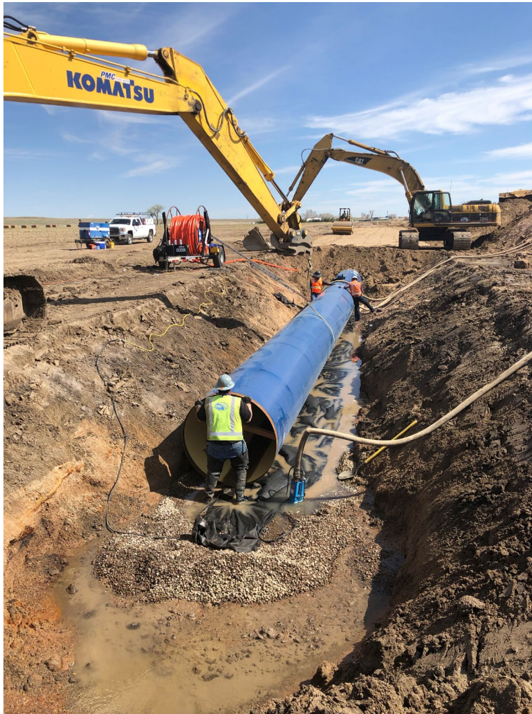
Figure 2 – Installation of 54” Walker Pipeline
