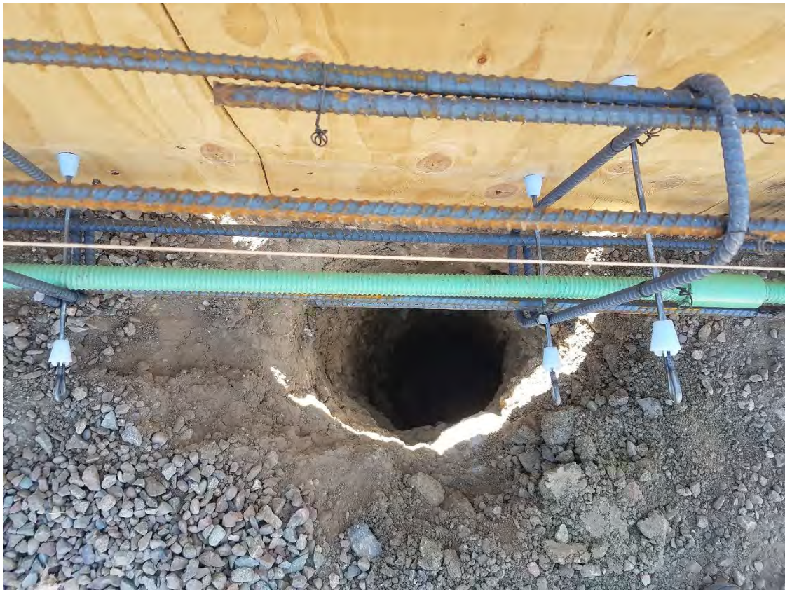
Photo 7 Pier holes dug; rebar placed in holes (not shown here)
