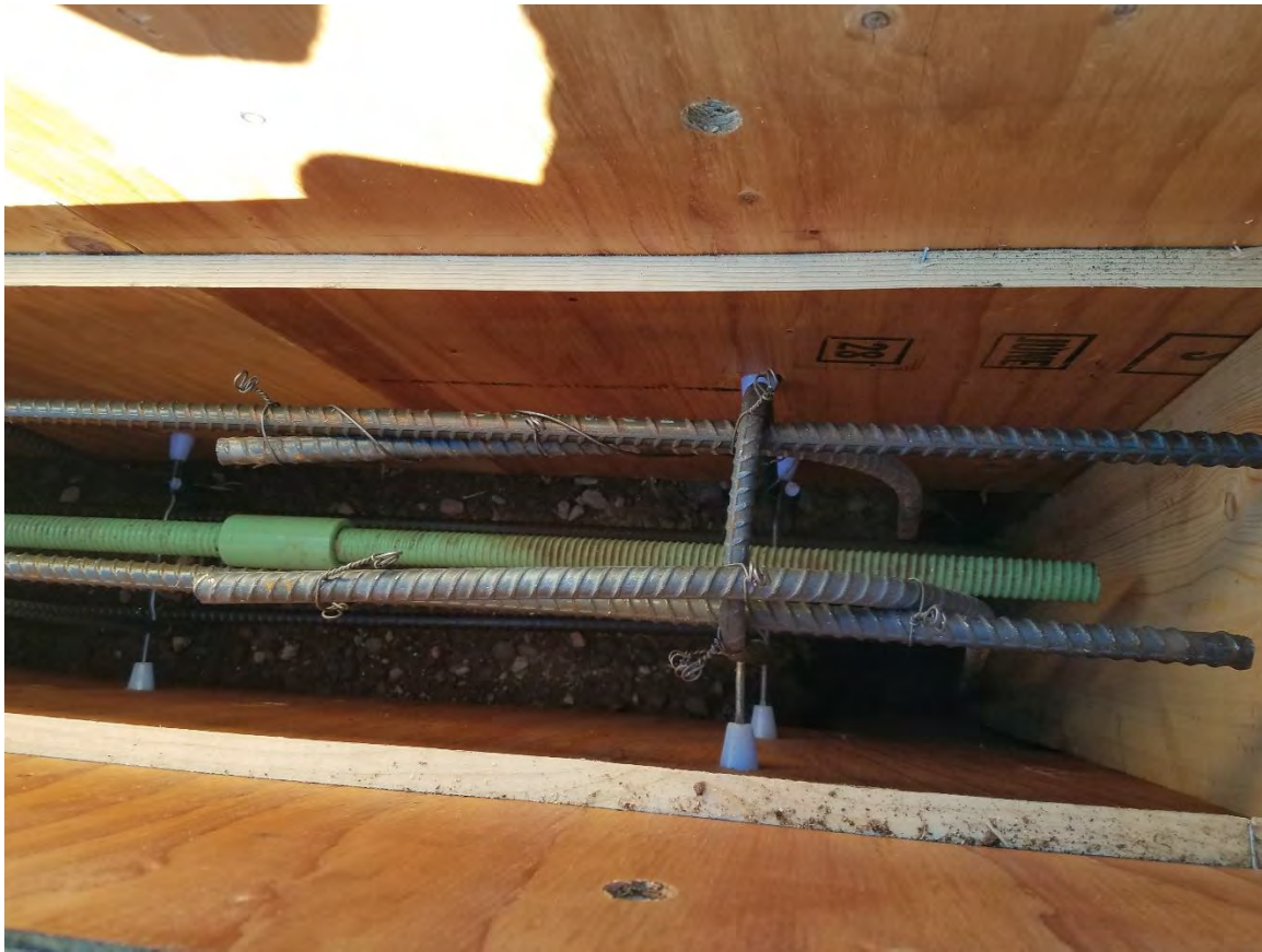
Photo 2 Rebar and tension rod in place over pier
