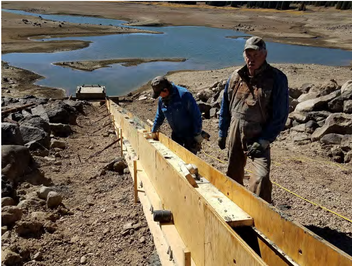
Photo 6 Waiting to begin Truck #2 pour at 1:37 pm
