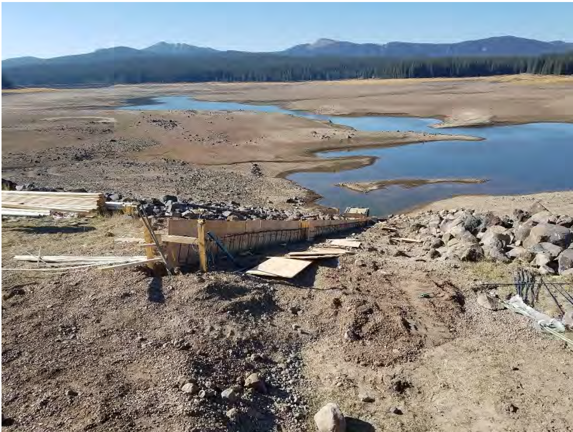
Photo 9 Gauge beam work site from top of dam
