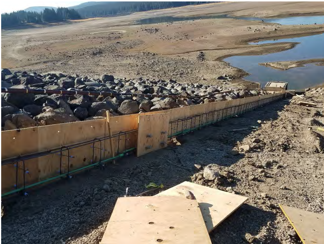
Photo 3 Longitudinal rebar in place top & bottom
