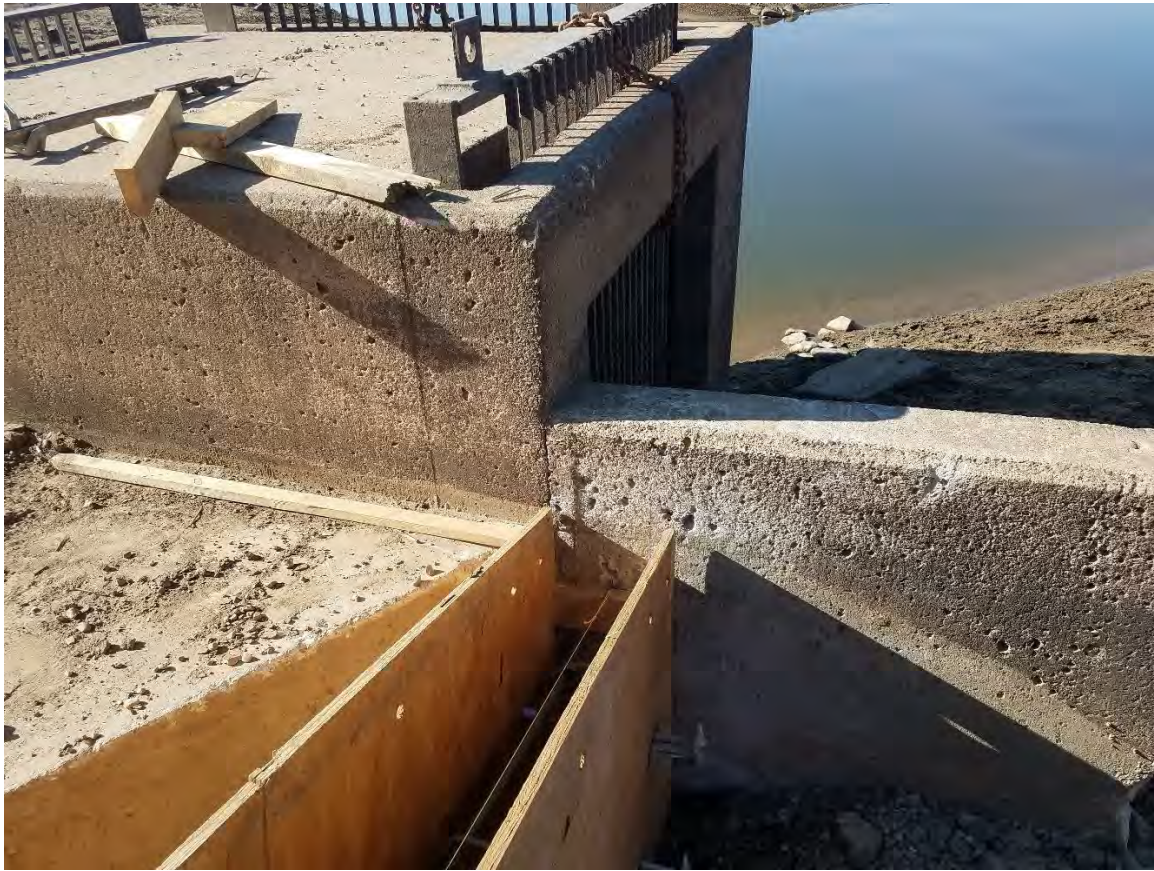
Photo 4 Beam meets existing inlet structure
