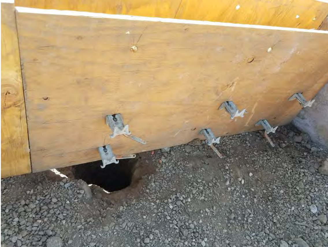
Photo 8 Form locks in place at bottom of beam
