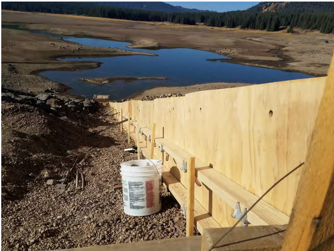
Photo 1 South wall forms loosely set
