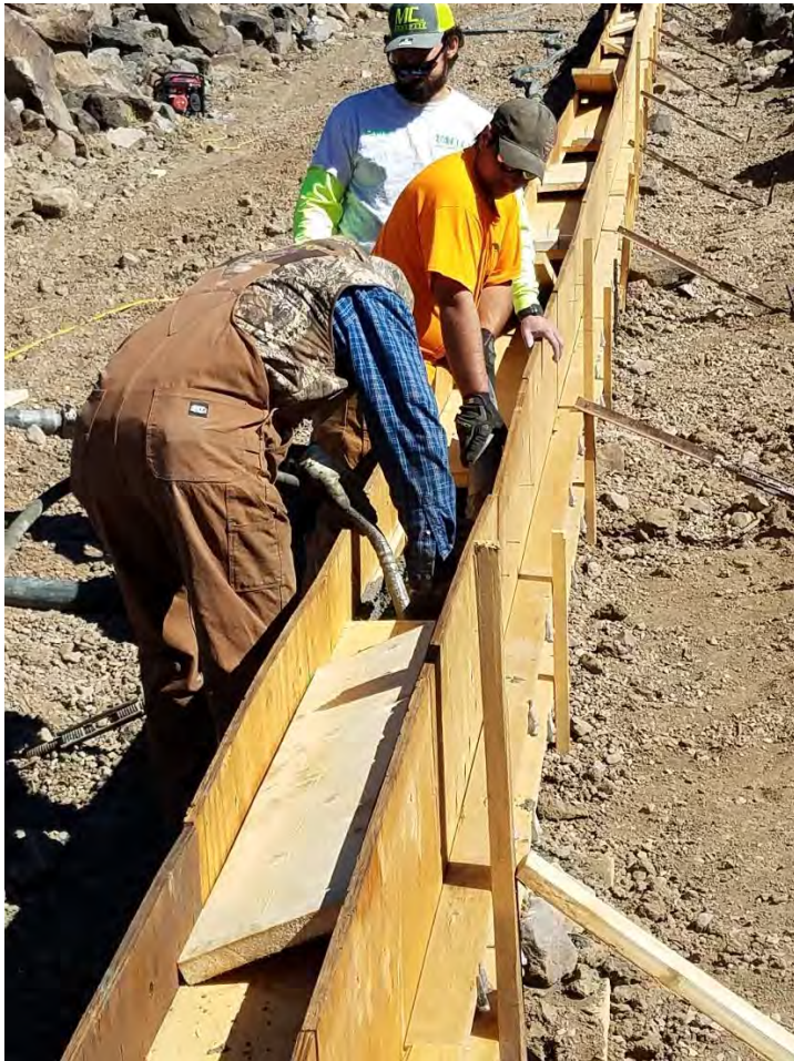
Photo 5 Vibrating to fill under form cap
