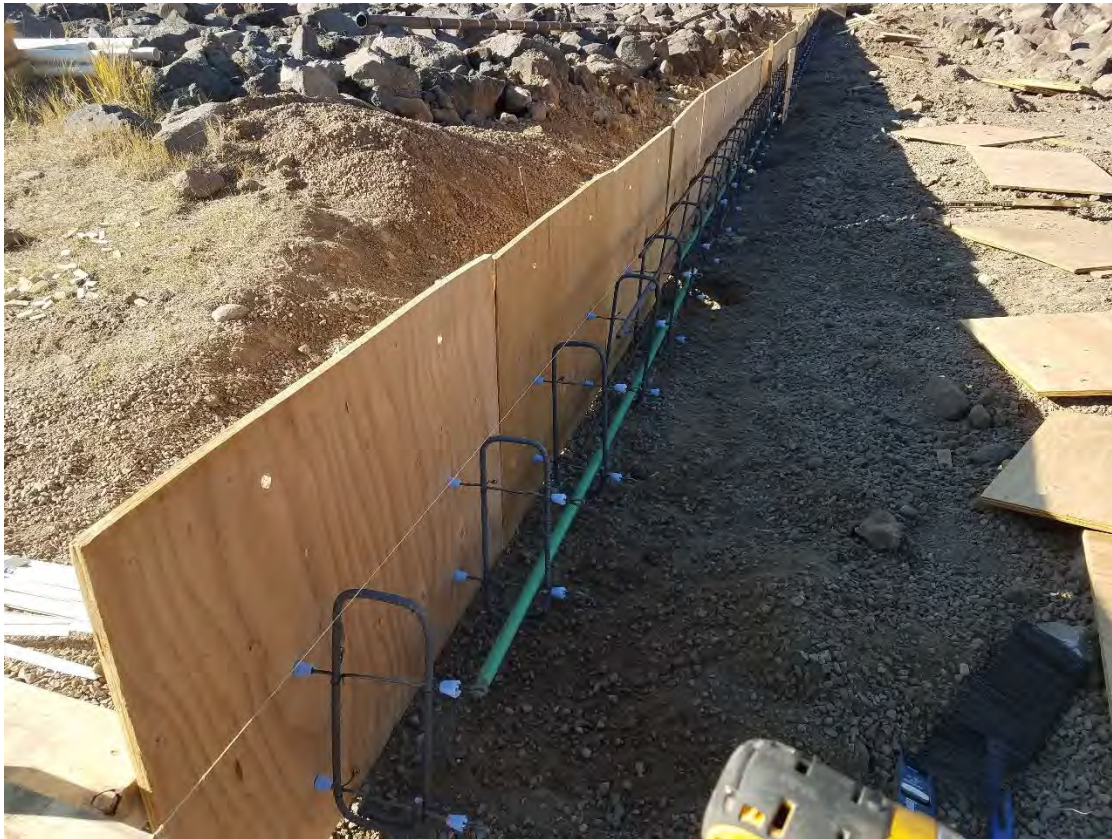
Photo 2 Rebar stirrups with tension rod loosely placed
