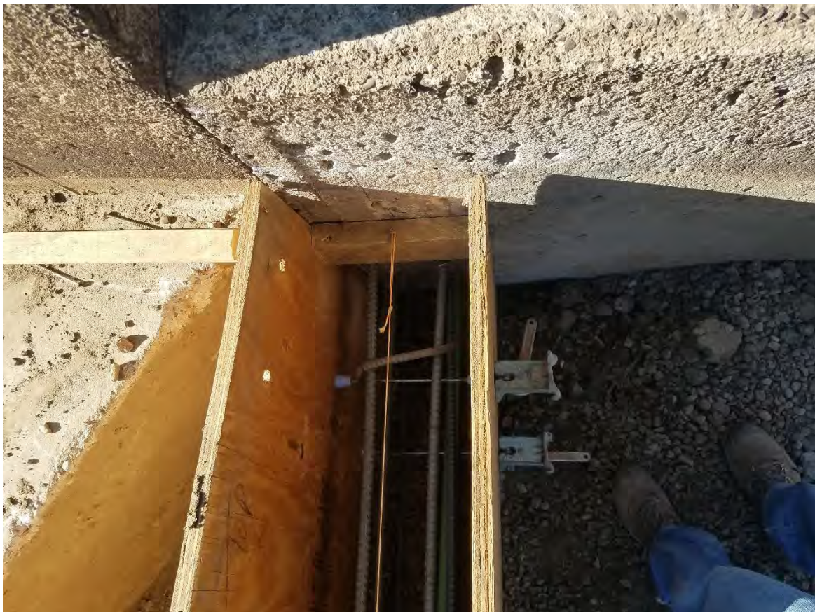
Photo 5 Six pins grouted into existing concrete for tie in
