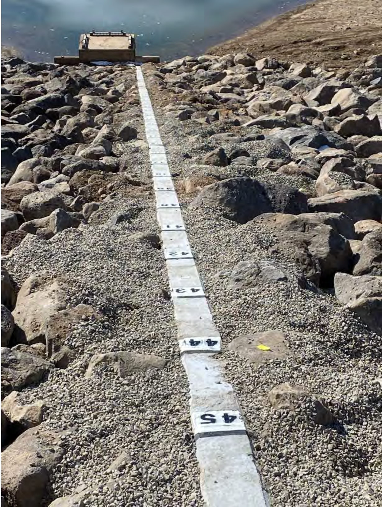
FIGURE 1 COMPLETED OVERLAND RESERVOIR GRADE BEAM
