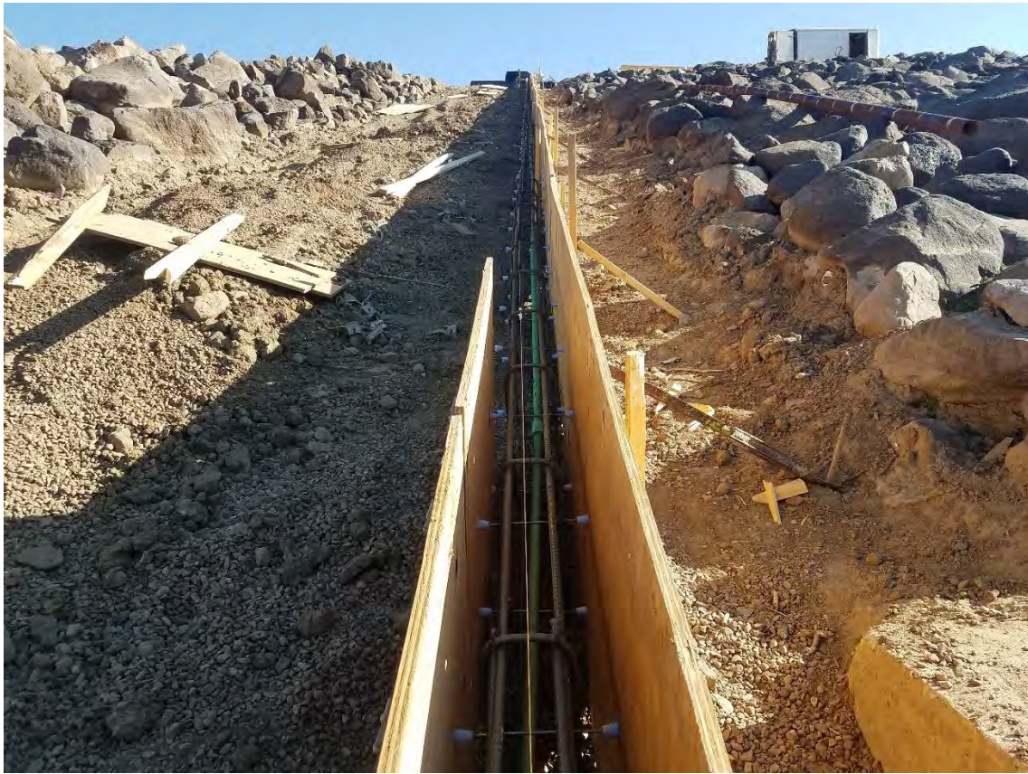
Photo 6 Beam rising from inlet
