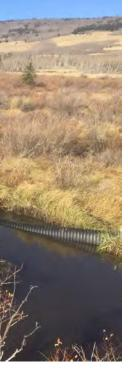
← Lower of two pond levelers. For most of the season when streamflow is low, the upstream leveler (background) carries full flow. The secondary downstream leveler (foreground) kicks in when streamflow is high.
