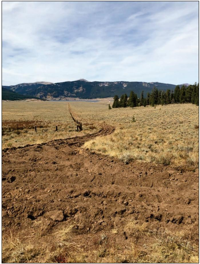
Photos above are before and after of a long illegal route we ripped with a dozer. We also seeded before and after the dozer with a native 4 seed mix. Photos below are also in Taylor Park, near the photo location above. This was a steep hill and we ripped, seeded, and pulled in slash to slow erosion. We also pulled up the sediment plum at the base which was washing into a fen downstream.
