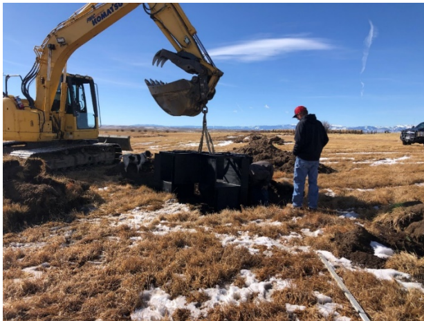
Figure 8. Custom T-box being installed at Sherman Creek Ranch. The structure will allow irrigation
