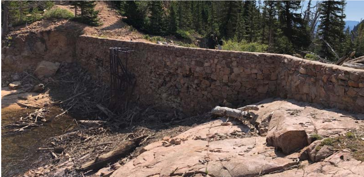
Figure 1. Dam face of Aqua Fria Reservoir and dilapidated headgates prior to completion of project. All debris has since been removed. The dam was hand-laid in ~1940 and the water irrigates over 500 acres of wet meadow habitat in hay production.
