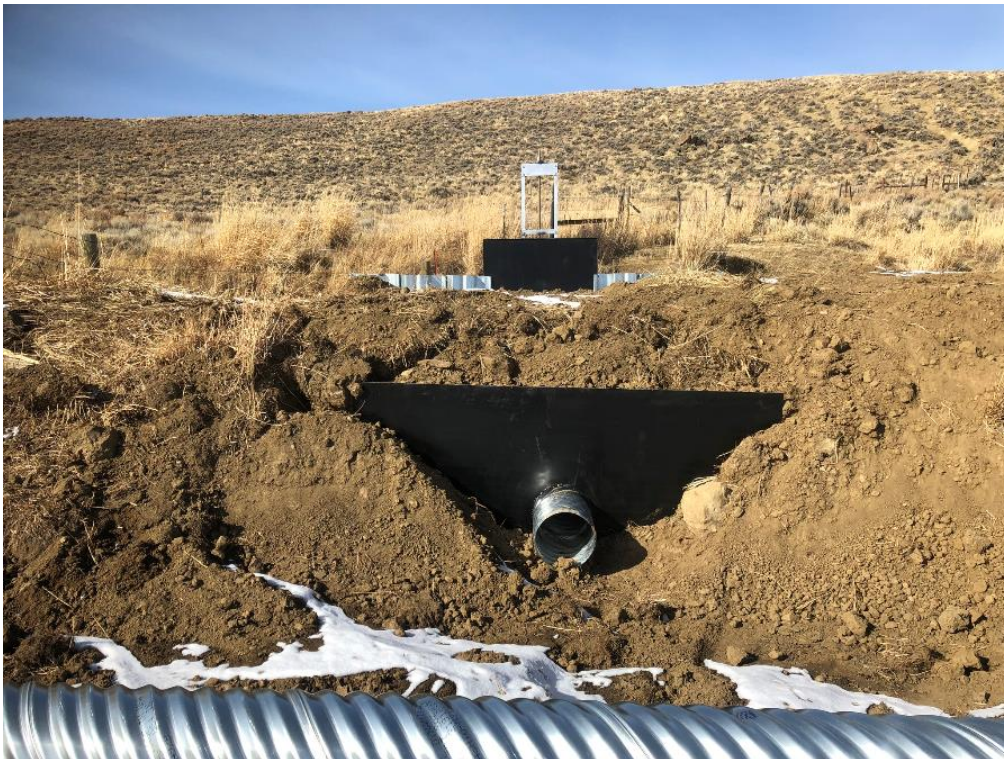
Figure 7. New custom headgate with supporting infrastructure installed at Russell Ranch.
