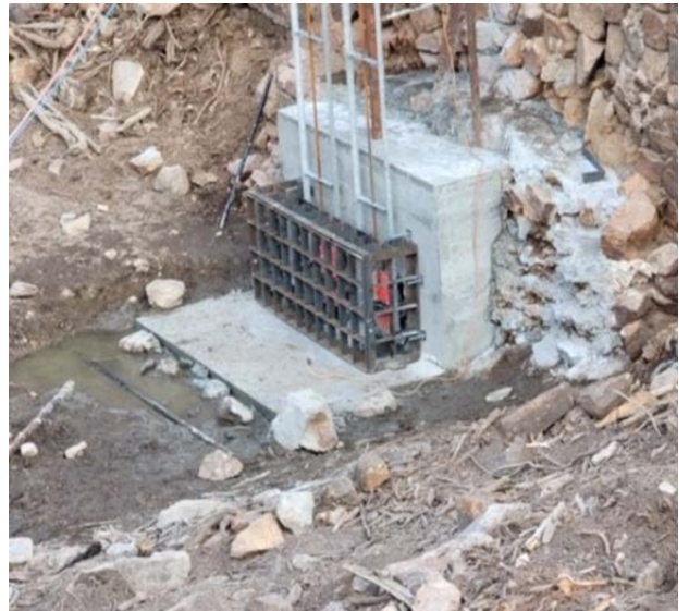
Figure 4. Newly installed headgates and debris curtain at the outlet of Aqua Fria Reservoir.
