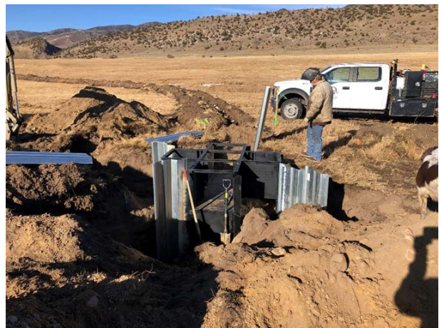
Figure 9. Custom T-box being installed with new ditching at Sherman Creek Ranch.
