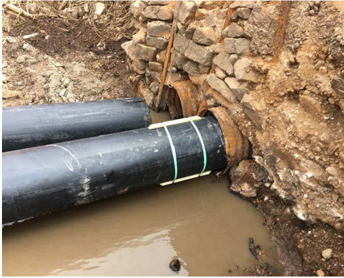
Figure 3. Installation of PVC inserts into dilapidated Corrugated Metal Pipe (CMP).
