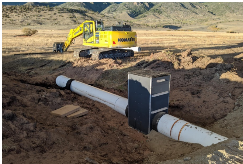
Figure 10. Installation of one of the Agri Drain inline stop log water control structures installed at Sherman Creek Ranch.
