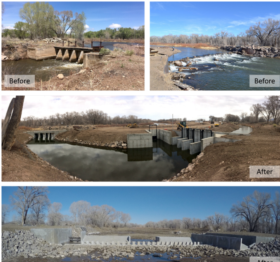
Figure 4. Before and after pictures of the Consolidated headgates and diversion dam.
