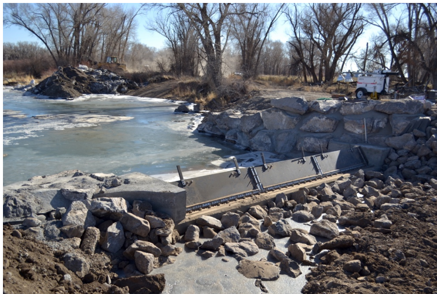
Figure 8. Obermeyer gate installed in the Centennial diversion dam.
