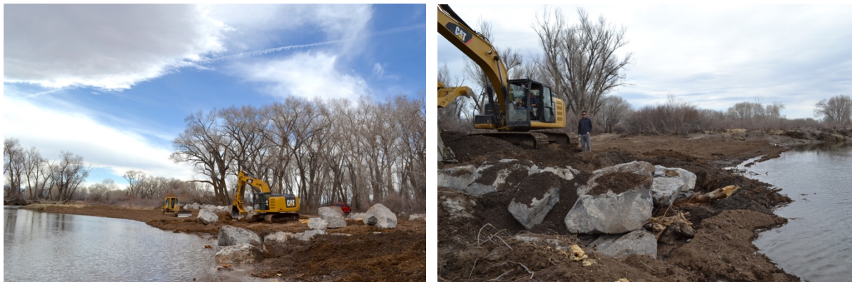
Figure 6. Streambank stabilization downstream of the San Luis Valley Canal Headgate.
