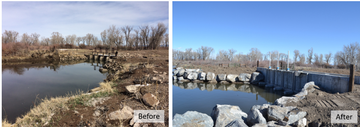
Figure 5. Before and after pictures of the San Luis Valley Canal headgate.
