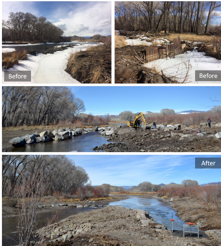
Figure 3. Top Left: Old diversion structure. Top Right: Old headgate structure. Middle: Placing rocks for the new diversion dam. Bottom: Completed concrete diversion structure, headgate, and trash deflector.
