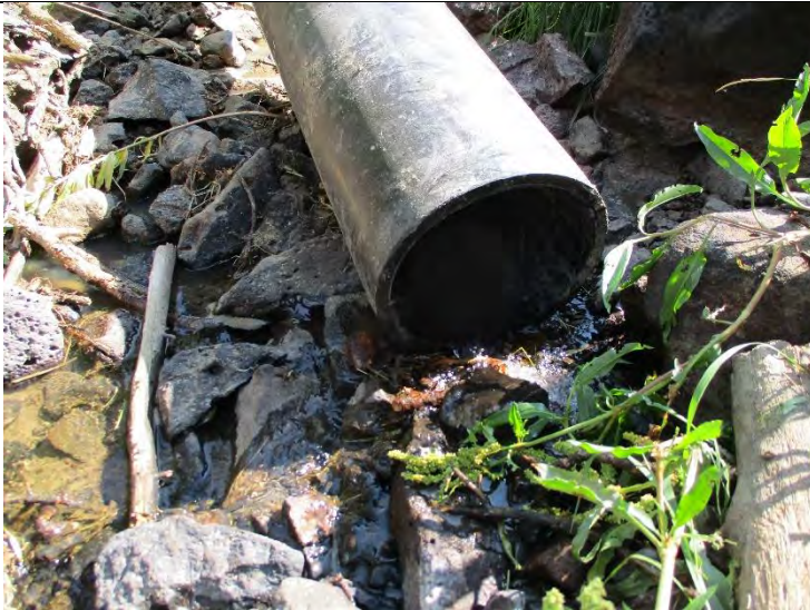
Photo 9. Flow depth of less than 0.5-inch conveyed by bypass pipe
