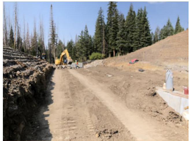
Photo 4. View looking south at the outlet channel on 9/18/20. Backfill is approximately at the top of the outlet pipe concrete encasement.
