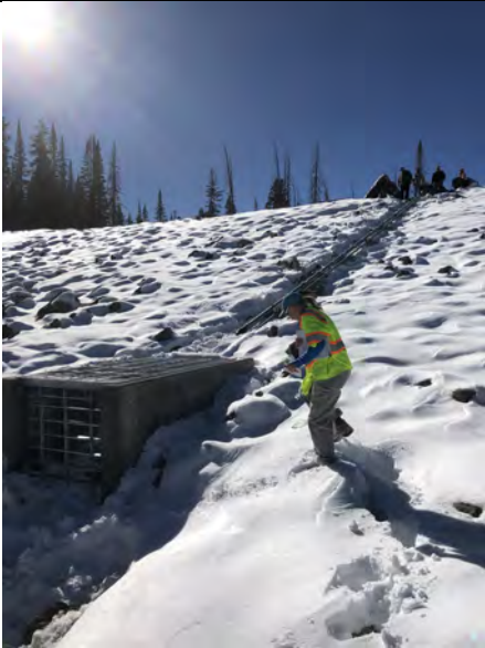
Photo 1. View of inlet structure looking up the upstream dam face. Gate stem is visible in the upper portion of the photo
