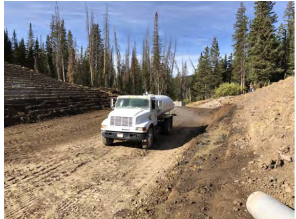
Photo 2. View looking south (downstream) at water truck moisture conditioning the subgrade prior to material placement.
