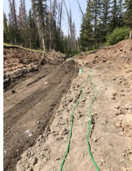
Photo 4. View looking south towards outlet of subgrade after proof-roll test.
