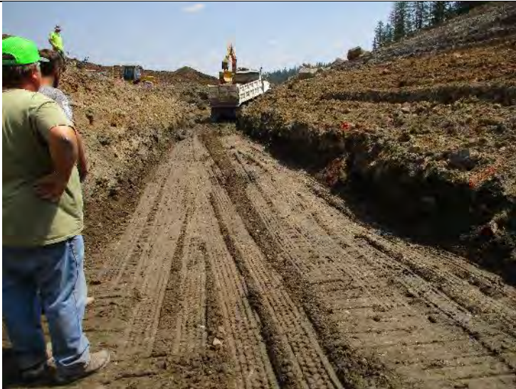
Photo 9. Kenworth loaded dump truck exits the outlet trench (looking upstream), following second proof roll.
