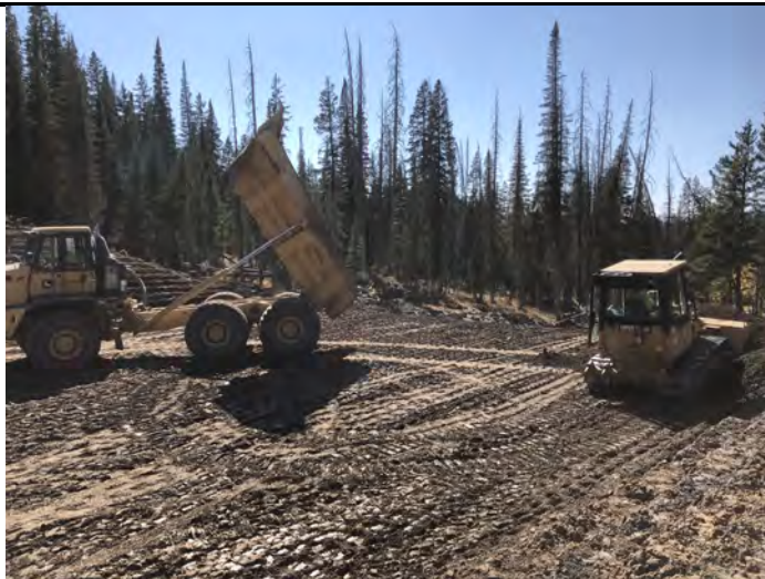
Photo 3. View of embankment material being dumped prior to spreading by D5 dozer
