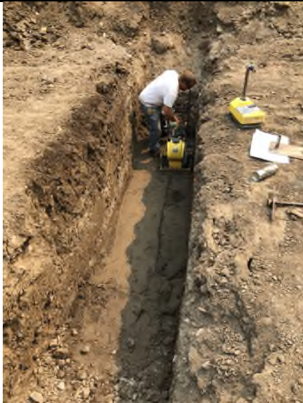
Photo 3. View looking east at sand diaphragm test section.
