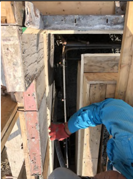
Photo 3. Close-up of inlet wall reinforcement during concrete placement on 9/18/20.
