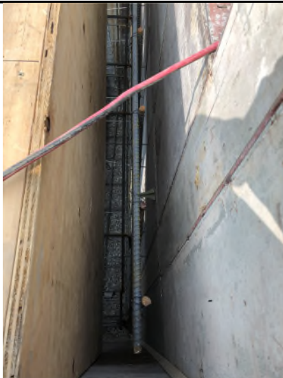
Photo 3. Close-up of inlet wall reinforcement. 2-inch wall chairs were installed prior to placement on the 18 th to provide required separation
