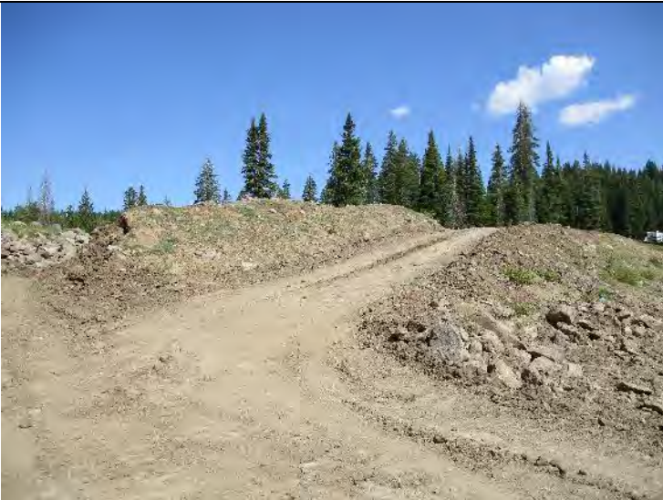
Photo 13. Material from the old breach (completed in 2018)
