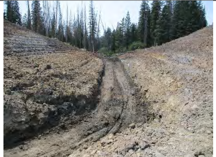
Photo 10. Foreground is the location of dump truck in previous photo, the approximate location of the intake structure (additional excavation needed) and the grade break/base of the equipment access into the outlet trench.
