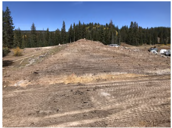
Photo 4. View looking west across the outlet channel embankment.
