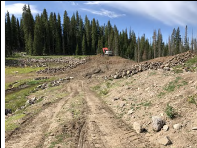
Photo 1. View looking east at existing breach excavation on July 16, 2020.
