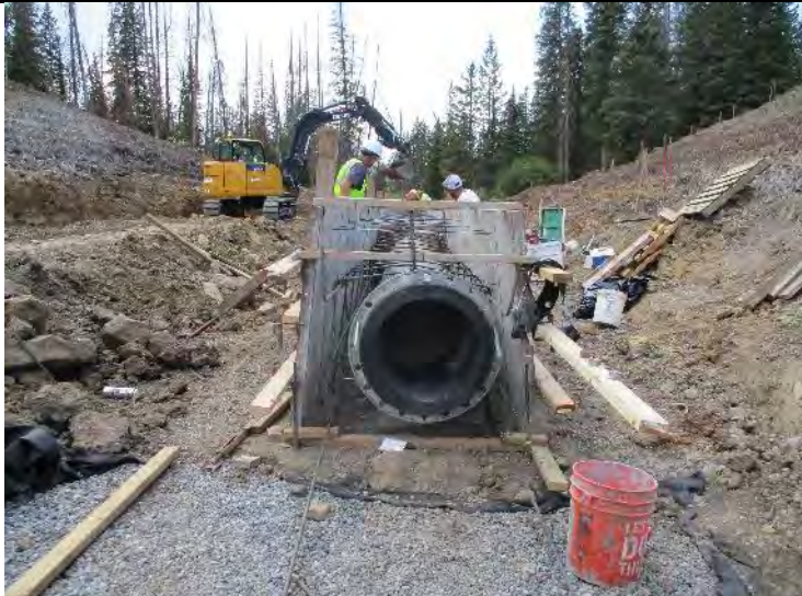
Photo 2. Inlet side. Con-Sy is awaiting an appropriately sized gasket to be delivered to the site.
