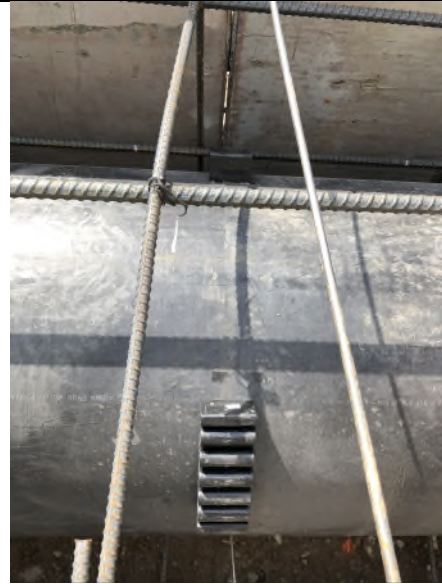
Photo 2. Closeup of fused HDPE flex restraint installed at STA 1+60 per plans.
