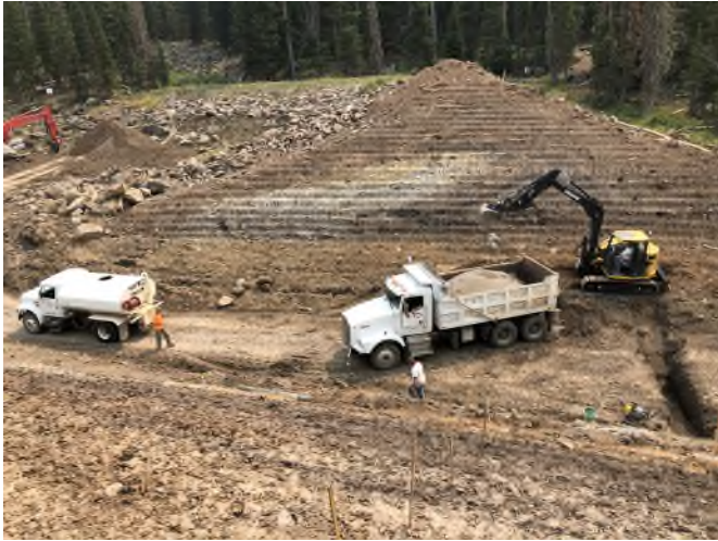
Photo 1. View looking east at sand diaphragm trench at STA 1+20 on 8/19/20. Note water truck dump truck of clean sand and excavator used to place the sand material.
