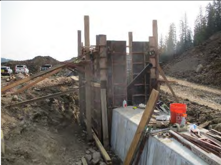
Photo 7. Exterior view of formwork.
