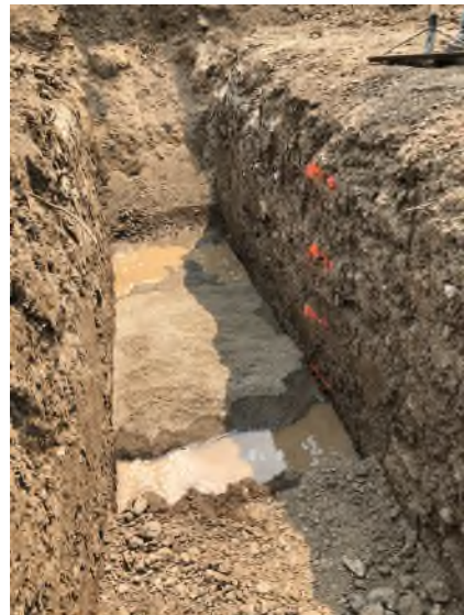
Photo 4. View looking east at initial test section which was too wet for compliant filter sand installation and which was subsequently removed prior to Test #2.
