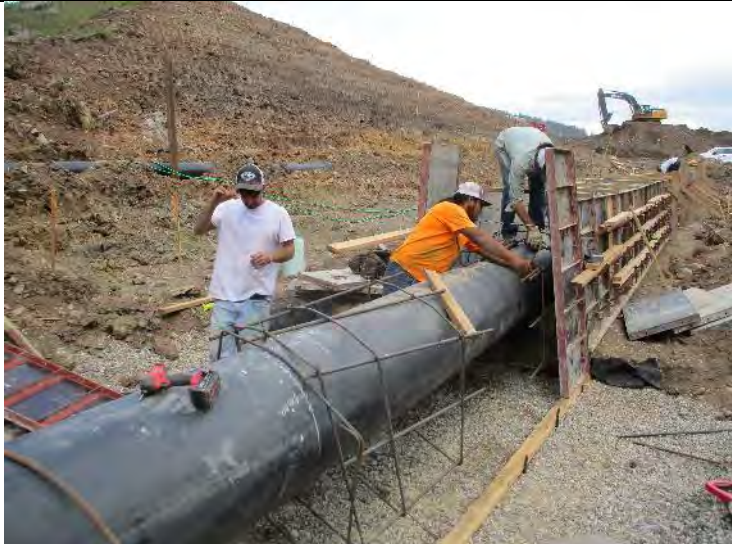
Photo 4. Placing steel at the terminal end of the pipe.
