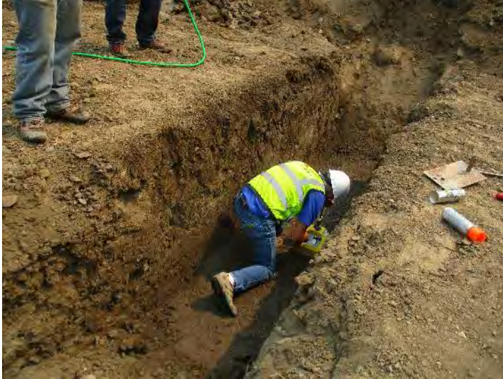
Photo 5. Nuclear gauge testing.
