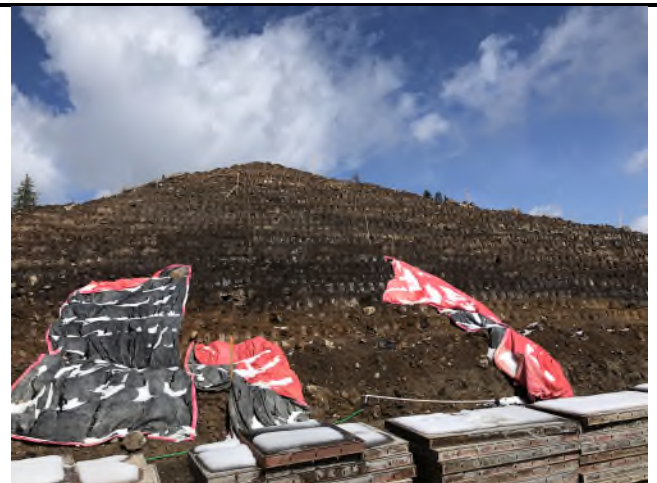
Photo 4. View of concrete blankets used to protect outlet formwork from rain and snow. Note dark areas of the embankment from precipitation events on 9/9 and 9/10.
