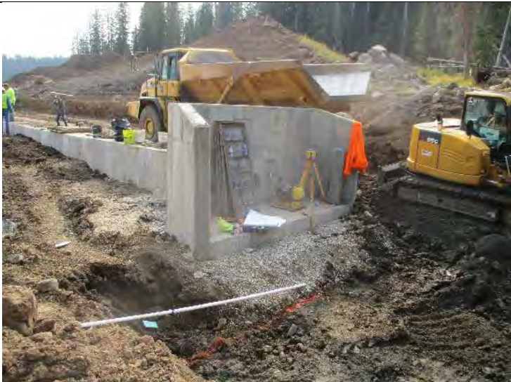
Photo 9. View of the outlet terminal headwall.
