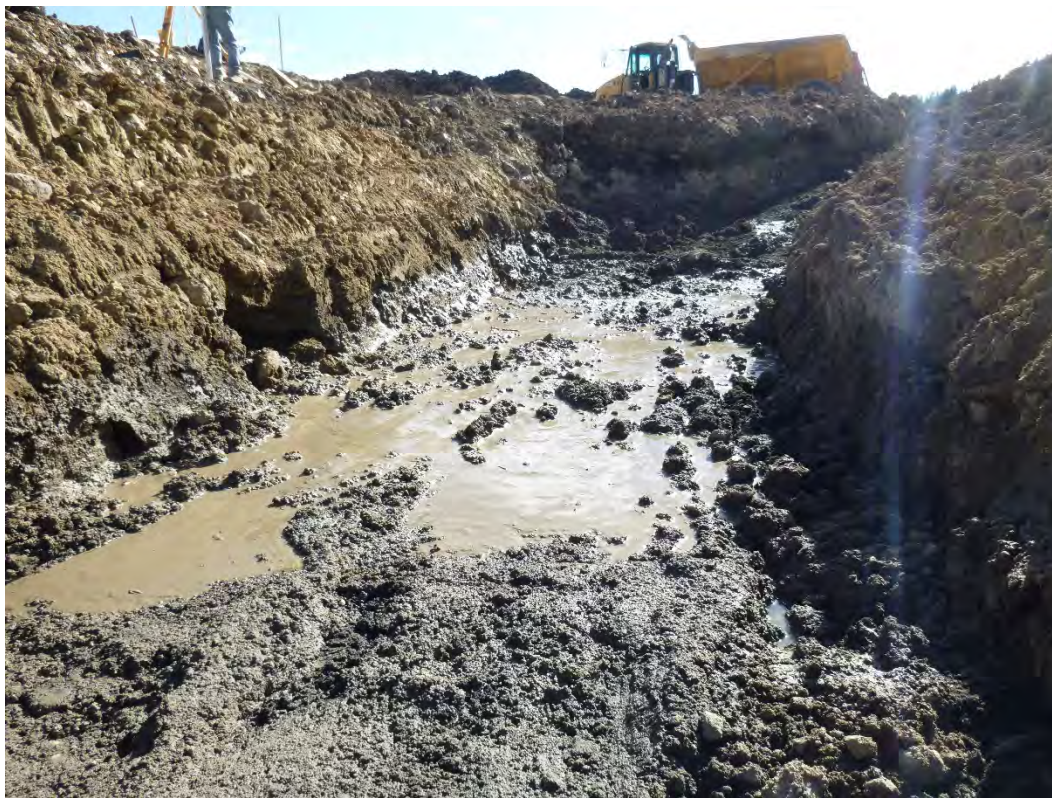
Upstream end of outlet works foundation; estimated Sta. 0+40.
