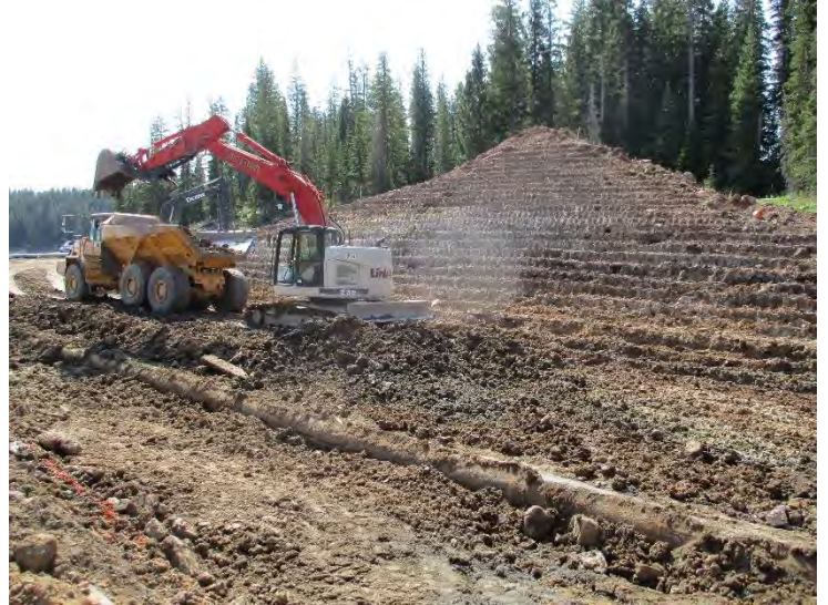
Photo 8. View of the old, exposed pipe, prior to removal
