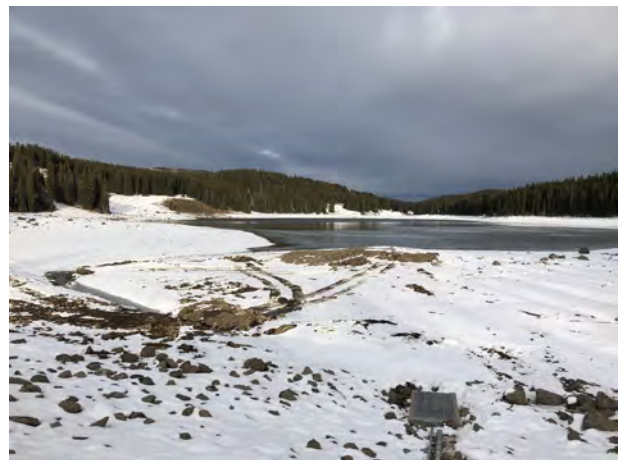
Photo 4. View looking north at Deep Ward Lake. Note inlet structure at bottom of photo. Photo taken on 11/20/2020.
