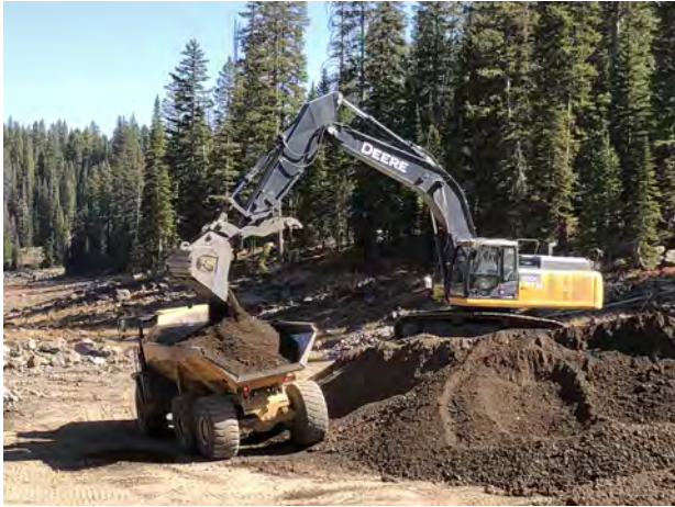
Photo 1. View of loading operation of screened embankment material for placement of on the next embankment lift.
