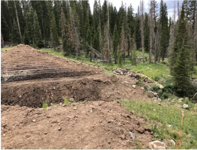
Photo 1. View looking east at existing breach excavation progress on July 22, 2020.
