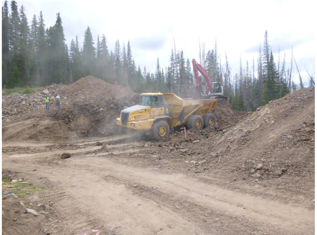
Expansion of existing breach per Excavation Plan.
