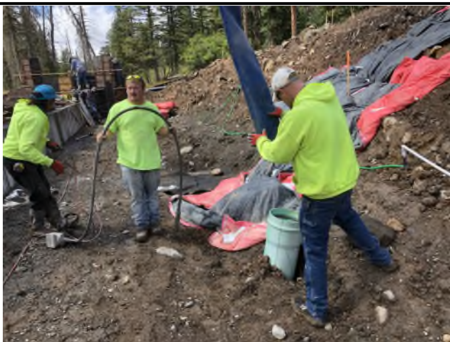
Photo 3. ConSy crew grouting in the dewatering wells with concrete.
