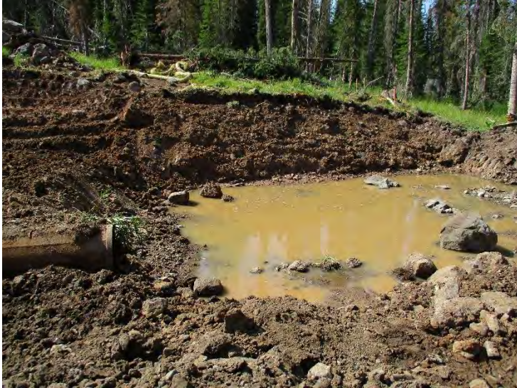
Photo 7. Stilling basin - terminal end of pipe (area to be dewatered)
