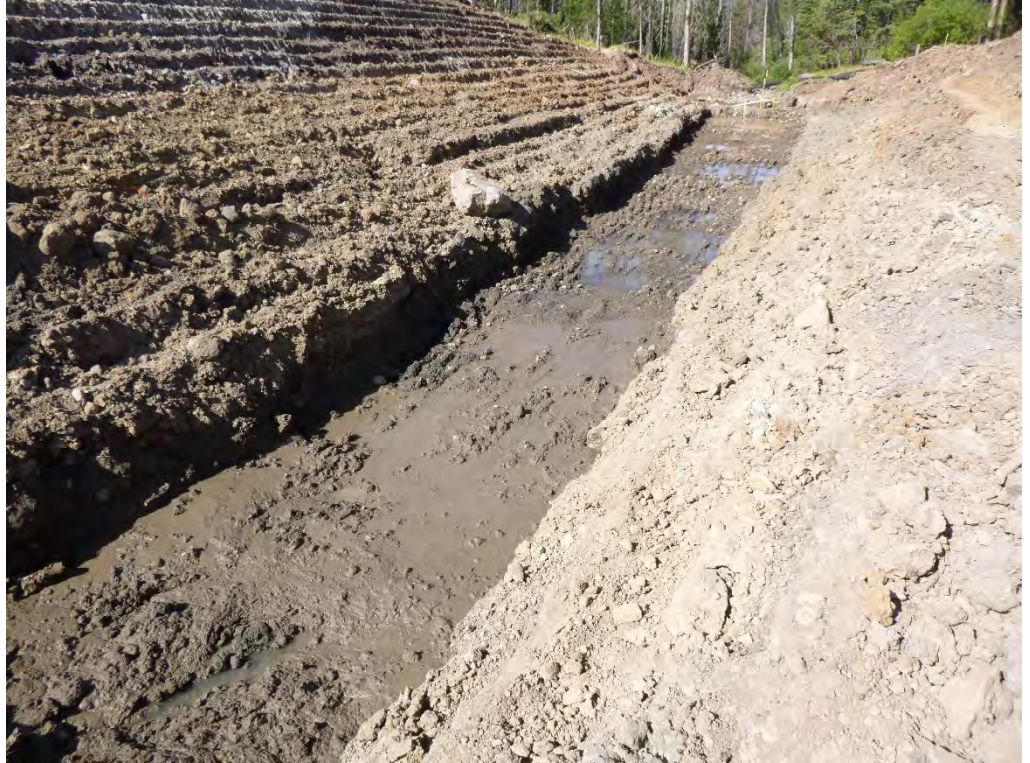
Overall view of outlet works foundation looking in downstream direction.
