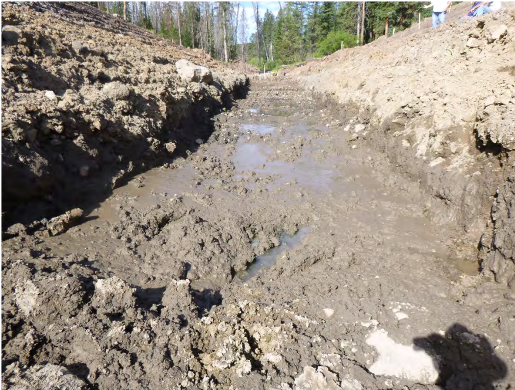
View looking downstream along outlet works foundation.
