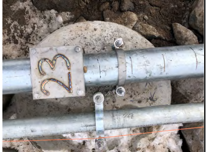
Photo 2. Detail of typical gate stem support pier at the 23-foot level marker.
