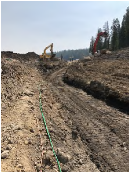
Photo 3. View looking north at subgrade prior to proof-roll test.
