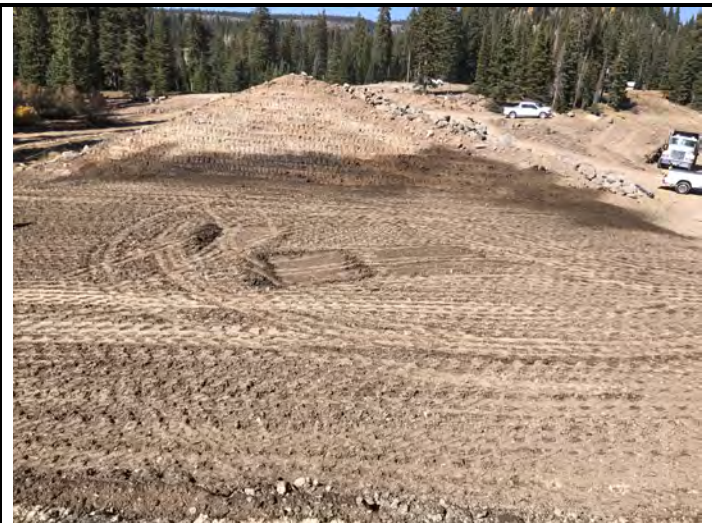
Photo 4. View looking west across breach at typical test location for nuclear moisture-density testing.
