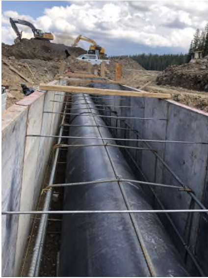
Photo 1. View looking north at HDPE outlet pipe encasement formwork and reinforcing steel.
