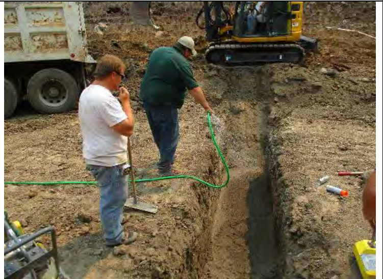
Photo 4. Moisture conditioning the filter material. Con-Sy may opt to apply water while material is in the truck.
