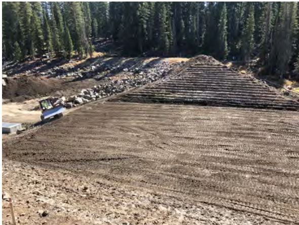
Photo 1. View looking east completed embankment lifts. Note previously moistened benches to the left of the water truck
