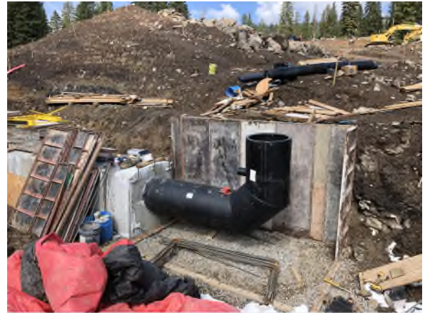
Photo 2. Closeup of fused HDPE inlet pipe prior to forming inlet structure.
