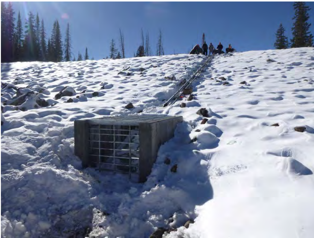
Outlet gate intake structure and trashrack.
