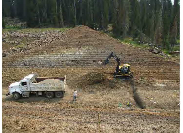
Photo 2. Dump truck backing up to test area (actual trench location) with excavator waiting.
