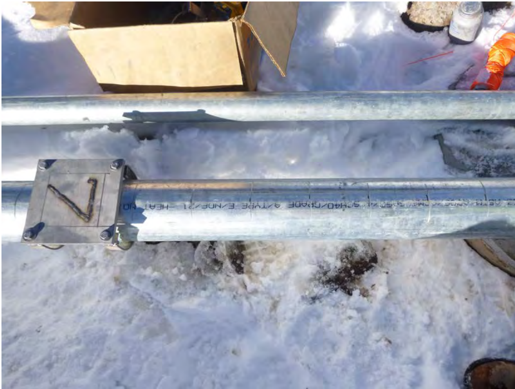
Close-up of typical 1-foot interval number plates and air vent scribes for staff gage tenths of feet.
