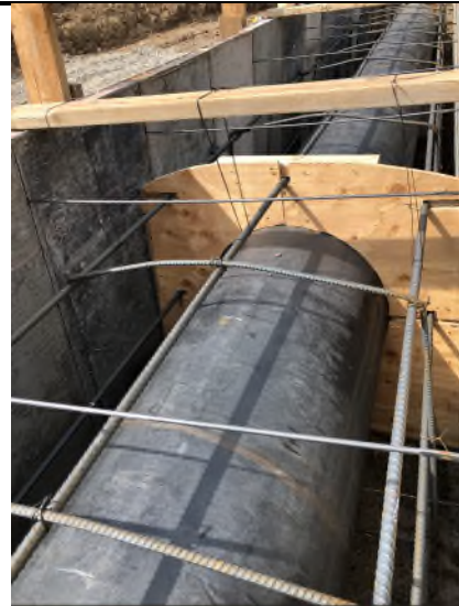
Photo 4. View of typical plywood bulkhead between 20-foot segments of encasement. 2"x4" wood crossbeam at top of photo is typical of 6-foot spacing for wire ties to provide required 5-inch spacing of rebar above the pipe during concrete placement
