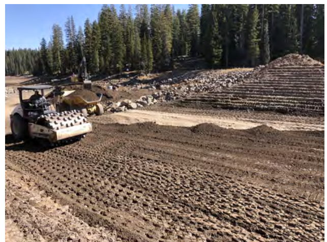
Photo 4. View of compaction of material spread in 8-9 inch lifts. Dump truck is in the background preparing to deliver more screened embankment material
