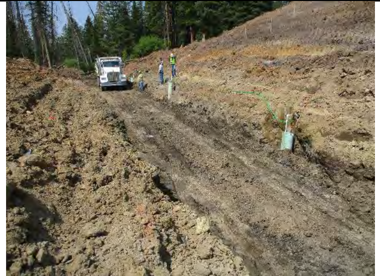
Photo 2. End of third pass. Soft spots were identified in the vicinity of the center and downstream wells.
