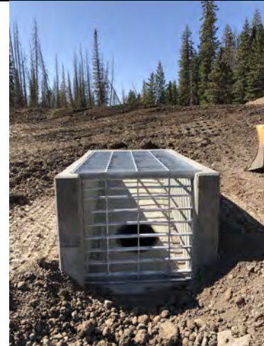
Photo 2. View looking south (downstream) at inlet structure with trash rack installed. Fresno gate was delivered to site that date.
