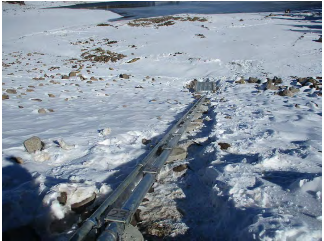
View looking down upstream slope along gate stem and air vent alignment.
