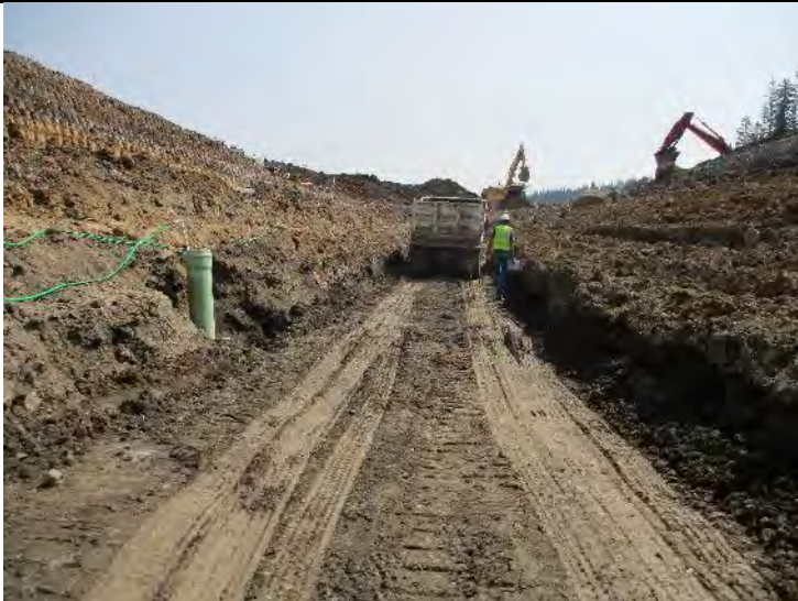
Photo 1. First proof roll, end of second pass.
