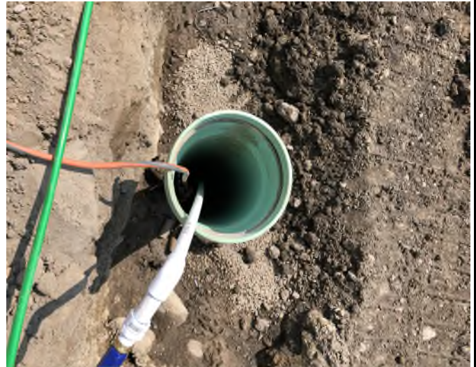
Photo 2. Close-up one of three dewatering wells installed by ConSy. PVC and PureCore pipe connects to the outlet bypass pipe..
