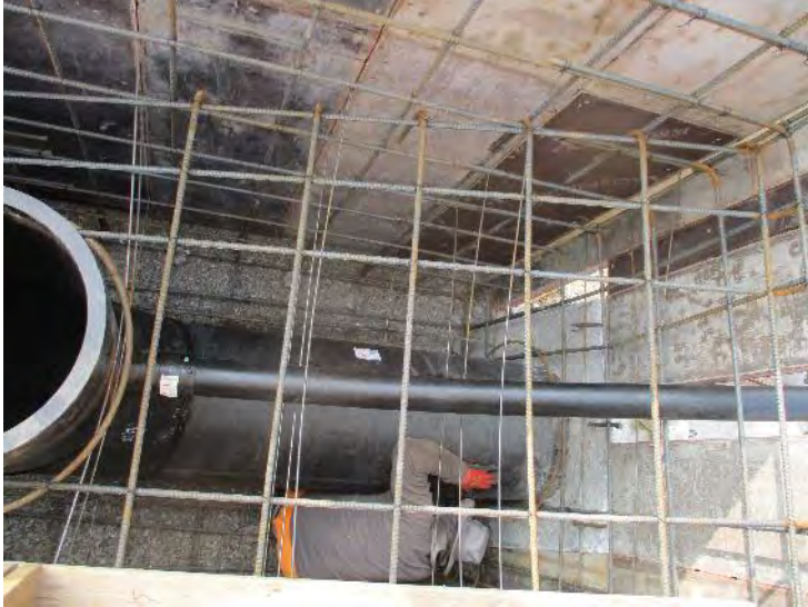
Photo 5. Overhead view of intake structure steel.
