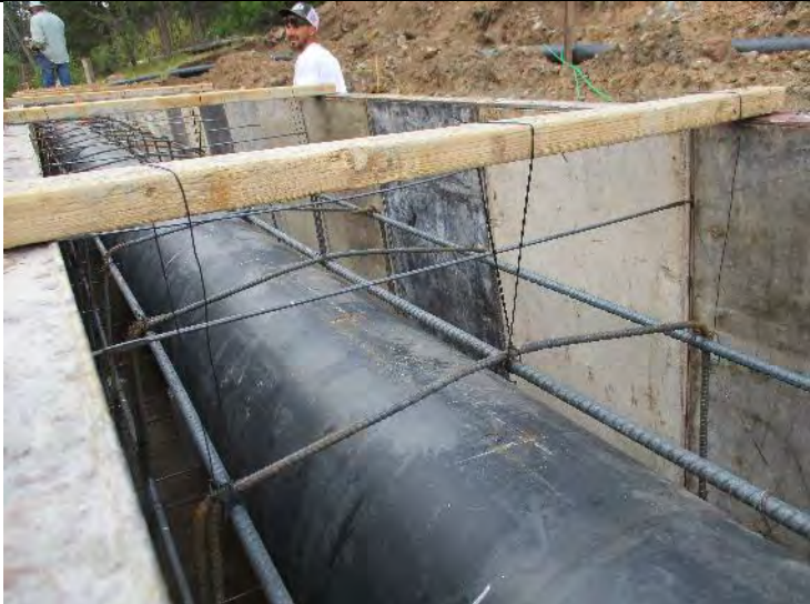
Photo 3. Ties every 6-feet to suspend the structural steel cage a minimum of 3-inches above the ground. Sidewall chairs to be placed to ensure 3-inch clearance from wall forms.
