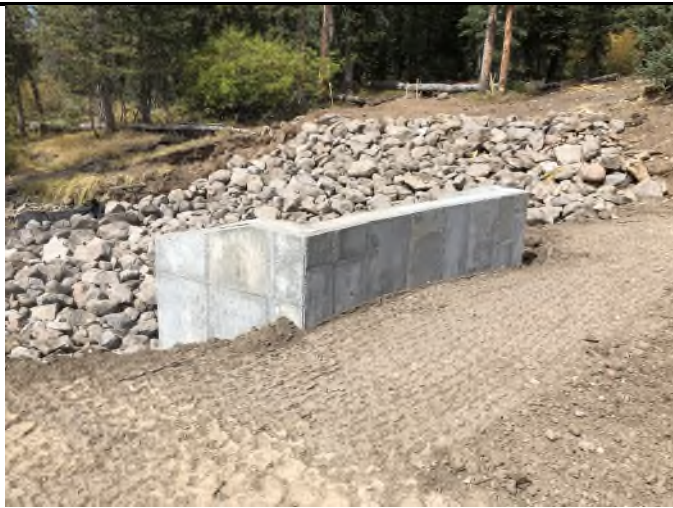
Photo 3. Close-up of the outlet structure and stilling basin rip-rap
