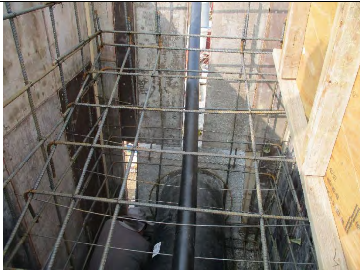
Photo 3. Looking toward the back wall of the intake structure from the reservoir side.
