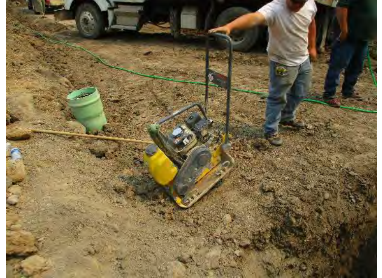
Photo 6. The Wacker Packer. Following one half of the pass, a strap was affixed to the compactor, which was raised by the excavator and turned around to complete the second half of the pass. The Wacker Packer was slightly wider than the trench.
