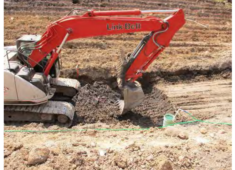
Photo 4. Two spots identified as yielding during proof roll were overexcavated by two additional feet, then backfilled with embankment materials and compacted.
