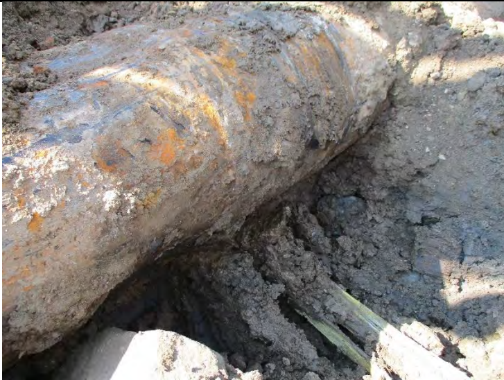
Photo 1. Exposed area beneath old pipe - note woody debris from forms left in place during concrete collar construction
