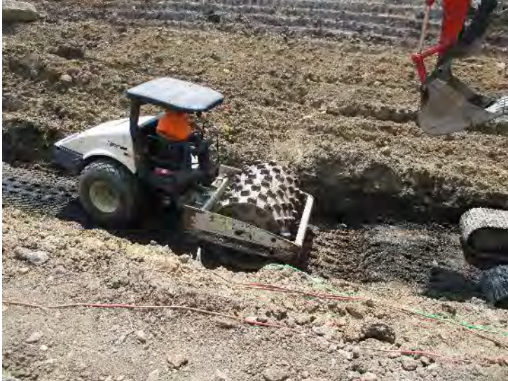
Photo 7. Backfilling: three lifts of embankment materials, each compacted by five passes with a sheepfoot roller.
