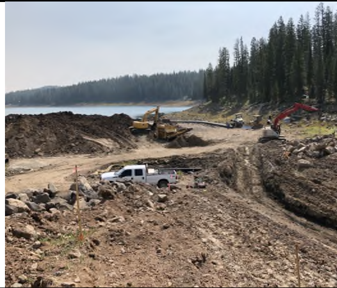
Photo 1. View looking north at outlet channel prior to subgrade proof-roll test on August 14, 2020.
