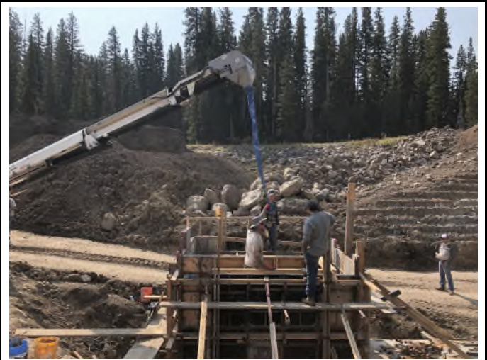
Photo 2. Concrete placement at inlet structure using conveyor belt and tremie.
