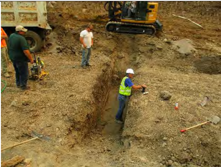
Photo 7. Grab sample collection following completion of test section, to evaluate for over-compaction and increased fines.
