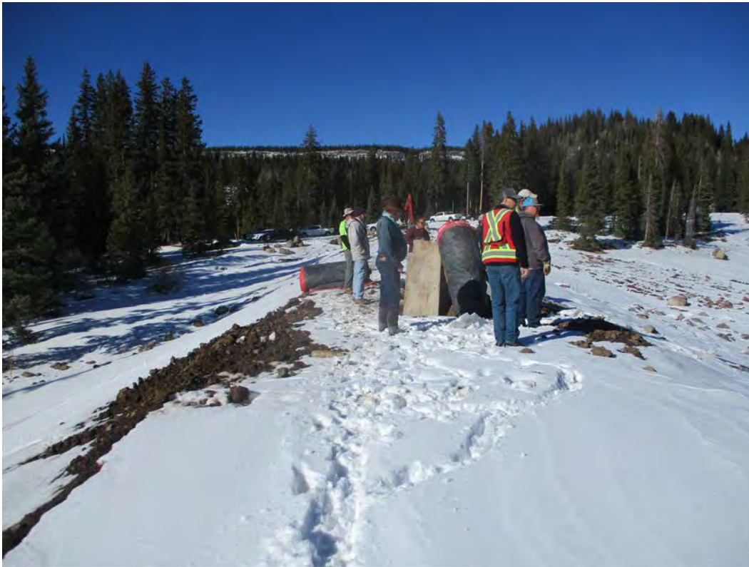
Dam crest area just left gate operator support structure in need of minor grading to fill in low spot and correct drainage.
