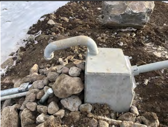
Photo 3. Close-up view of outlet gate control wheel block. Photo taken on 11/20/2020.
