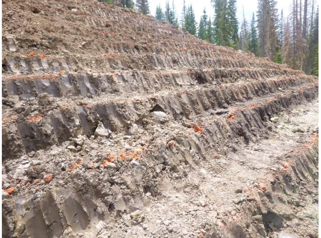
Close-up of benched sideslope.
