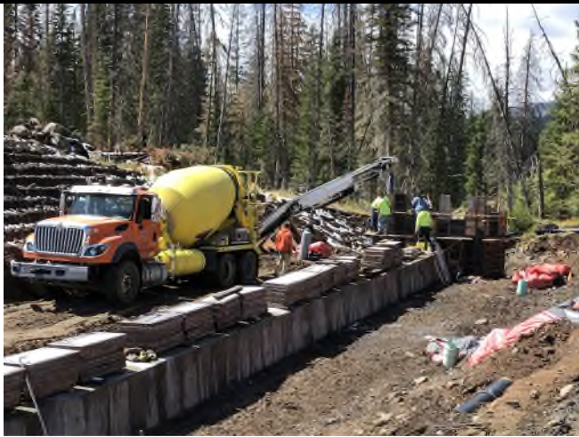
Photo 1. View looking south at concrete placement for the outlet structure.
