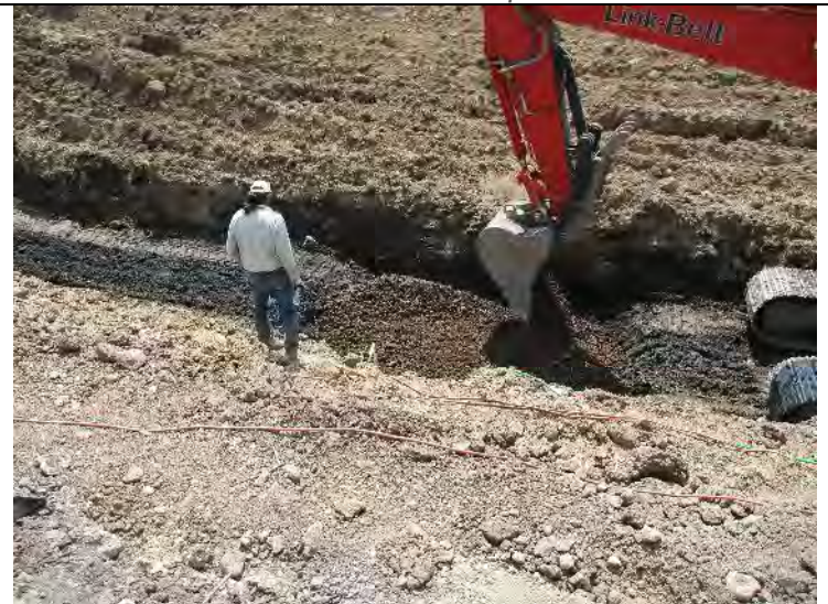
Photo 6. The excavator spreads embankment material into the 2-foot overexcavated areas.
