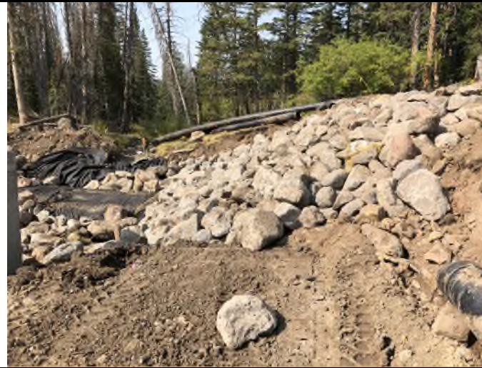
Photo 1. Rip-Rap placement at outlet spillway taking place concurrently with the inlet structure concrete placement on 9/18/20
