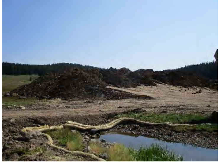
Photo 12. Newly excavated stockpiled material - Con-Sy plans to transport a shaker/screener to the site to facilitate removal of large D-50 elements
