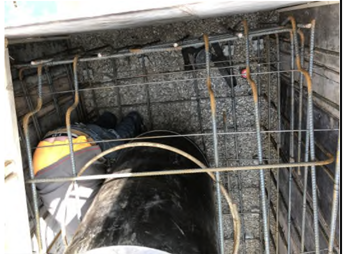
Photo 2. Closeup of inlet reinforcing steel placement.
