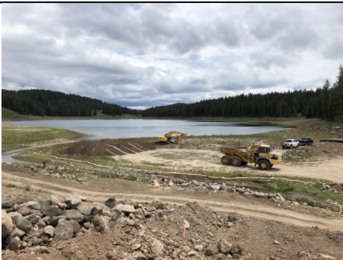
Photo 3. View of Ward Lake reservoir and material stockpiling progress.
