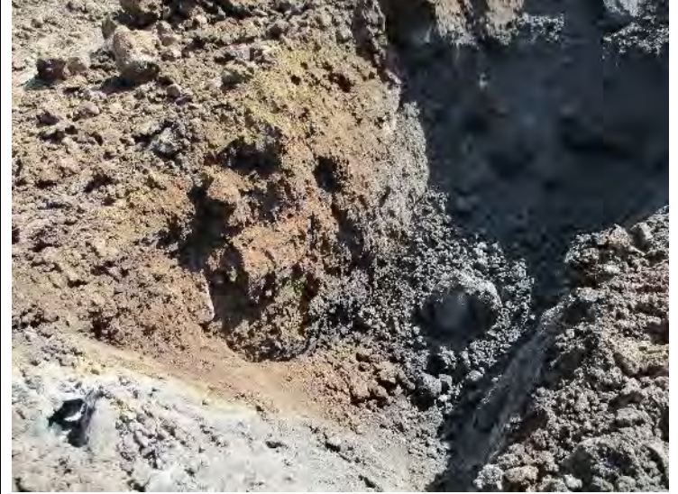
Photo 16. View into excavation directly adjacent to outlet - generally clayey material
