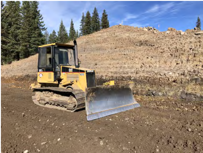
Photo 3. Close-up Cat D5 dozer used to mix and spread embankment material. Note curved blade.
