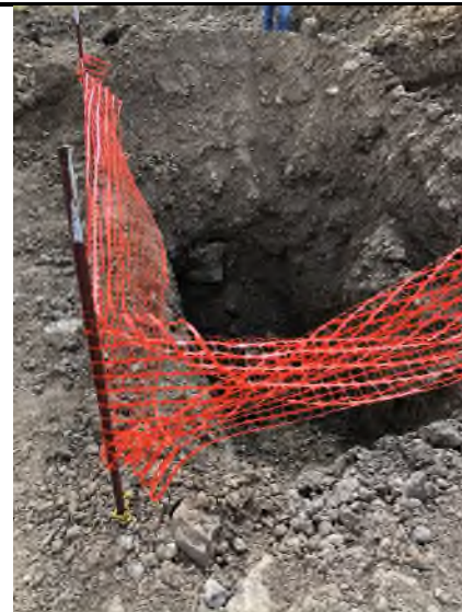
Photo 4. View of test pit excavated on the east side of the existing steel outlet pipe to observe site soils.
