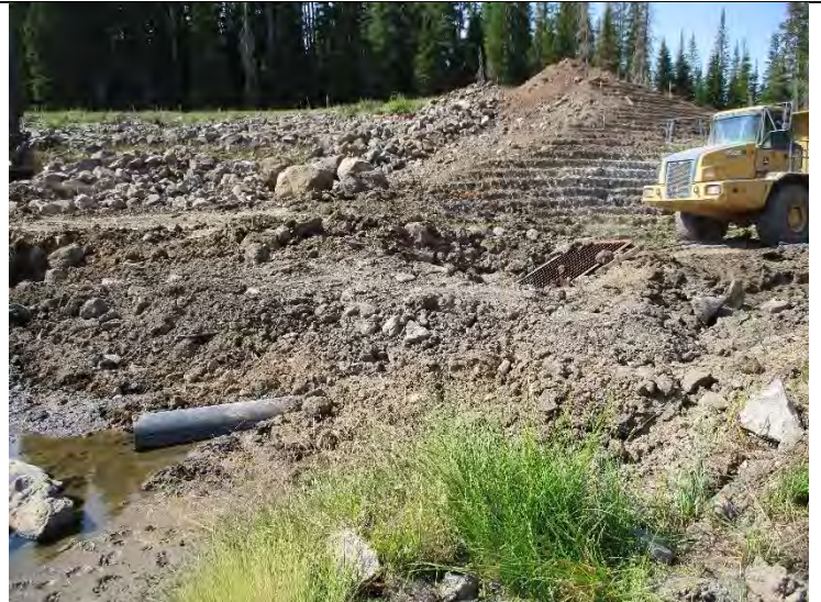
Photo 10. Bypass pipe inlet - old trash rack is visible in center right of photo
