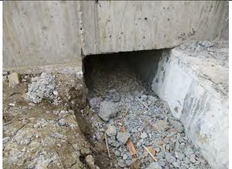
Photo 8. Rectangular void for filter sand, just upstream of outlet headwall (reference detail B on sheet 14).
