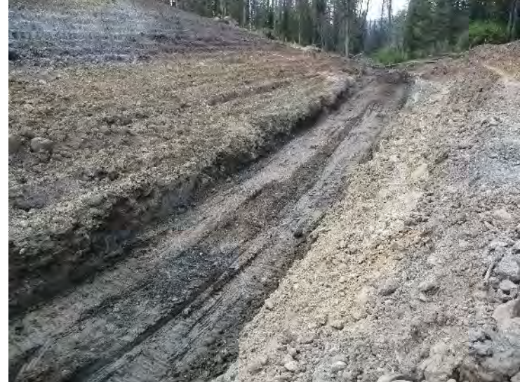
Photo 8. Second proof roll. Looking downstream.
