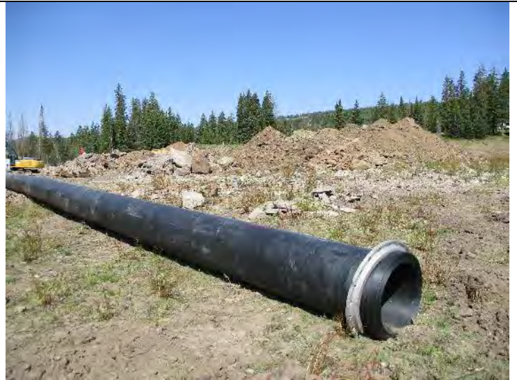
Photo 14. The new pipe
