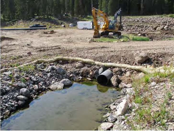
Photo 11. Access over bypass - photo is taken upstream from Photo 10
