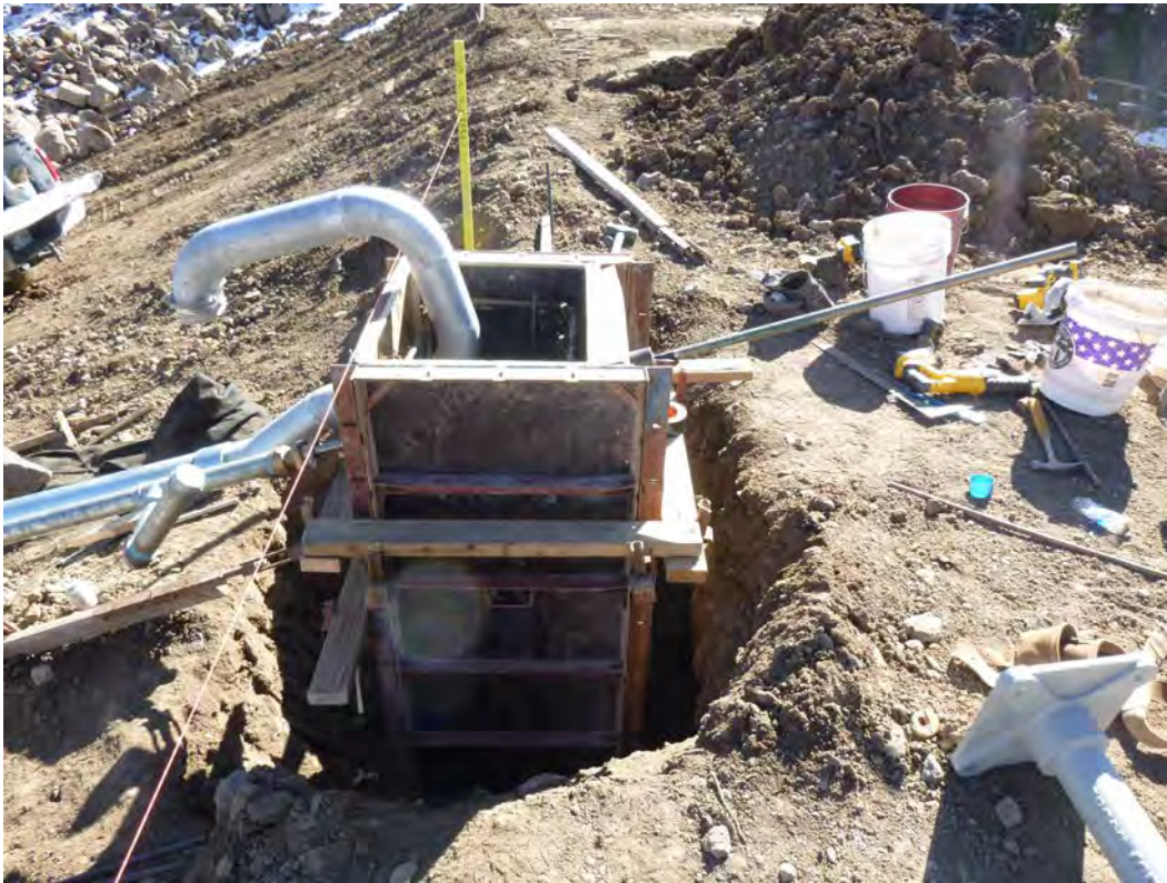
Gate Control Hand Wheel Support Structure concrete reinforcement and formwork.
