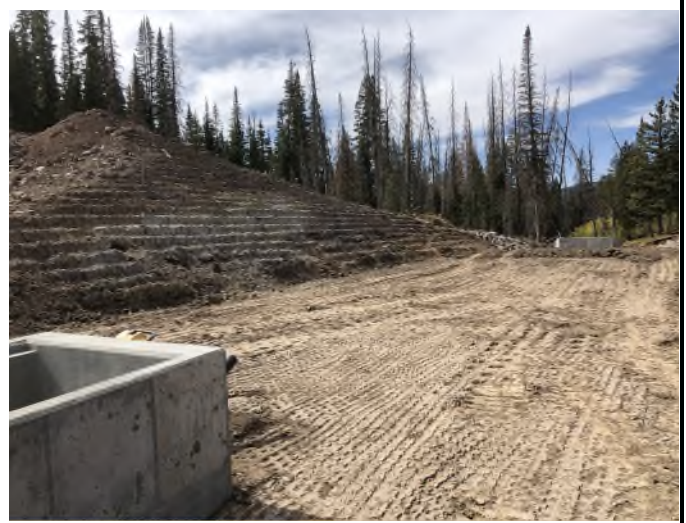
Photo 2. View looking south (Downstream) at embankment fill above the outlet pipe encasement. Note inlet structure on the lower left of the photo.
