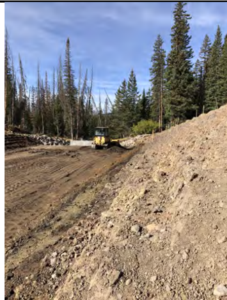
Photo 4. View looking south (downstream) at D5 Cat dozer spreading embankment soil on the first benched lift.
