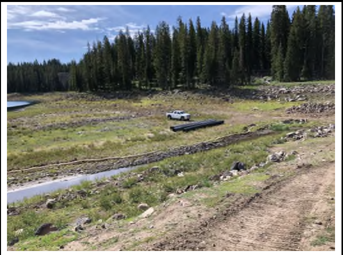
Photo 2. View looking northeast at erosion control measures of inlet channel and HDPE pipe for the outlet.
