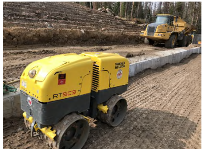
Photo 4. View of remotely operated compactor used to compact the first 3-feet of embankment adjacent to the outlet pipe encasement section.
