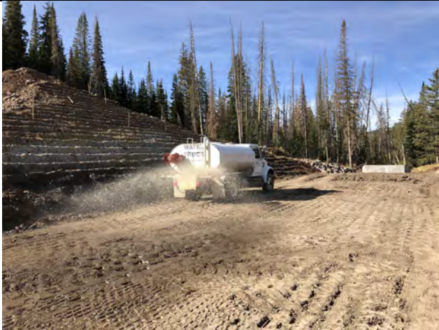
Photo 1. View looking south (downstream) at water truck wetting subgrade prior to embankment material placement. Note previously moistened benches to the left of the water truck
