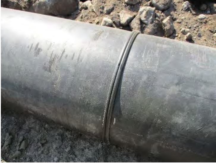
Photo 15. Close-up view of pipe weld
