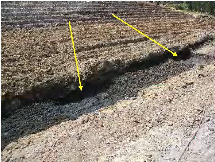
Photo 5. Two overexcavated spots.
