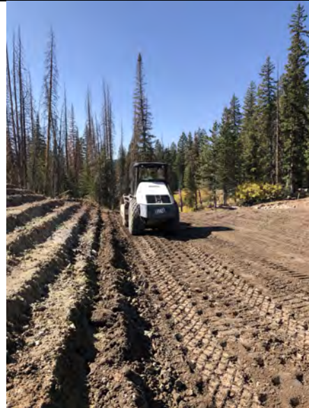
Photo 2. View looking south (downstream) at single drum sheepsfoot compactor during lift compaction on the east side of the breach.
