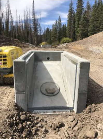
Photo 1. Close-up of inlet structure looking downstream.
