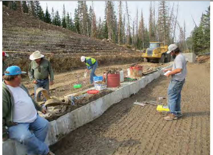
Photo 10. DOWL and Con-Sy collect nuclear gauge readings of the embankment material.
