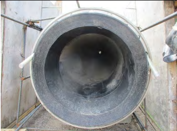
Photo 1. Looking downstream into the HDPE pipe, a slight bend to the right is noted. Temperatures range from mid-to-low 40s in the evening to upper 60s during the day.
