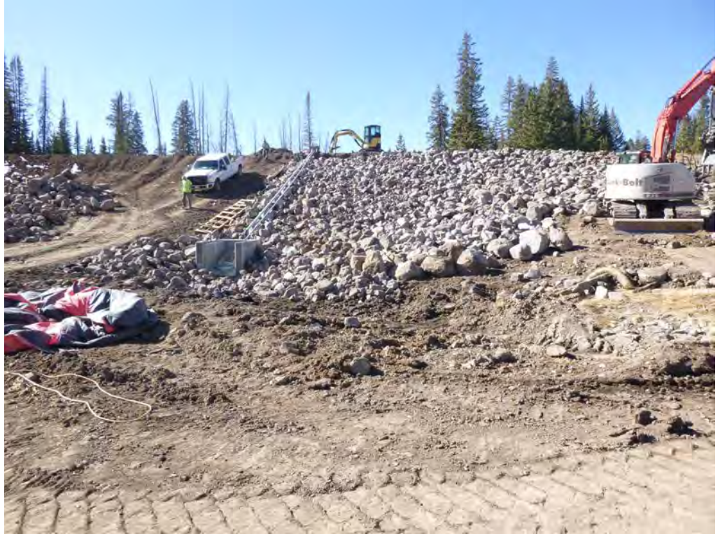
Overall view of breach repair section and upstream outlet works.
