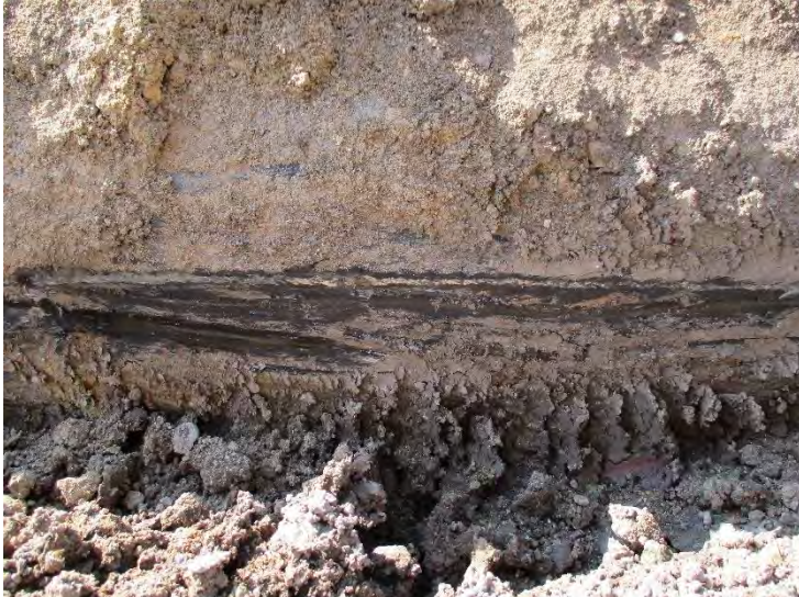
Photo 3. Pipe is described as 1/4-inch thick, asbestos wrapped welded steel pipe with arc weld joints (reference C-0590 specifications) - photo shows outer material scraped away, revealing steel beneath
