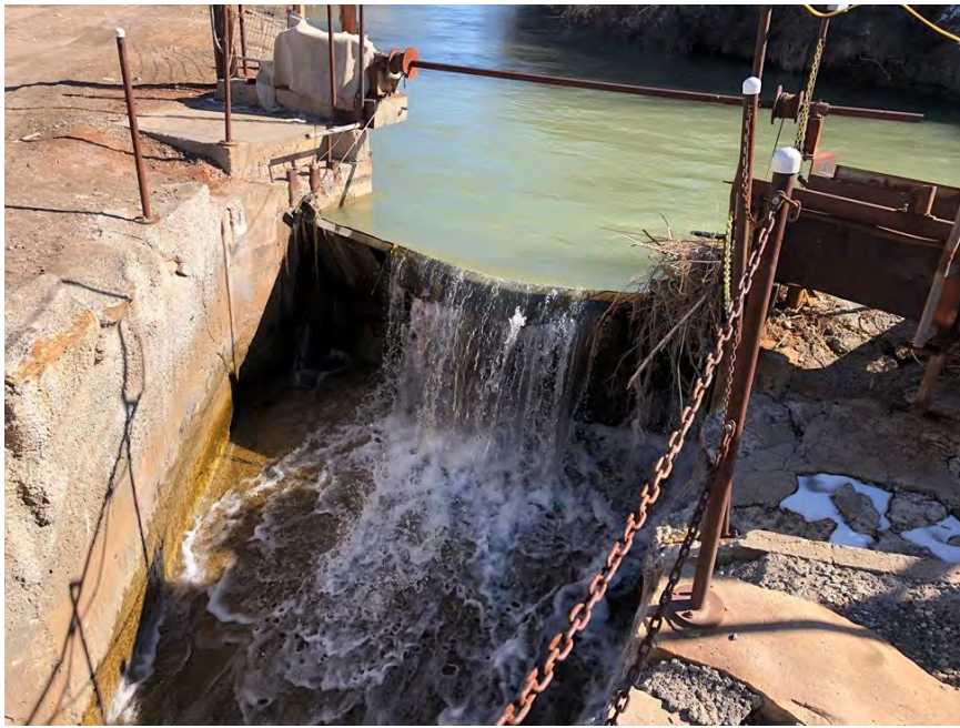
Figure 2.4.1. Current Condition of Overshot Gate on Bypass Chute
