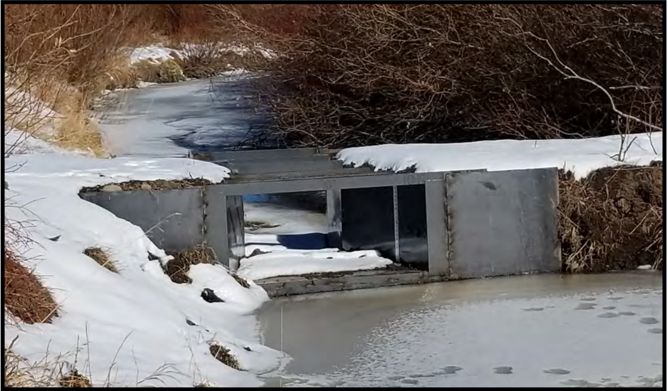
Photos of Parshall flume showing 30" throat x 24' deep channel. Sheet steel is 1/8" galvanized. Wing wall and cut-off projections have been increased for durability.
