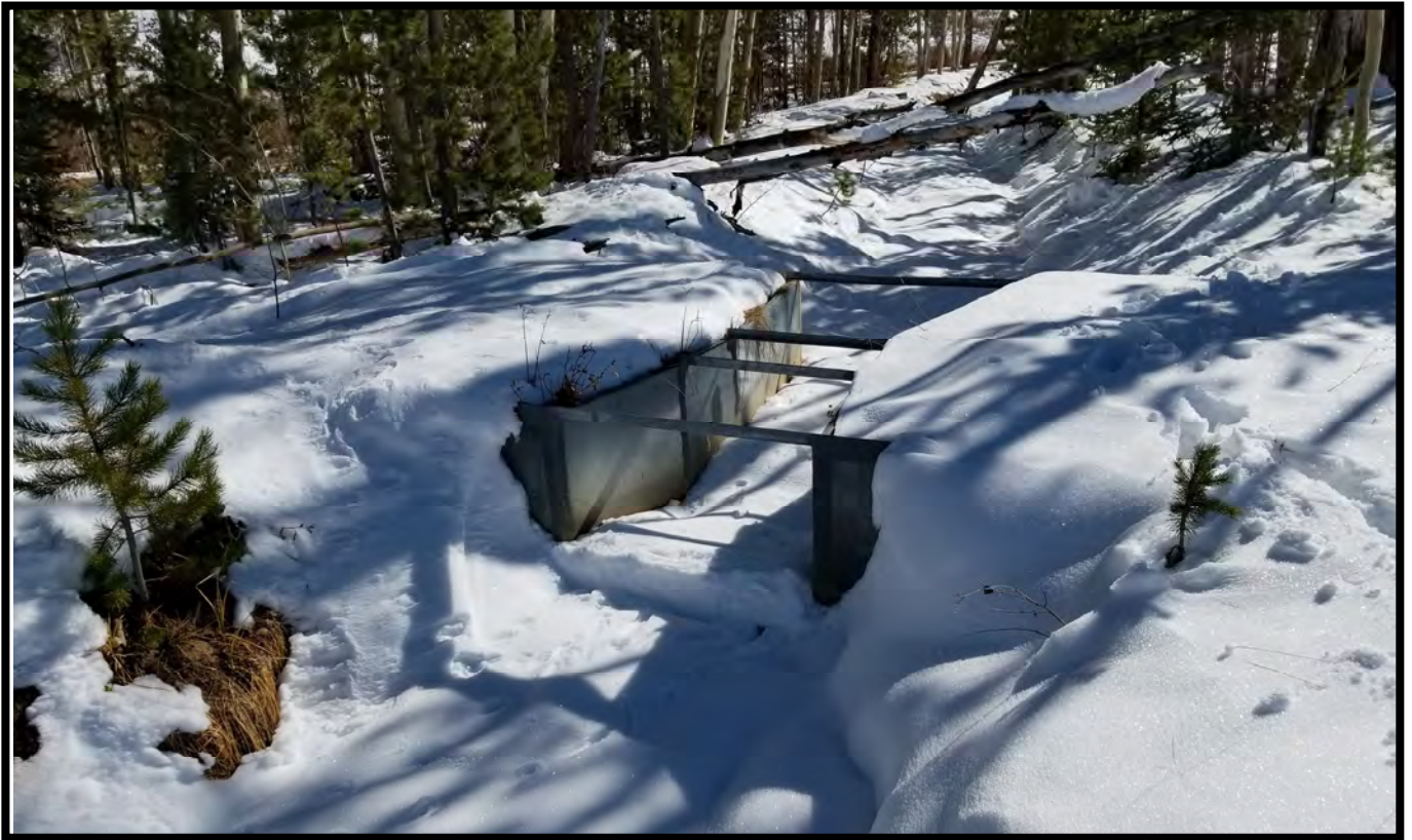
Photos of Parshall flume showing 36" throat x 2' deep channel. Sheet steel is 1/8" galvanized. Wing wall projection increased using pressure treated plywood.
