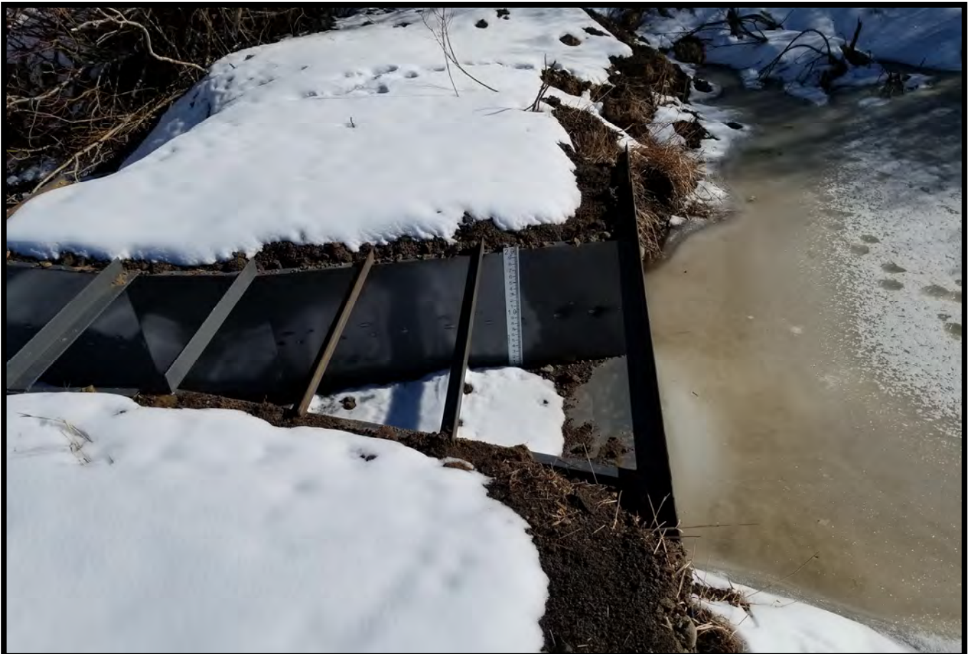
Photos of Parshall flume showing 30" throat x 24' deep channel. Sheet steel is 1/8" galvanized. Wing wall and cut-off projections have been increased for durability.
