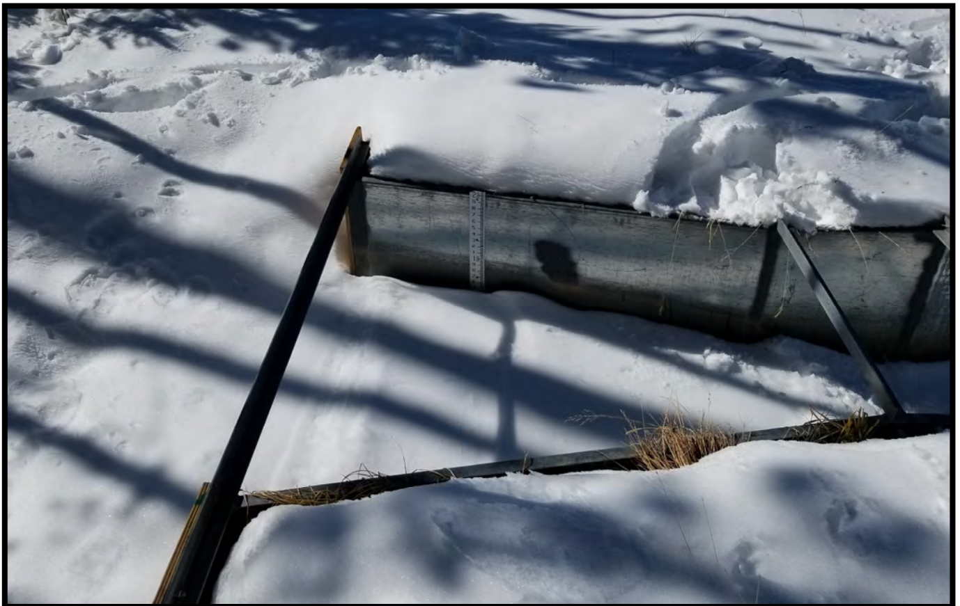
Photos of Parshall flume showing 36" throat x 2' deep channel. Sheet steel is 1/8" galvanized. Wing wall projection increased using pressure treated plywood.
