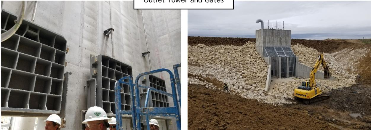
Construction of Mud Mat and Outlet Terminal Structure
