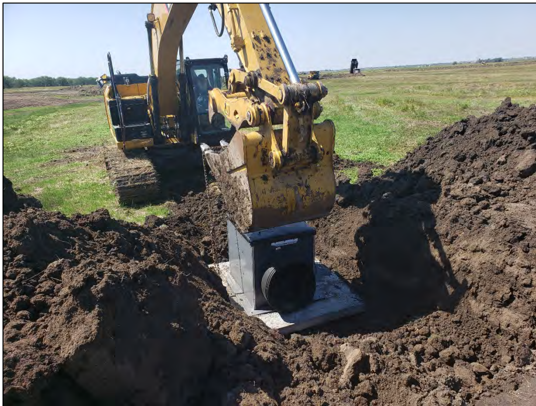
Figure 4. Installing outlet pipe on structure. Note anti-seep collar.
