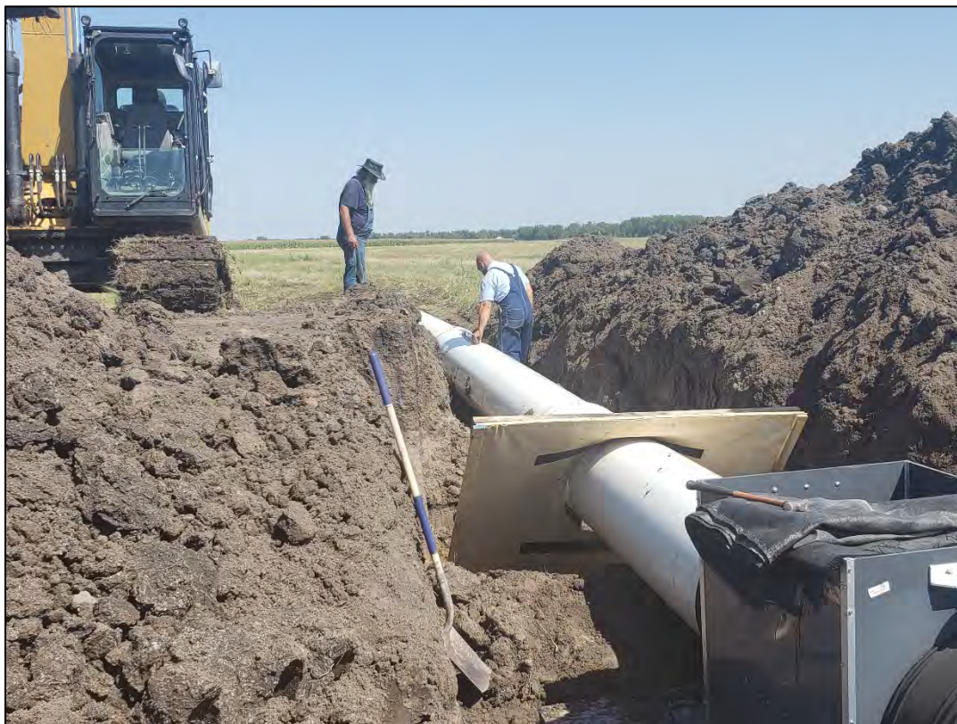
Figure 4. Installing outlet pipe on structure. Note anti-seep collar.
