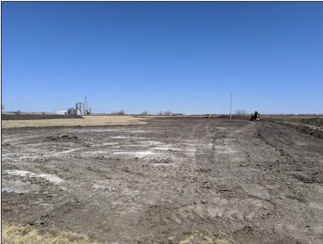
Figure 6. Earth-moving to build embankments on east wetland levees.
