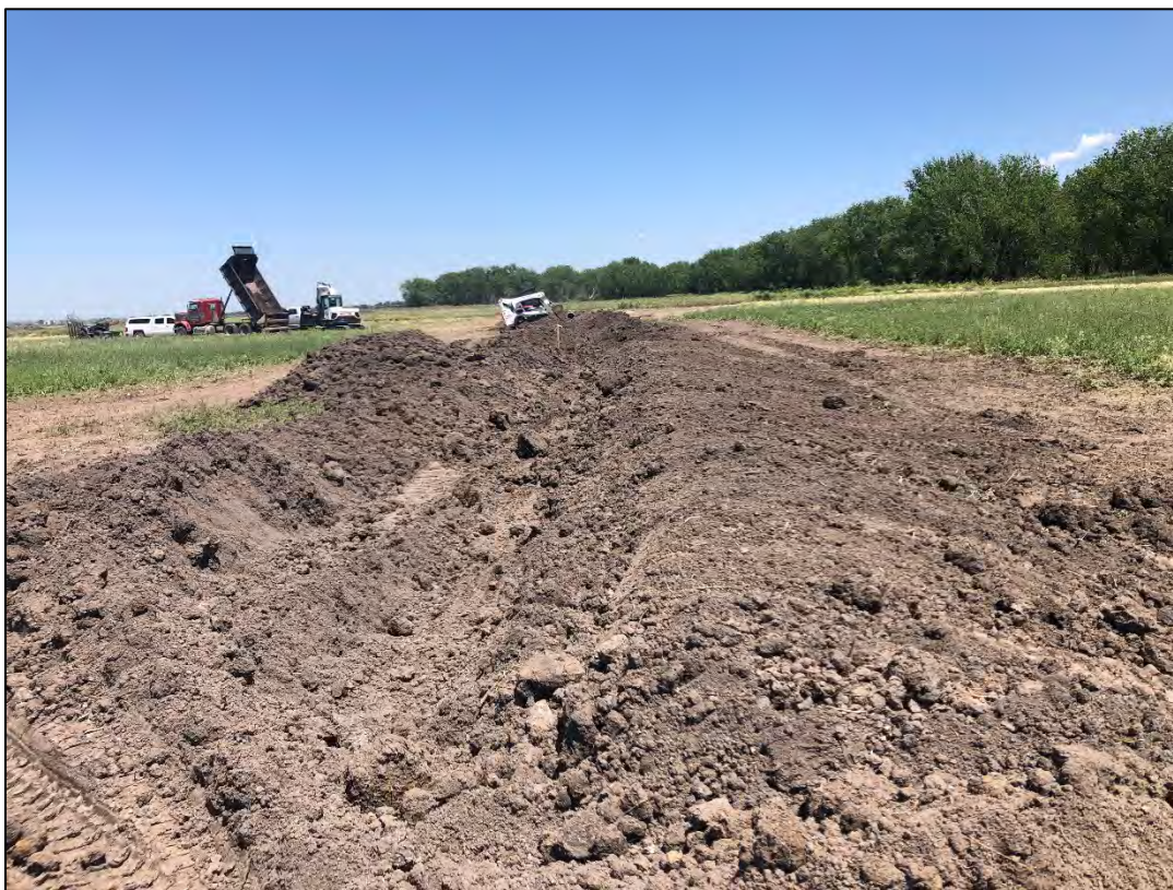
Figure 2. Finishing the west wetland embankment.
