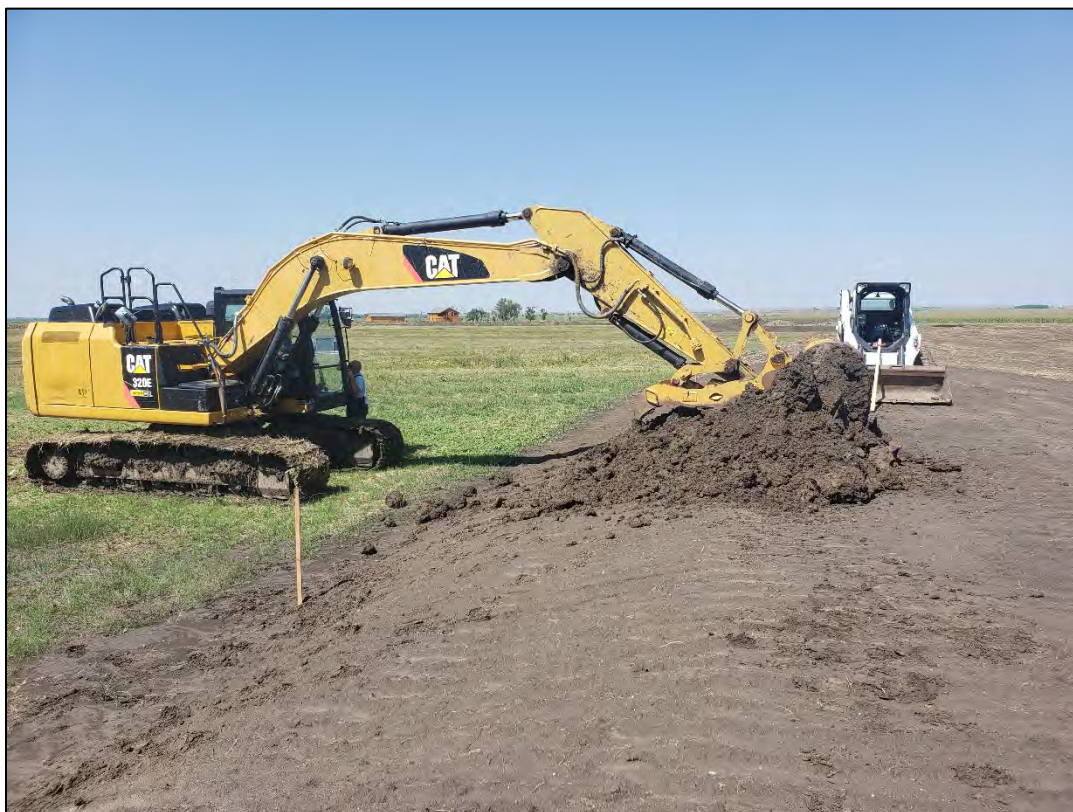
Figure 2. Finishing the west wetland embankment.
