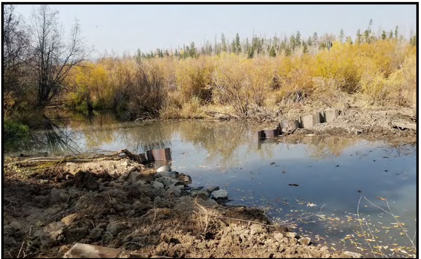
Photos of Headgate pipe. Pipe is 18" x 20' ADS N12 pipe. Gates are Waterman C10 or equal, flat back 18" cast iron slide gates with 5' frames. Compaction is present and installation is good. Sheet Piling is PZ22. Rock is sound, durable and angular in shape and meets required dimensions.
