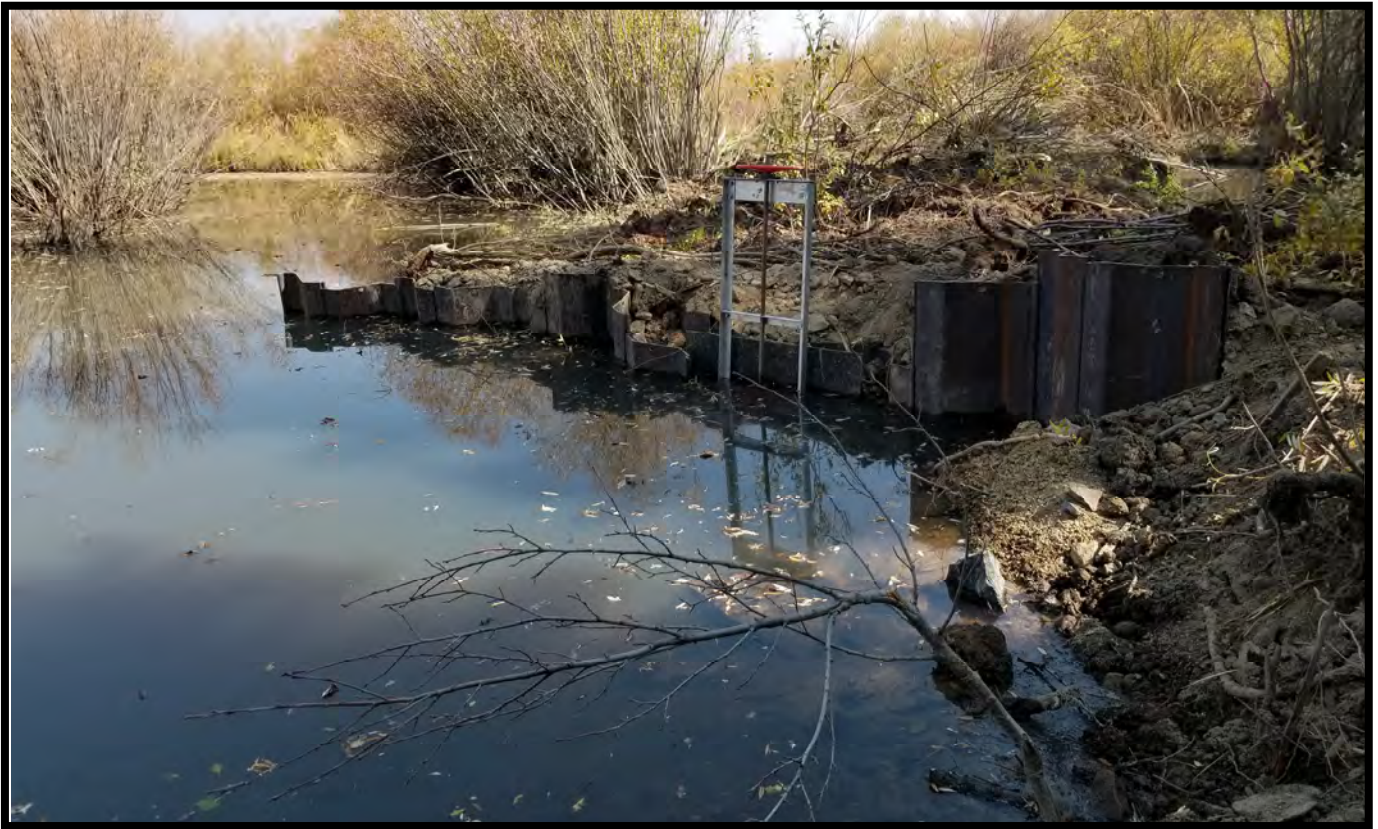
Photos of Headgate pipe. Pipe is 18" x 20' ADS N12 pipe. Gates are Waterman C10 or equal, flat back 18" cast iron slide gates with 5' frames. Compaction is present and installation is good. Sheet Piling is PZ22. Rock is sound, durable and angular in shape and meets required dimensions.
