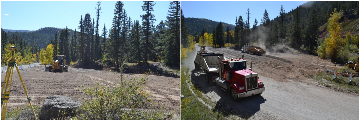
Figure 7. OHV unloading and parking area site grading and construction
