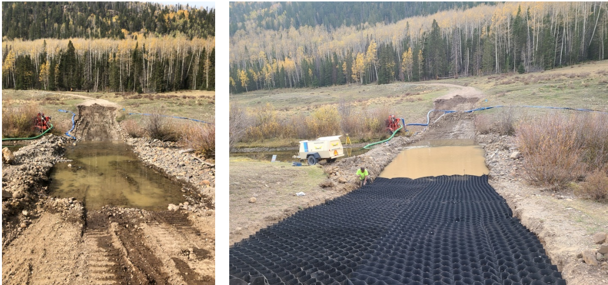
Figure 6. FS Road 390 Stream Crossing Construction
