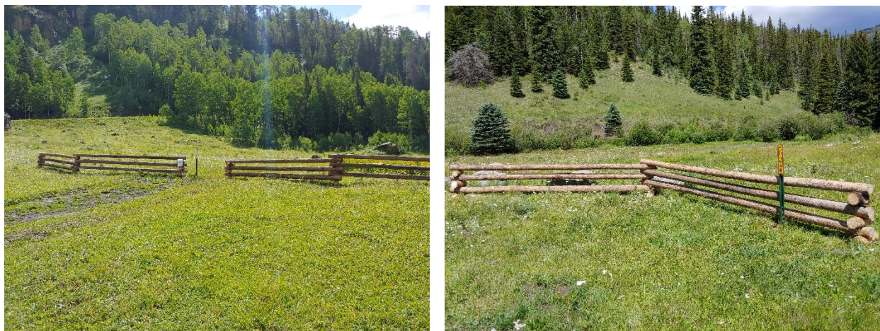
Figure 8. Worm Fencing and U-channel signs
