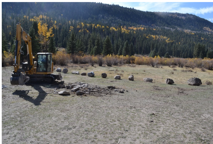
Figure 12. Boulder placement
