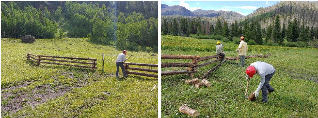
Figure 4. Worm Fencing and U-Channel Installation
