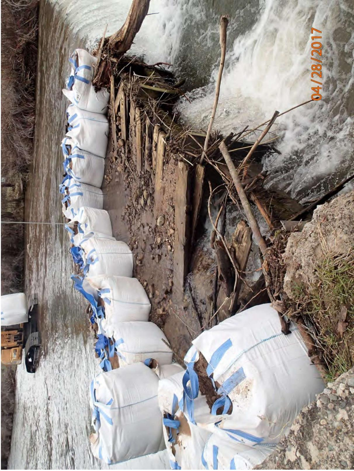
Photo 3: Florida Canal Diversion Structure - Emergency Repair 2
