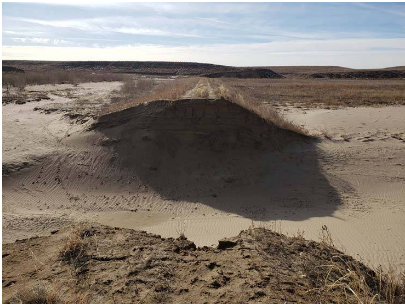
Photo 2: Dam #4 at Breach
