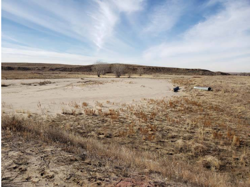
Photo 3: Dam #4 below breach showing displaced outlet pipe downstream
