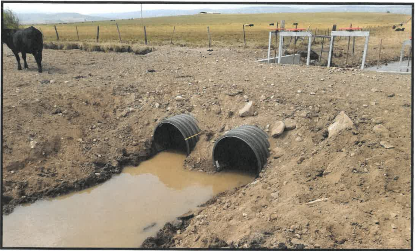
Above: Photo of the outlet end of the pipes (HDPE 36" x 20') in the main ditch—staples ditch.
