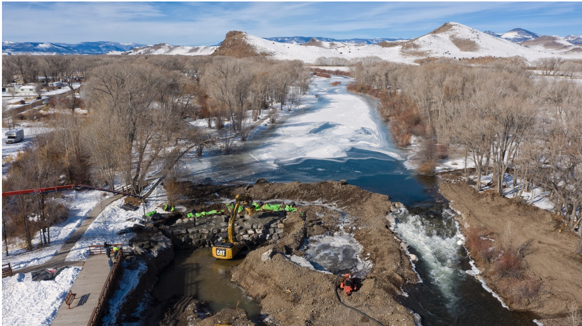
Figure 5. Construction of Grouted Rock Playwave.
