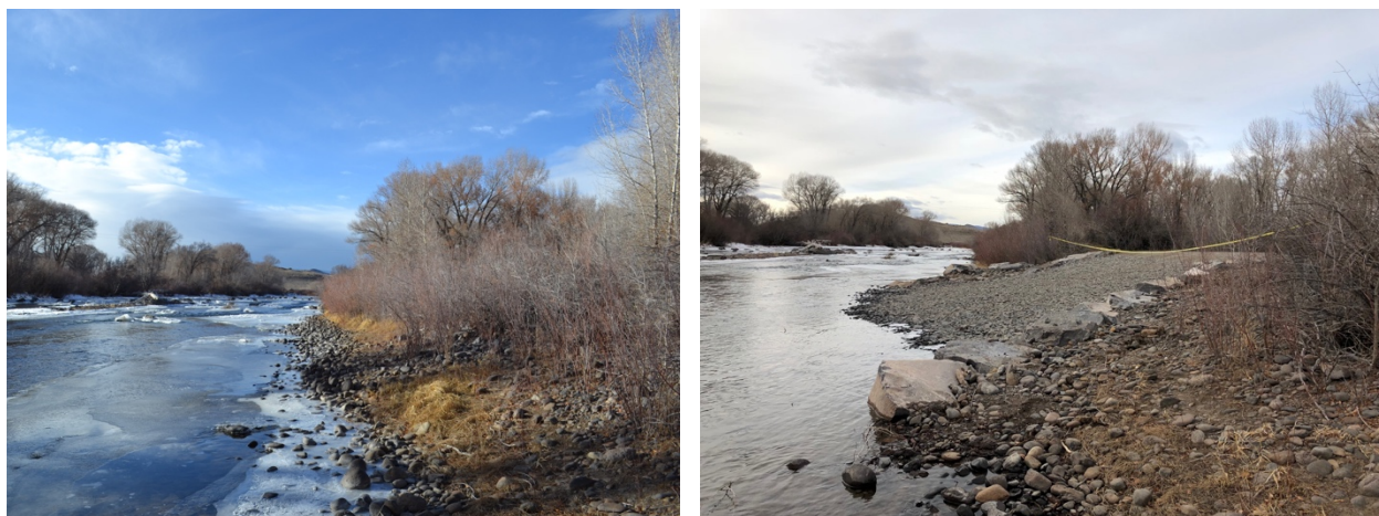
Figure 8. DNRP Boat Ramp Site Before (left) and After (right) Construction.
