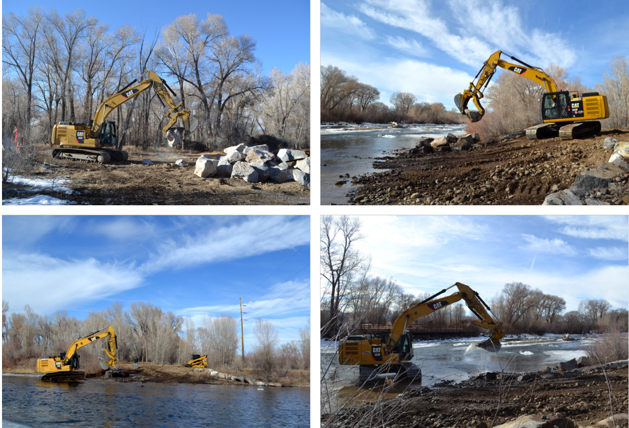
Figure 4. Construction of DNR Boat Ramp.
