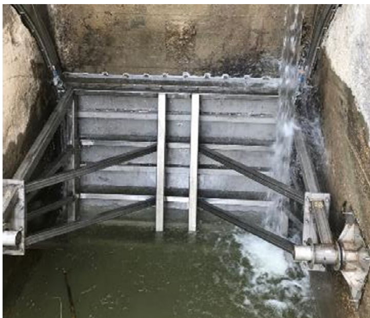
Figure 6. New Stainless Steel Bypass Gates.
