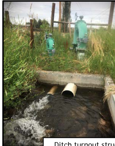
Ditch turnout structures for shareholders
