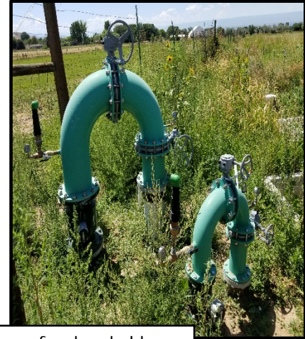
Ditch turnout structures for shareholders
