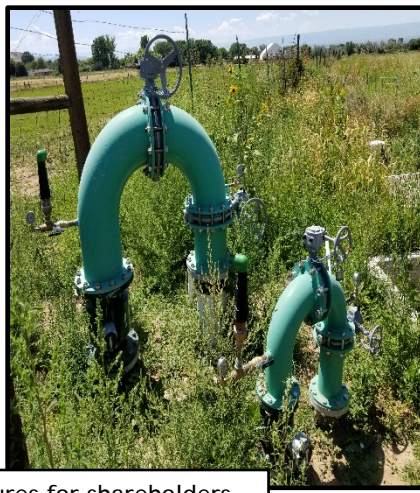
Ditch turnout structures for shareholders
