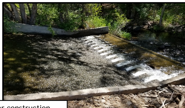
Inlet structure after construction
