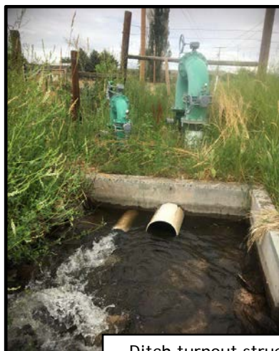
Ditch turnout structures for shareholders
