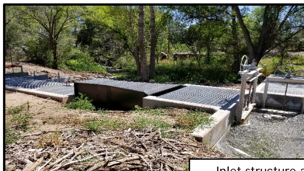
Inlet structure after construction
