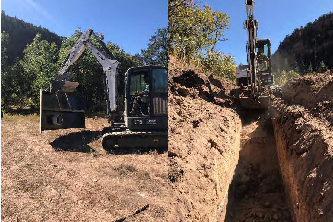
Figure 1 Hood Exc. excavating trench for pipe
