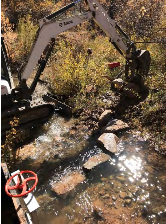
Figure 4 Hood Exc. Installing diversion weir
