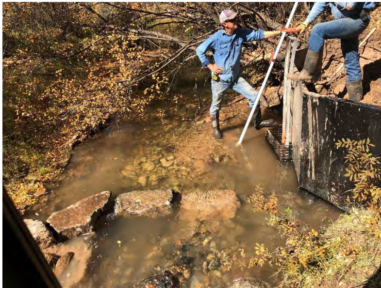
Figure 3 TU and ER staff installing new headgate
