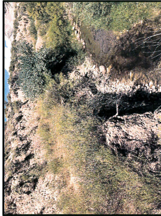
Parachute Creek undercutting nearing Diamond Ditch embankment. Ditch to be re-aligned away from creek.
