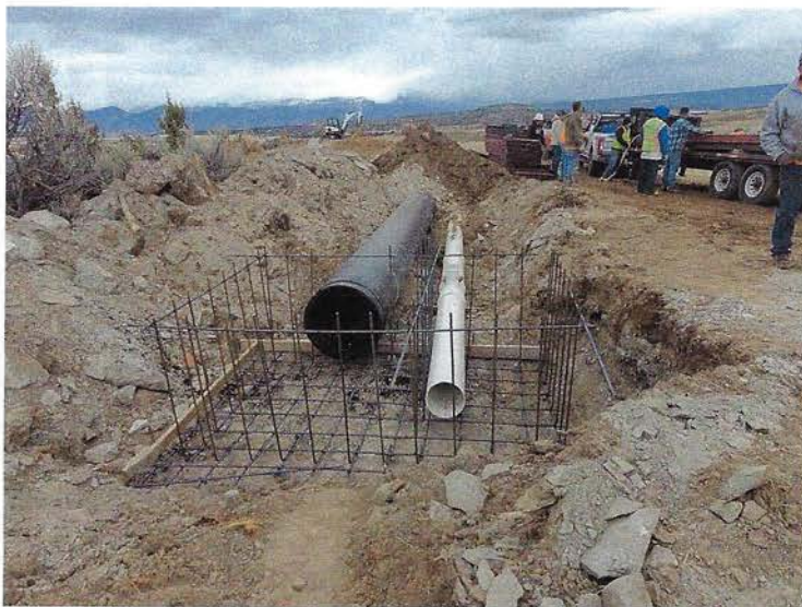
The two pipelines entering the outlet structure shown before forming and all rebar installed
