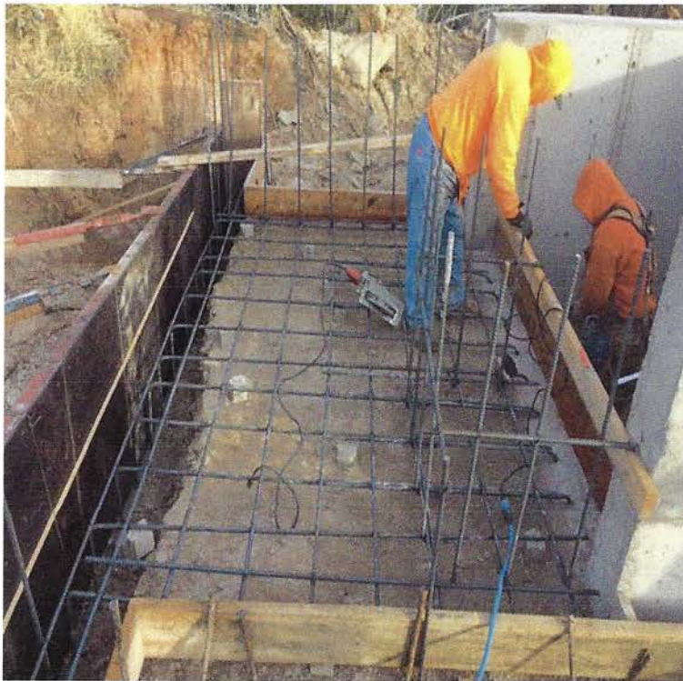
Forming and installing rebar for the inlet structure.
