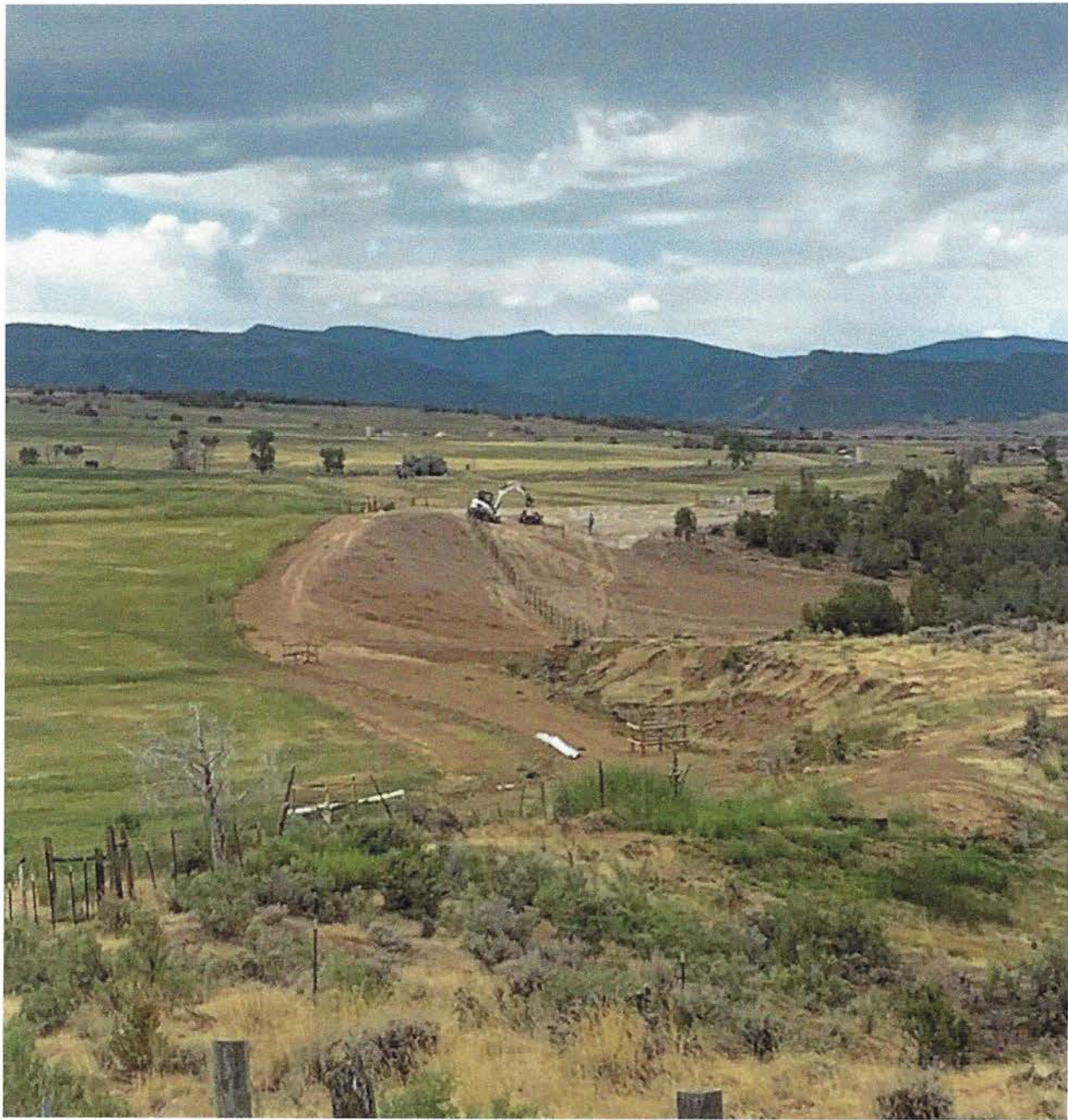
Completed grading and shaping for mulching and seeding, providing vegetative cover and growth.
