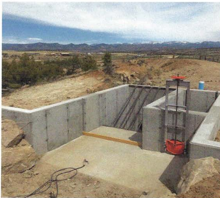
New inlet structure at the beginning of the pipeline, one side is for the main ditch, the other for Fazzi's fields.
