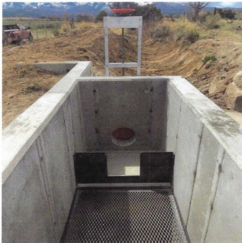
Inlet to Fazzi irrigation pipeline with measuring device and screen for cleaning.
