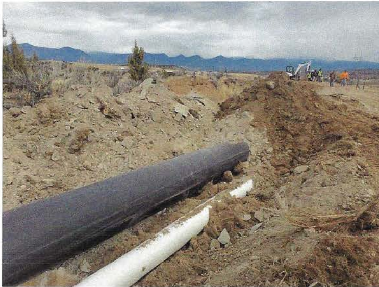
Installation of the two pipes, one HDPE the other PVC - PIP
