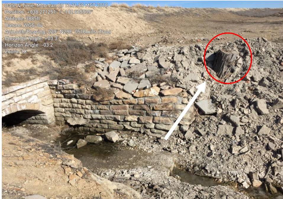
Photograph 3: 36-inch Diameter Tree Stump at Tunnel End Wall (red circle), Left Retaining Wall, and the outlet works.
