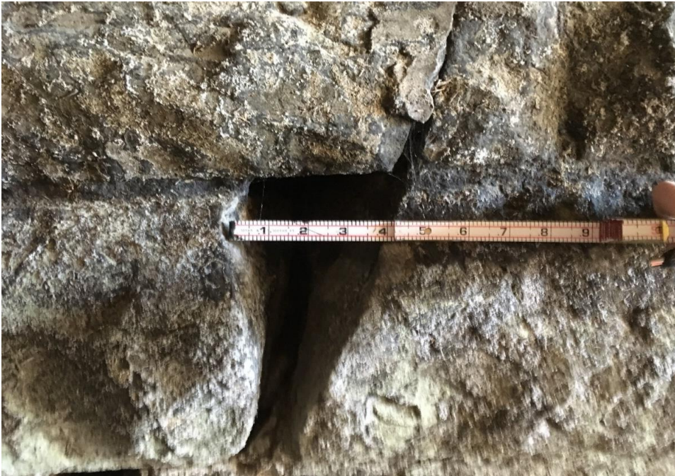
Photograph 6: Left tunnel wall void, 6 feet downstream of headwall.
