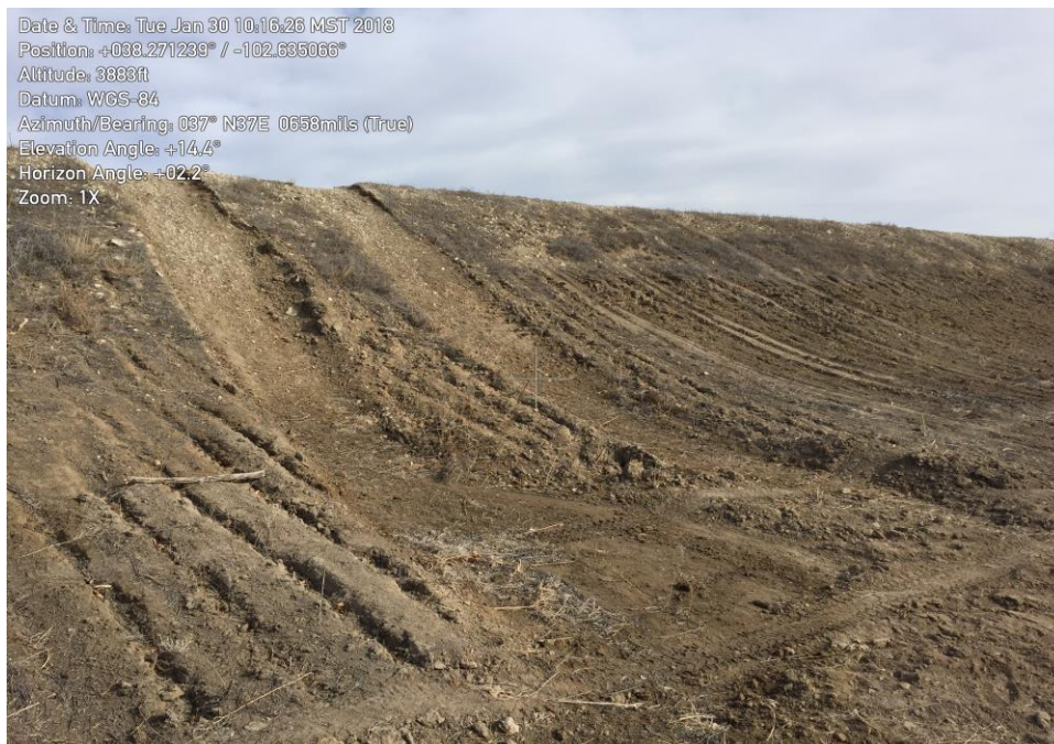
Photograph 2: Rutting on Downstream Embankment Slope (East of Outlet Works).
