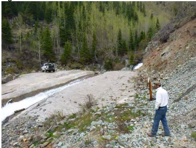
Figure 3-10 Boulder Creek raw water intake embankment dam
