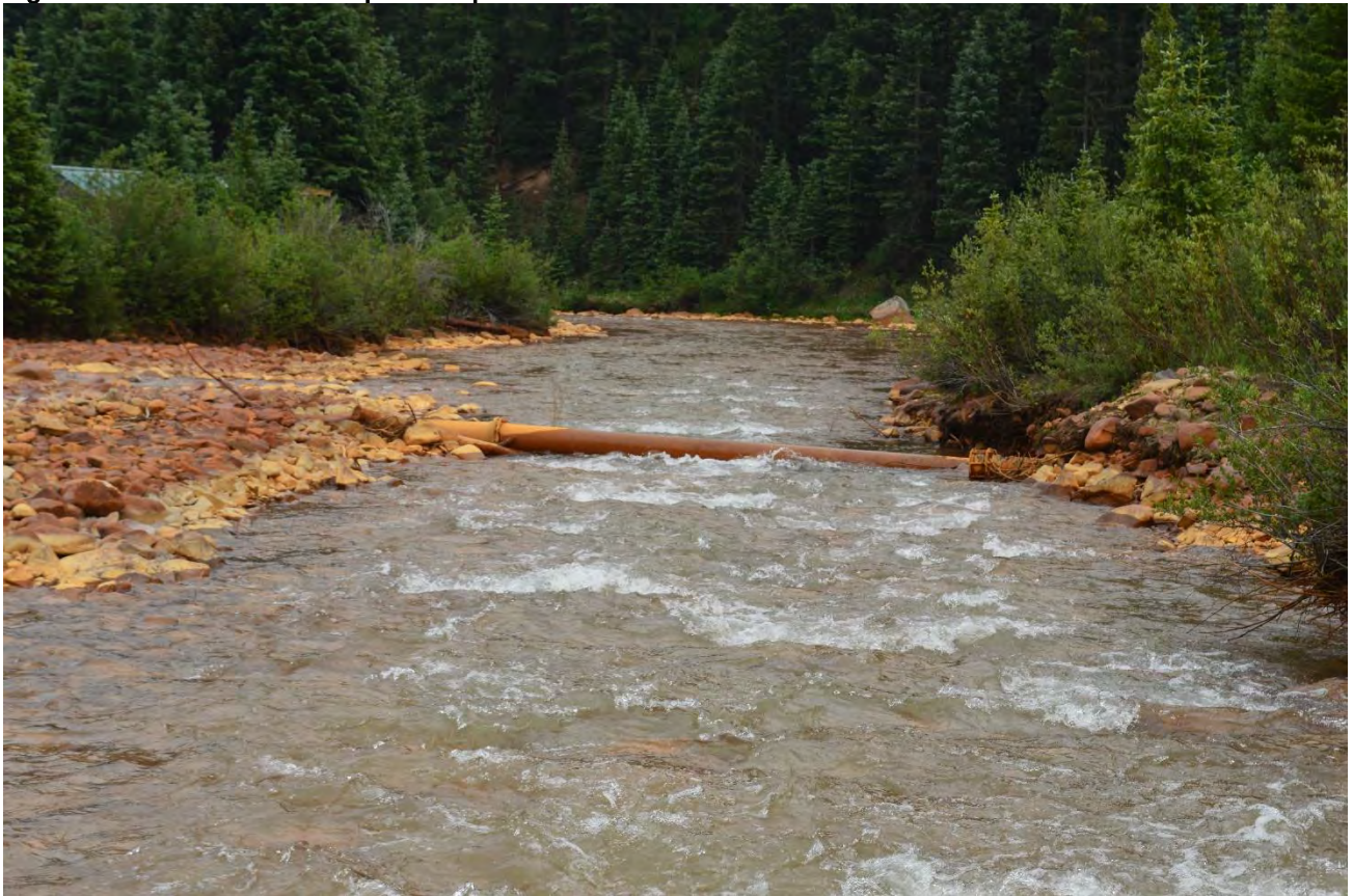
Figure 3-22 Mineral Creek Exposed Pipe
