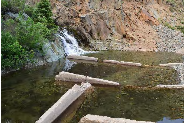
Figure 3-5 Shotcrete spillway and embankment
