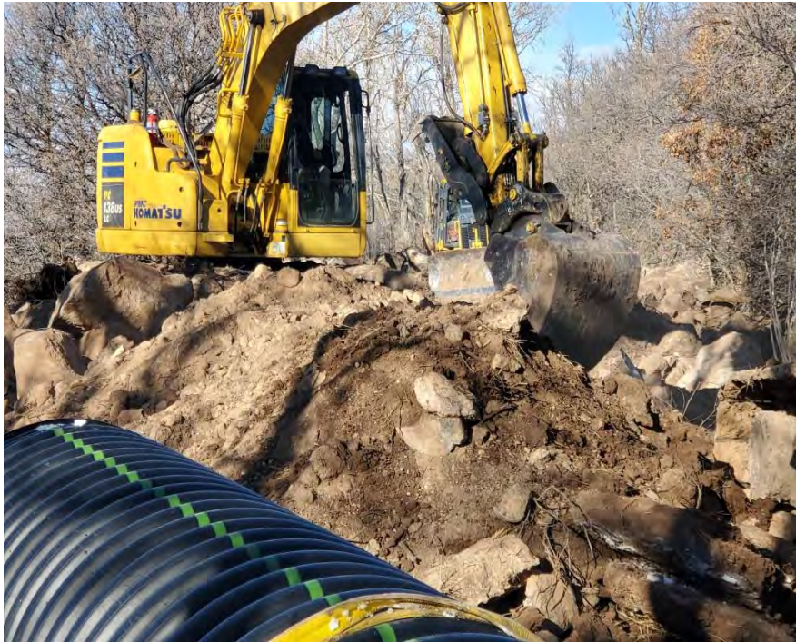
Excavator sorting large rock from finer materials to be used for bedding against the pipe.
