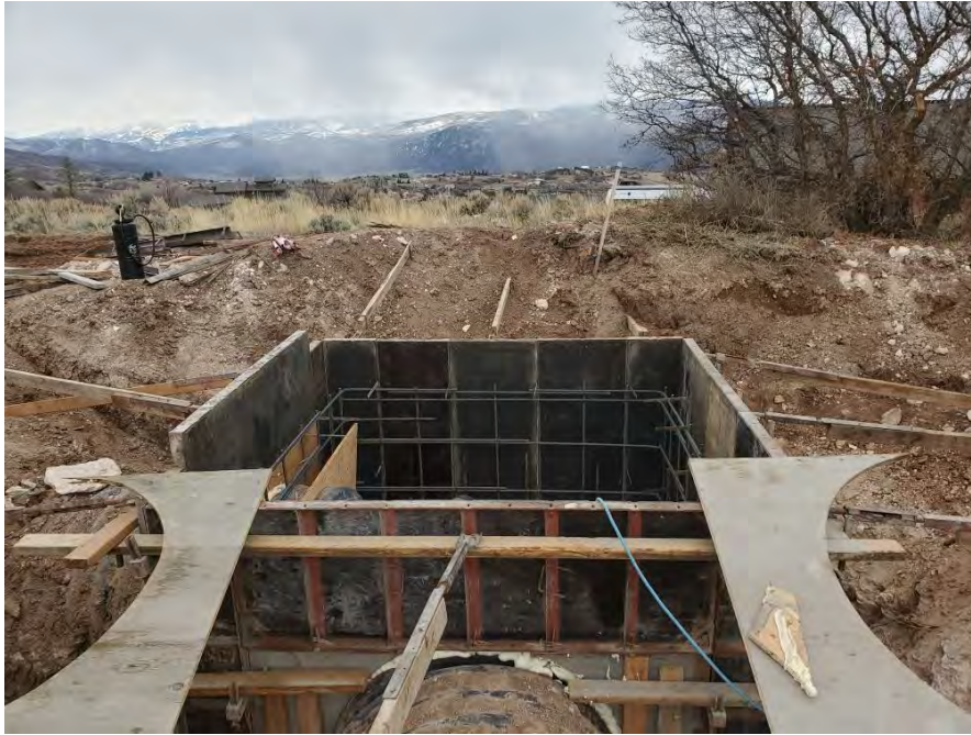
Forming of the connection box at the end of one of the section of pipe.
