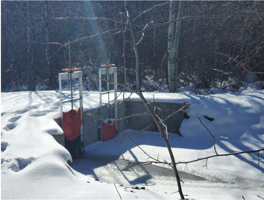
Splitter box for water to go to separate ranches.
