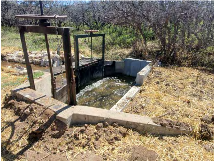
Another splitter box with water flowing after completion of the pipeline. Area has been smoothed, seeded and mulched as part of the final reclamation.
