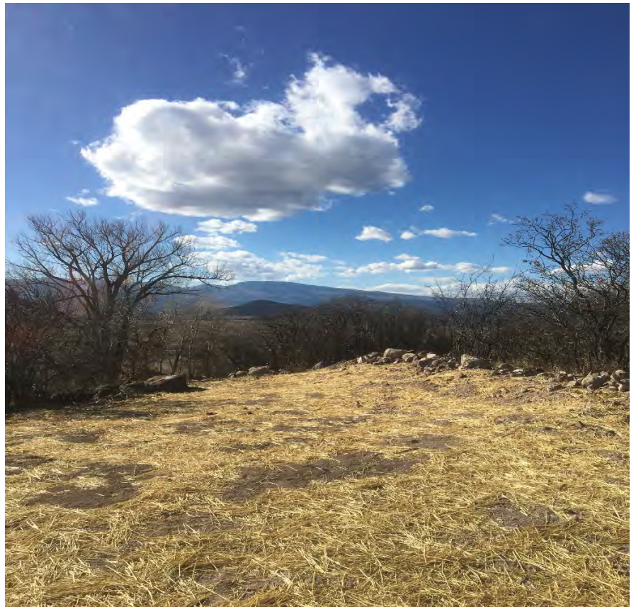
Buried pipeline after final grading, seeding and mulching of pipeline scar.
