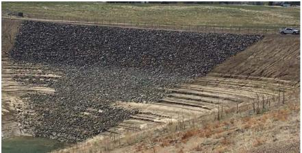
• Wave erosion undermining riprap
