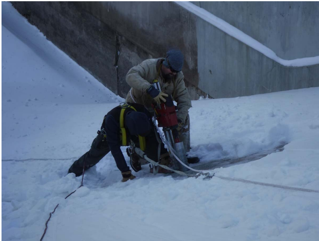
Photo 2: Coring through concrete slab
