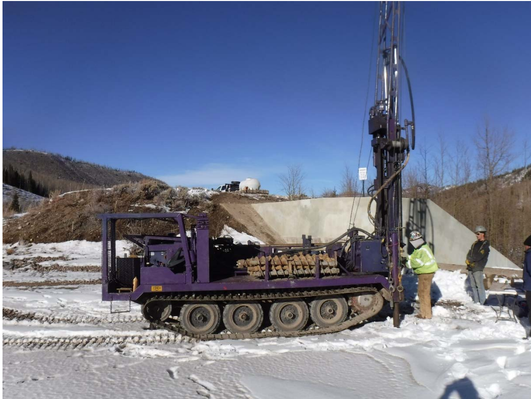
Photo 1: Track rig set up at borehole B2 upstream of the spillway apron
