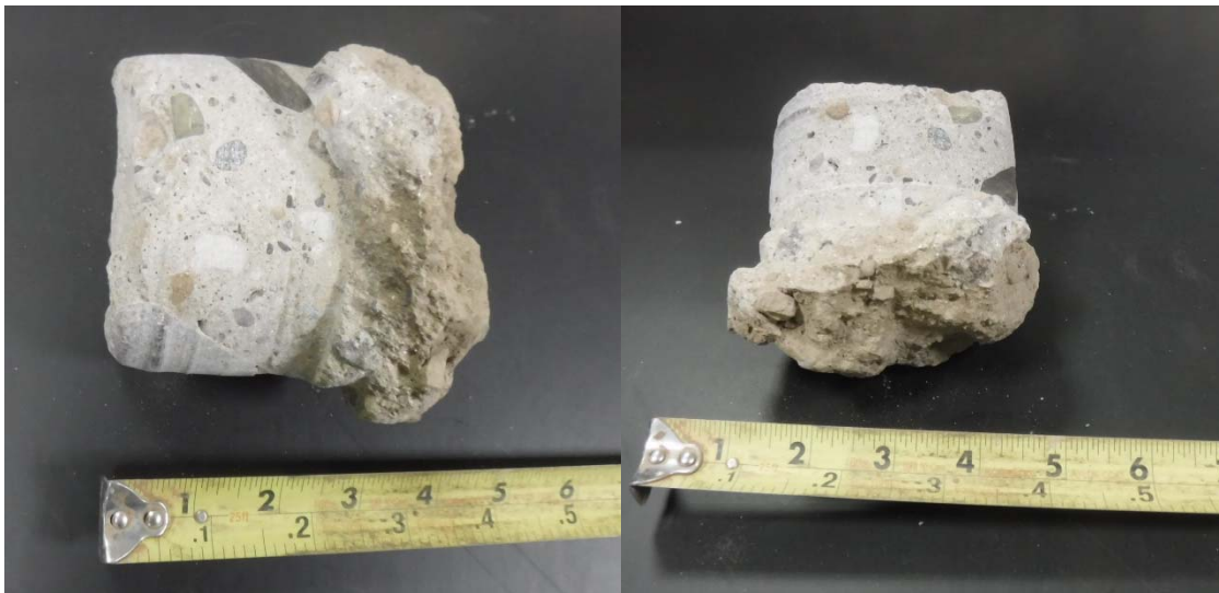
Photo 3. View of the mushroom shape of the concrete core removed from Core Hole 3
