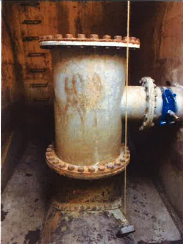
Photo 18: 30-inch by 16-inch tee installed in 1966 for water treatment plant modifications (looking west). Tee is tilted 1.5-inches north.
