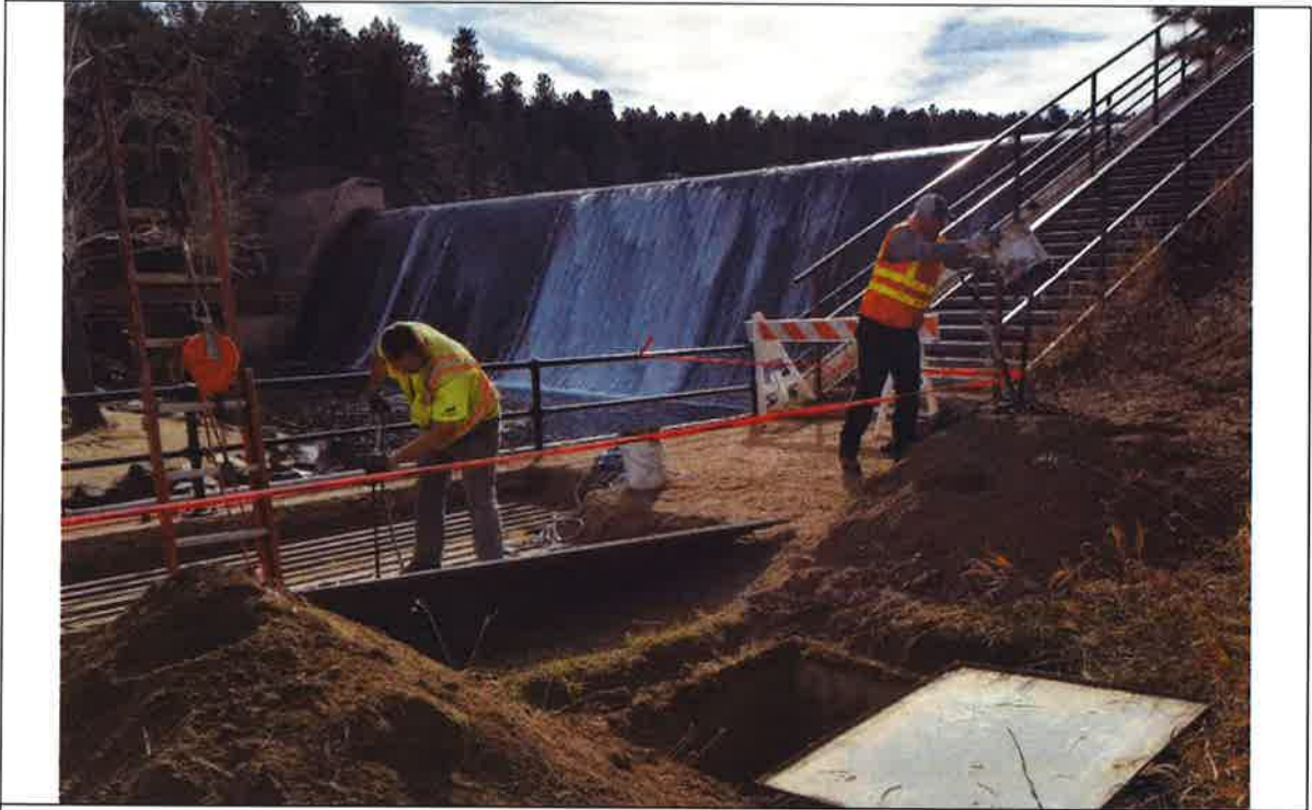
Photo 1: Evergreen Metro workers expose steel ribbing roof of the reservoir outlet vault. In the foreground the 16-inch water treatment plant valve vault is also open.
