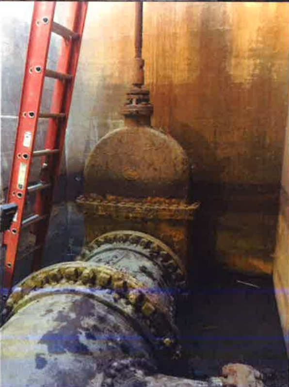
Photo 19: 42-inch to 36-inch reducer conduit and gate valve.
