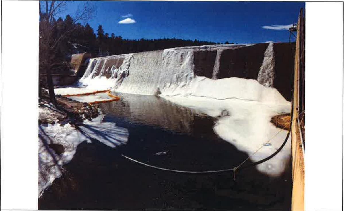
Photo 26: Sediment transport system from pedestrian bridge looking southwest. Date: 02-27-2019 Source: C. Masching (GEI)
