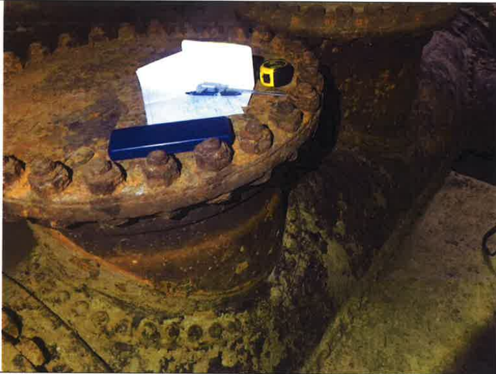
Photo 16: 30-inch blind flange with concrete fill to spring line of 42-inch conduit. Date: 12-07-2018 Source: C. Masching (GEI)
