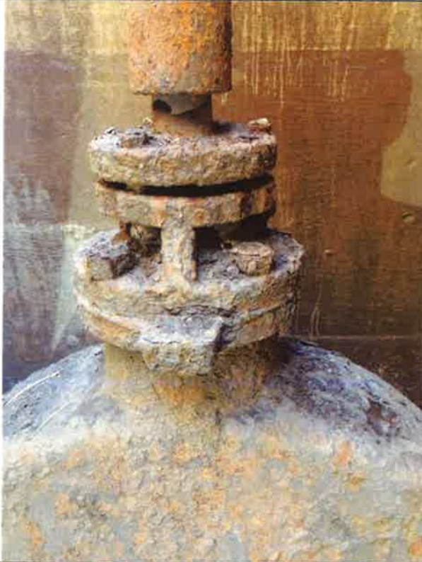
Photo 20: Gate valve mechanism above cover. Date: 12-07-2018 Source: C. Masching (GEI)
