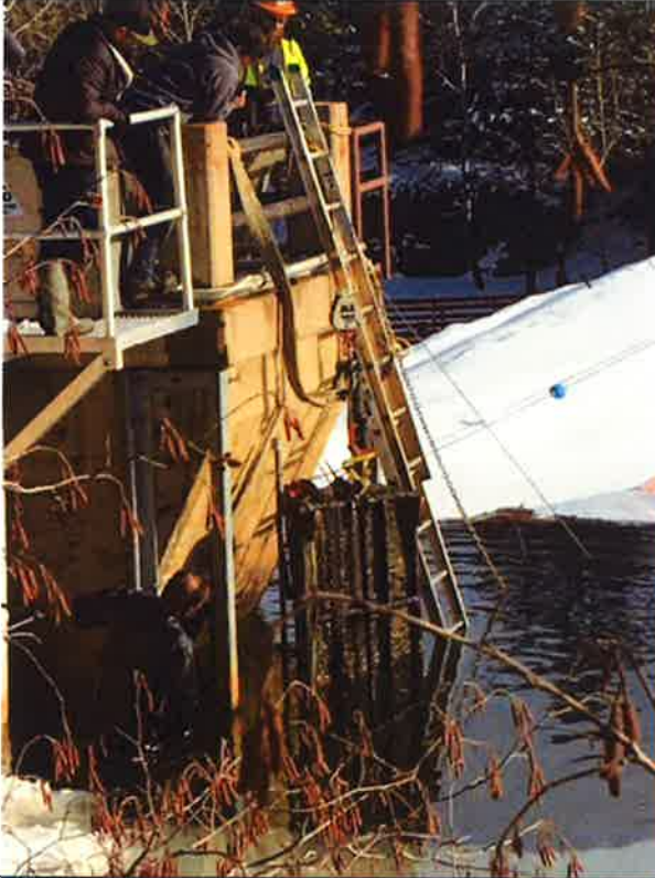
Photo 31: Removal of upstream gate leaf. Date: 03-05-2019 Source: C. Masching (GEI)
