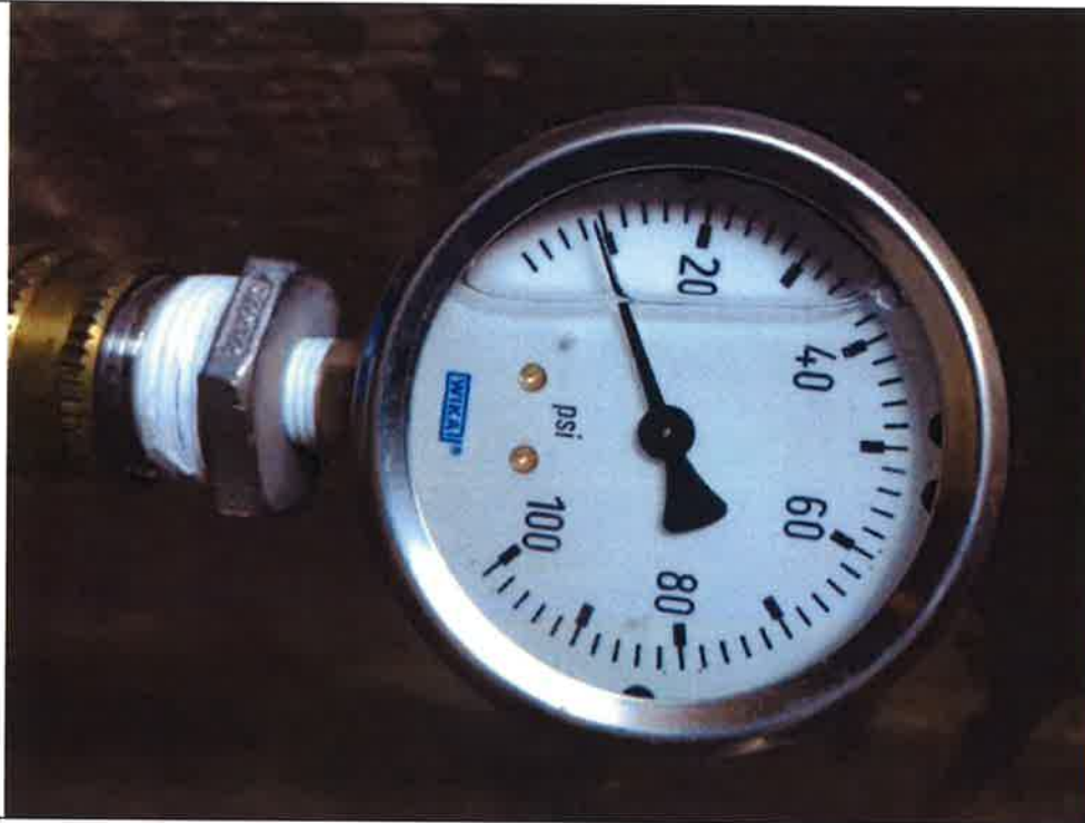
Photo 12: Wet tap gage on 16-inch line. Date: 11-15-2018 Source: G. Jeffrey (Evergreen Metro)
