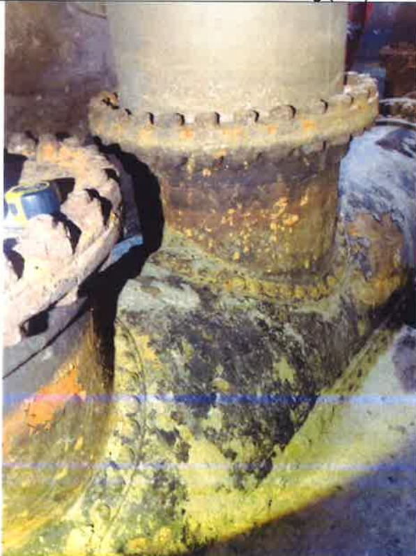
Photo 16: 30-inch blind flange with concrete fill to spring line of 42-inch conduit. Date: 12-07-2018 Source: C. Masching (GEI)
