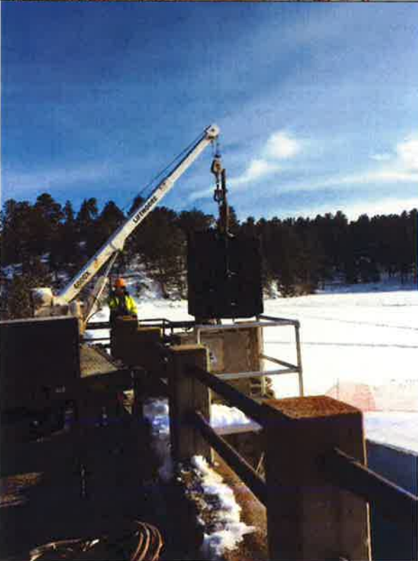
Photo 32: Additional view of gate leaf removed using truck-mounted crane. Date: 03-05-2019 Source: C. Masching (GEI)
