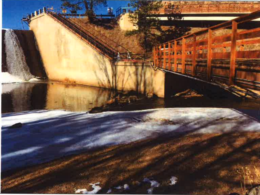
Photo 14: Left abutment and pedestrian bridge. Notice sediment at crest of outfall pipe. Date: 12-07-2018 Source: C. Masching (GEI)
