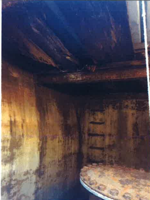
Photo 22: Steel members installed to support steel ribbing roof. Date: 12-07-2018 Source: C. Masching (GEI)
