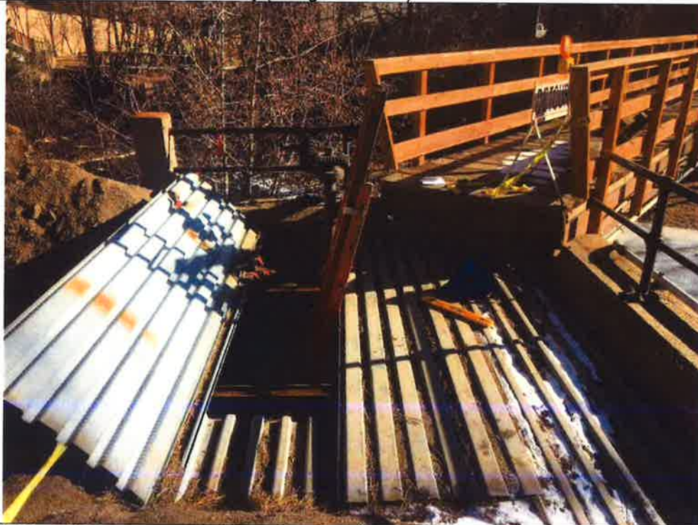
Photo 13: Steel ribbing over vault with steel beam support members running north-south. Valve operator is located above the vault, behind the ladder on the eastside of the vault. Date: 12-07-2018 Source: C. Masching (GEI)
