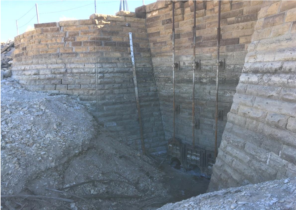
Photograph 1: Stone masonry upstream dam face and slide gates.
