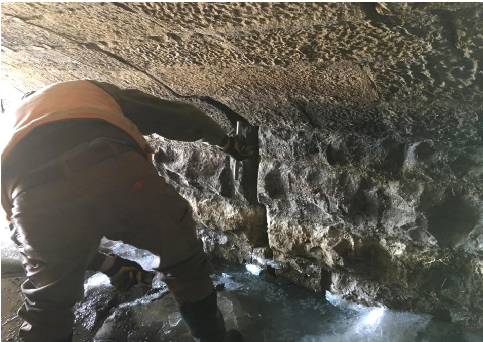
Photograph 7: Right tunnel wall void, 5 feet downstream of headwall.
