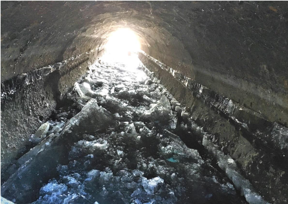
Photograph 3: 30-inch diameter riveted steel outlet conduit.
