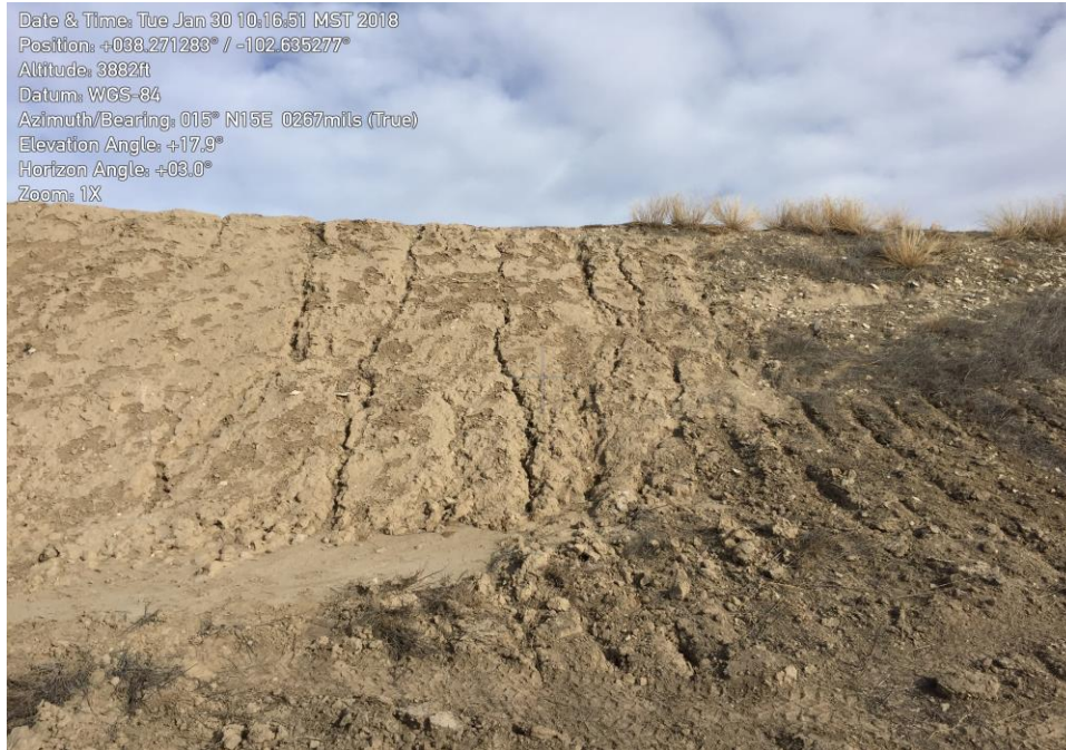
Photograph 1: Erosion Rills on Downstream Embankment Slope (East of Outlet Works).
