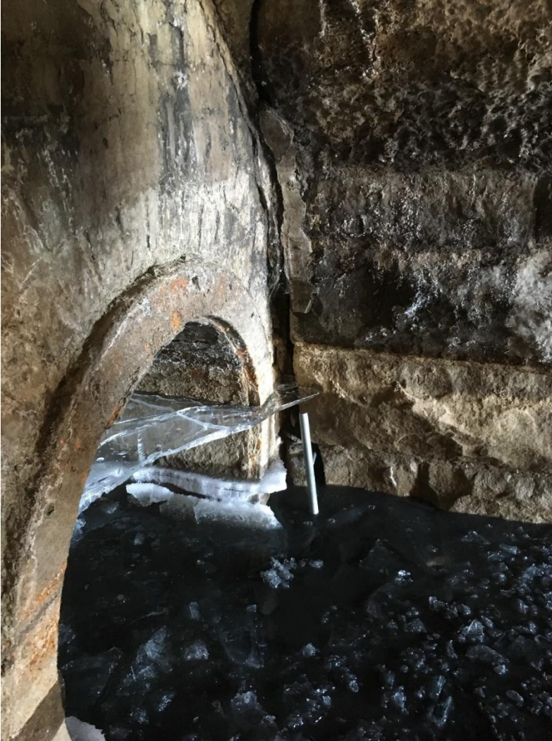
Photograph 5: Void between conduit headwall and left tunnel wall interface, showing soil probe in void
