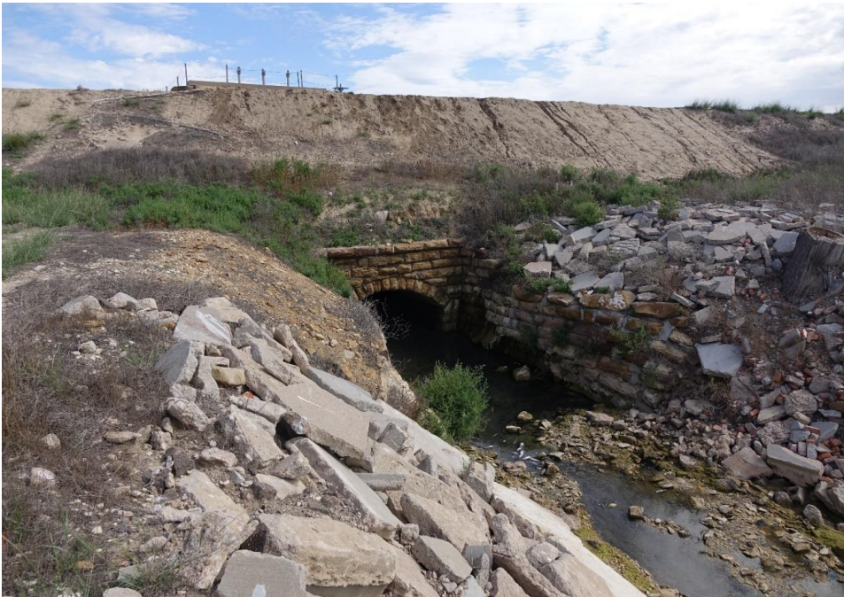
Photograph 2: Stone masonry downstream retaining walls.
