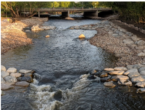
Drop structures/slope protection and willow plantings/bio-stabilization
