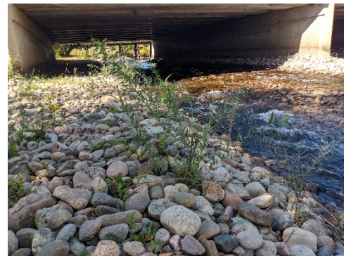
Drop structures/slope protection and willow plantings/bio-stabilization
