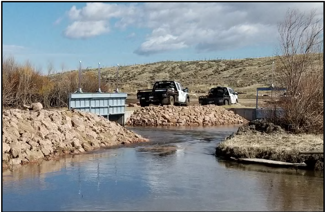
Upstream view of the new diversion and headgate, along with the rock streambank protection.
