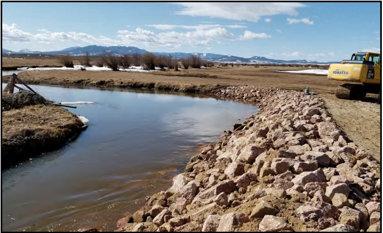
Rock rip rap along the upstream bank of the structures.
