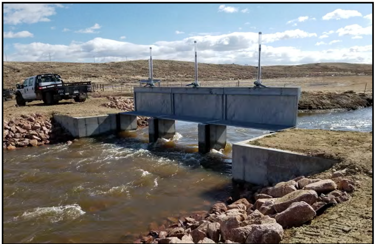
Rear view of the diversion and armored rock chute.
