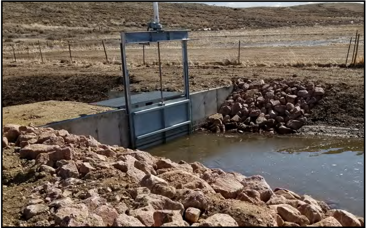
Front view of the finished 6 foot headgate and armored banks.
