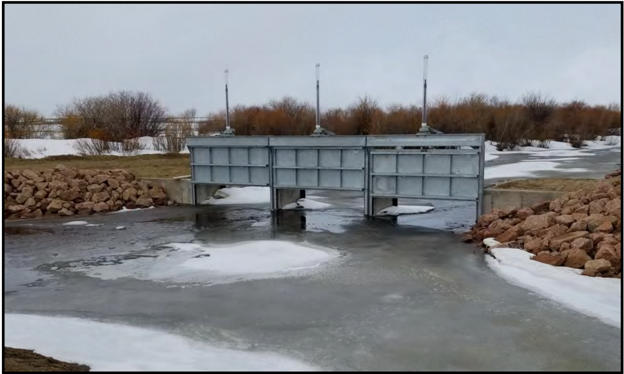
Front view of the finished diversion. The (3) 8 foot screw gates with concrete support structure and rock protection.
