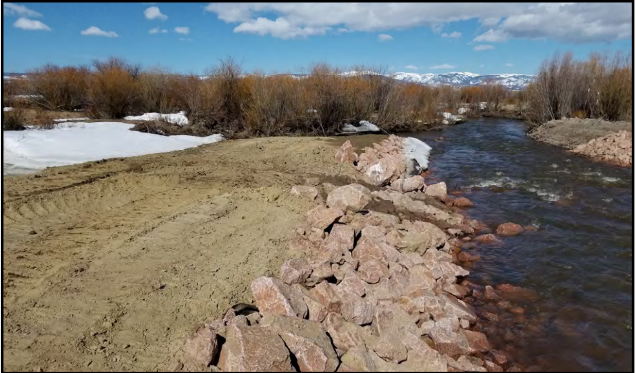
Additional rock rip rap on the stream channel.
