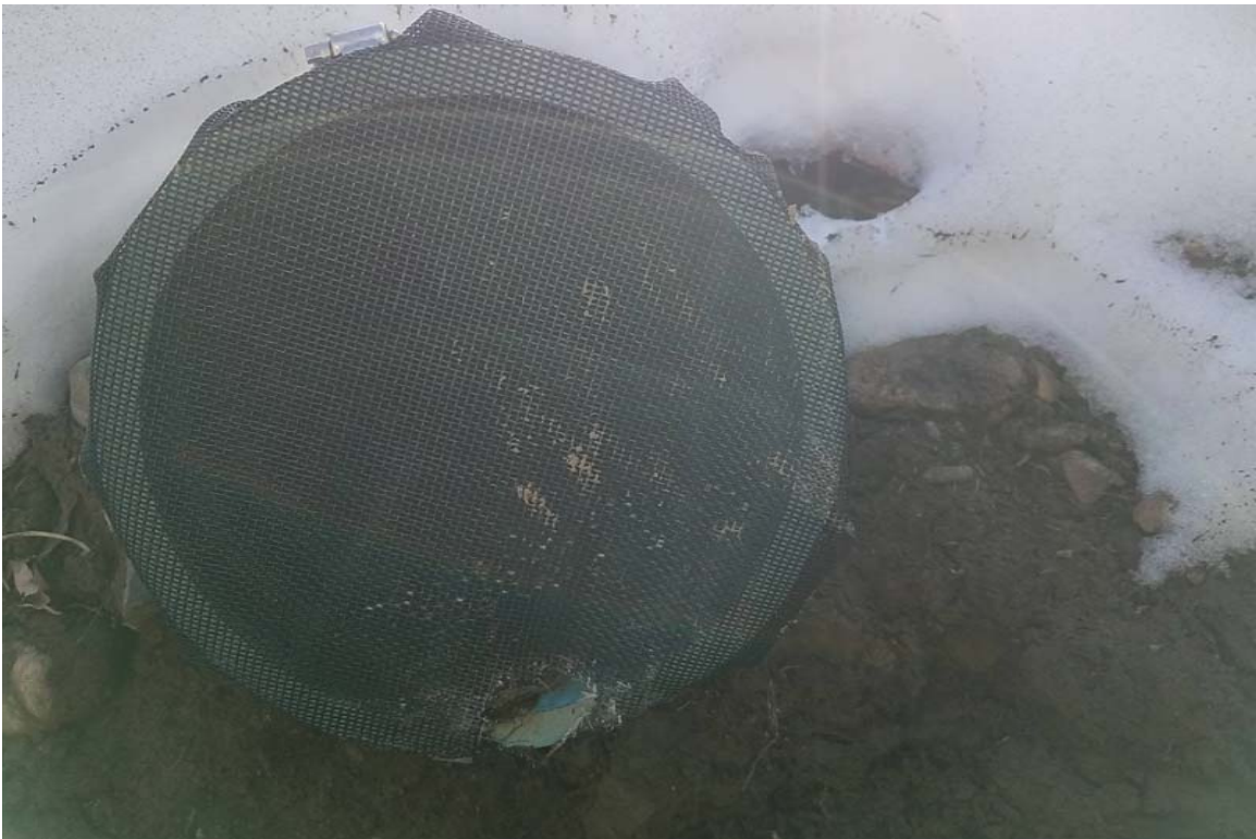
Toe drain Outfall #1 with rodent screen. Note hole in screen
