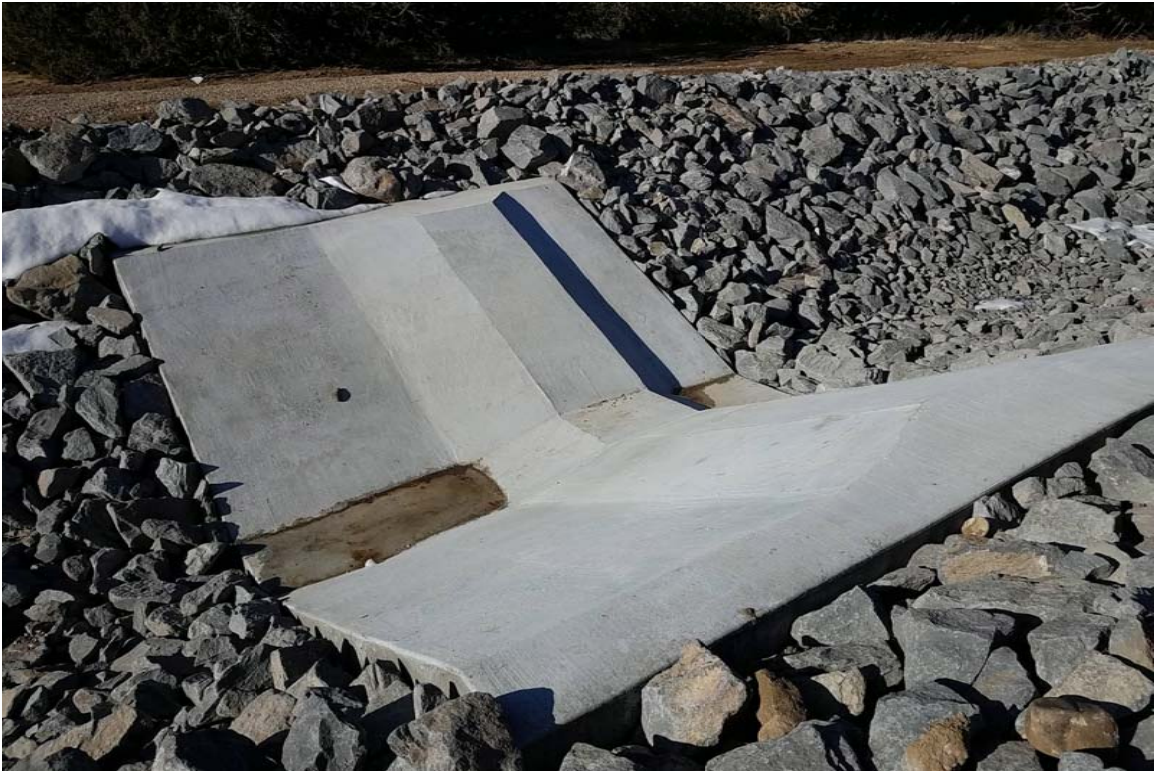
Completed reconstruction of outlet discharge channel ramp flume
