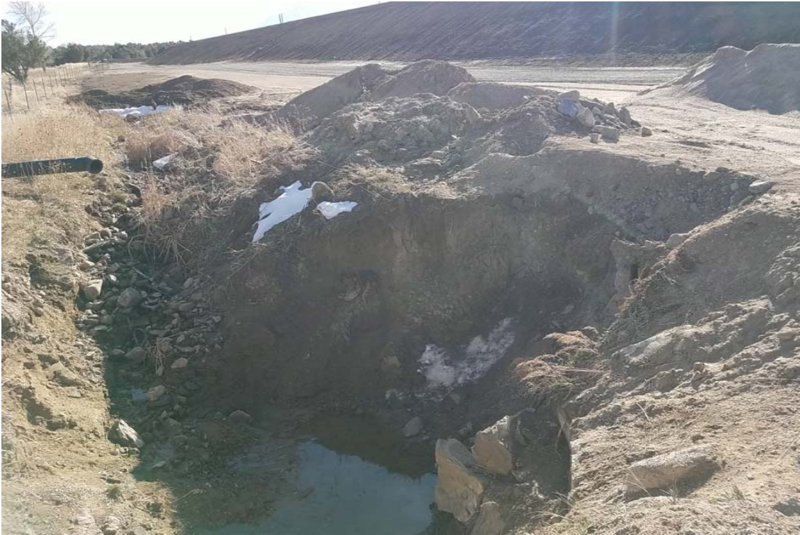
Excavation at water supply line to sand wash plant needs to be backfilled and reclaimed
