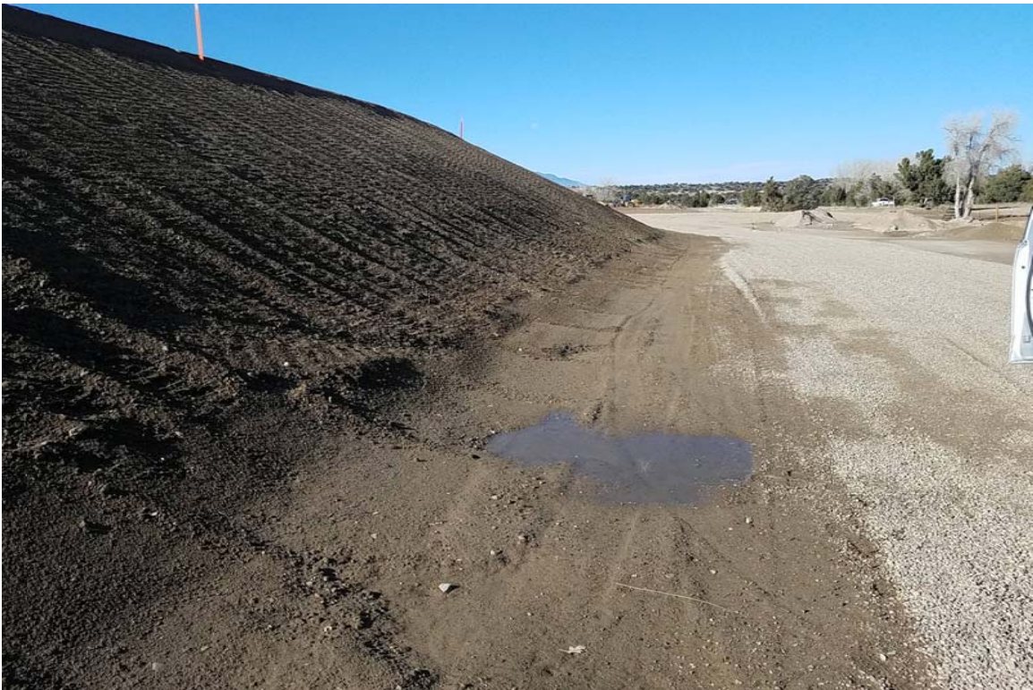
Minor regrading needed along downstream toe
