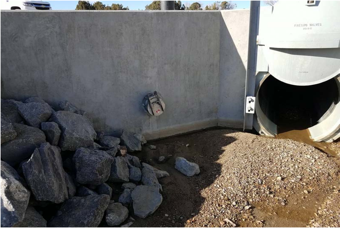
Toe drain Outfall #2 at Coler Ditch pumpback control structure
