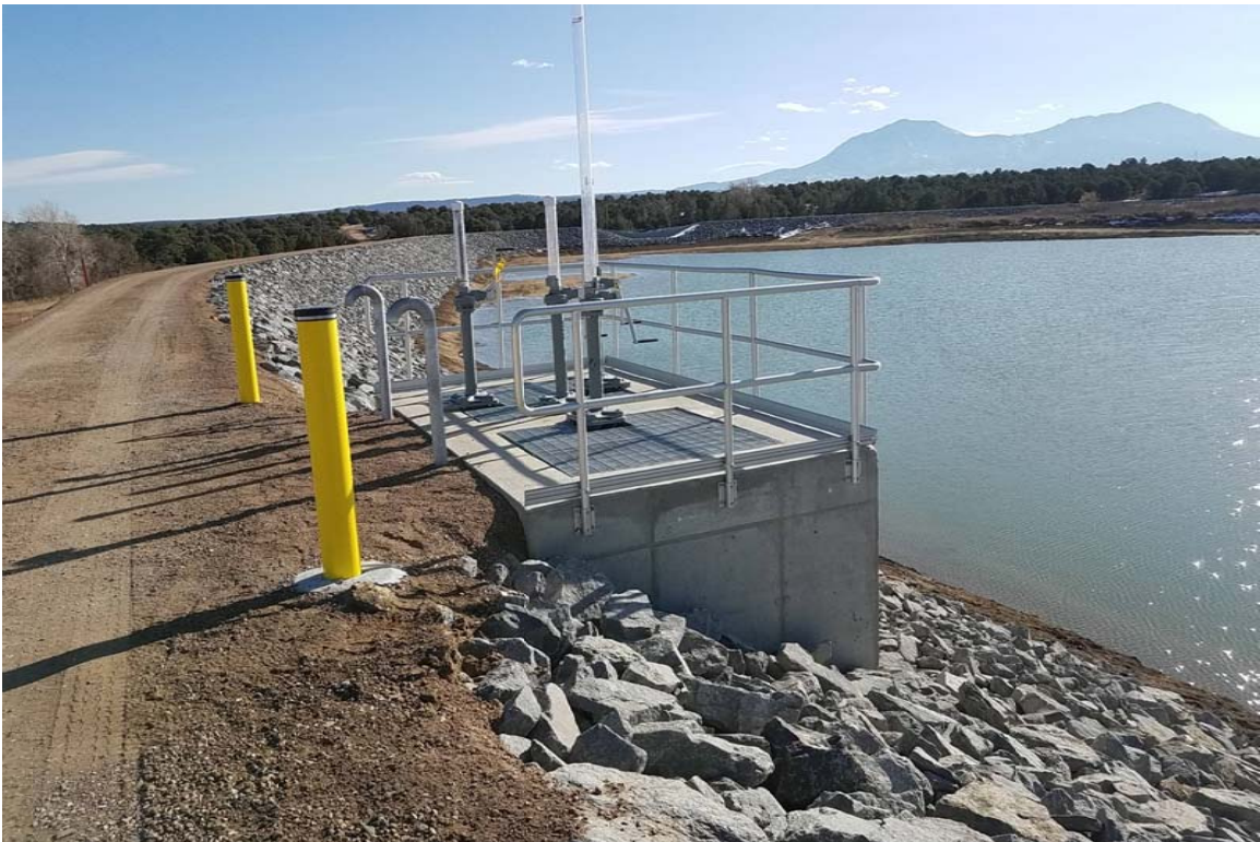
Outlet valve tower and bollards
