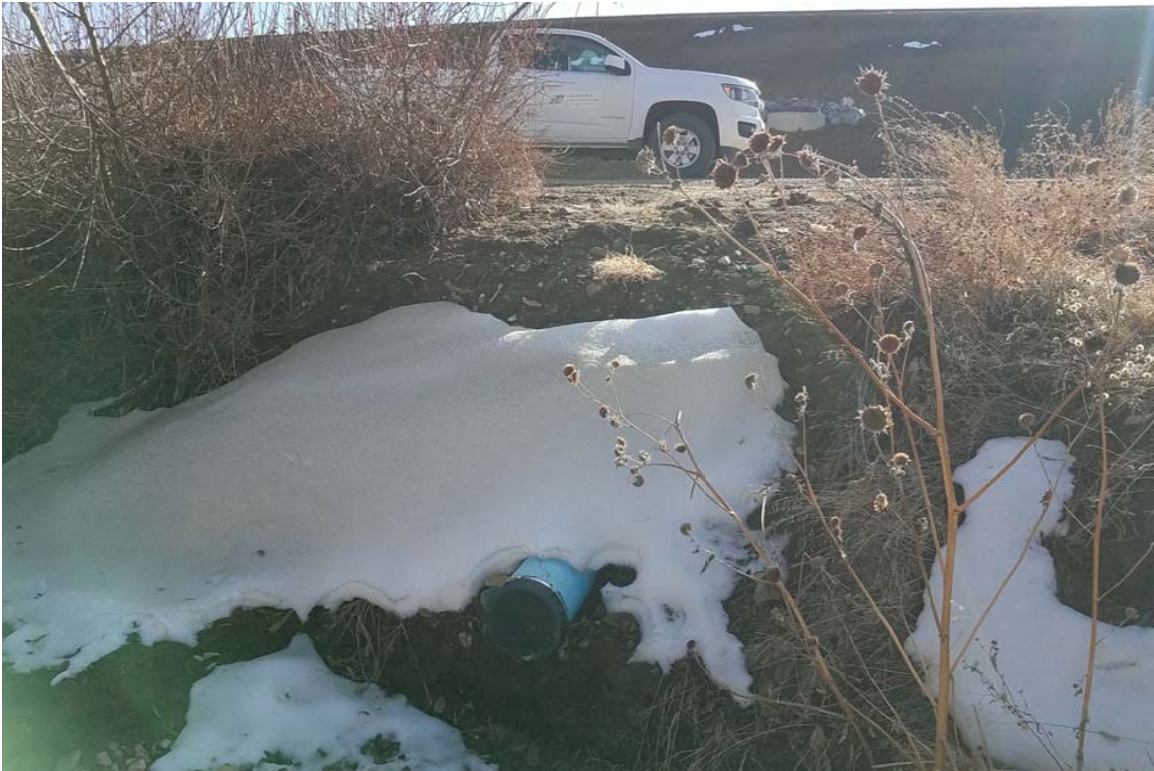
Toe drain outfall #1 (north end) with rodent screen and excavated outfall to allow measurement
