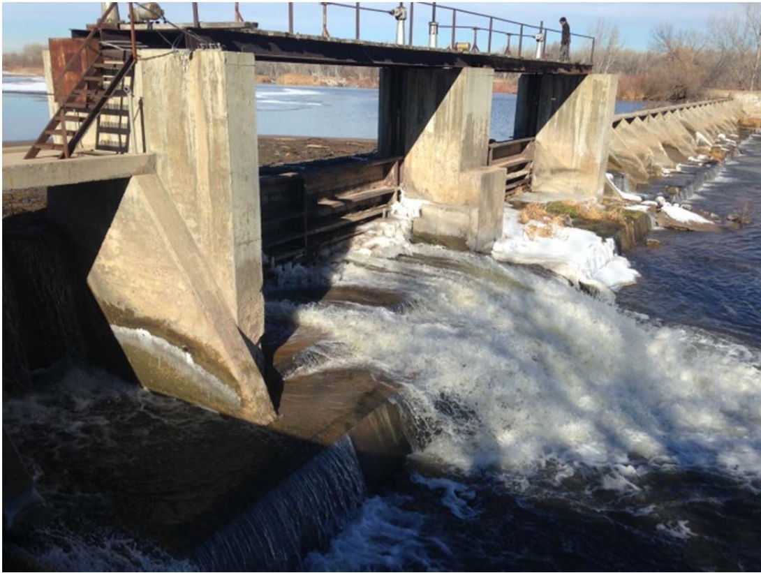
Fig. 9: Vertical gates, south section (looking upstream).
