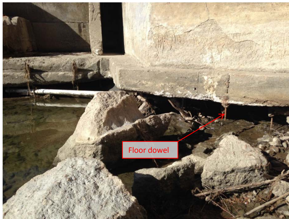
Fig. 1: Undermining and exposure of floor dowels, north section.
