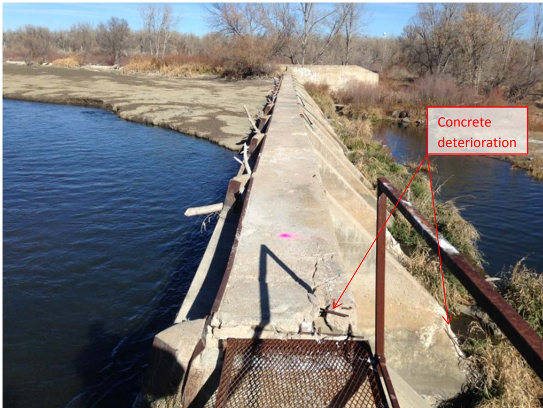
Fig. 7: South section buttress wall (looking north).
