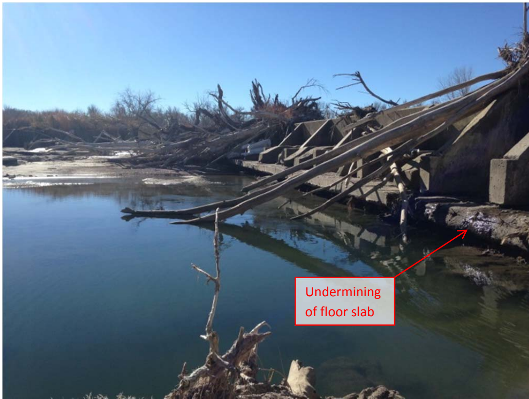
Fig. 3: North wall of structure (looking south).
