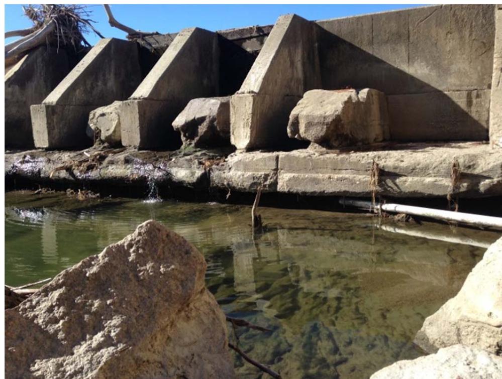
Fig. 2: Flash board bays, north section (looking upstream).
