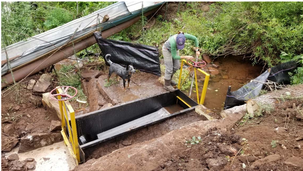
After: new fish screen installed
