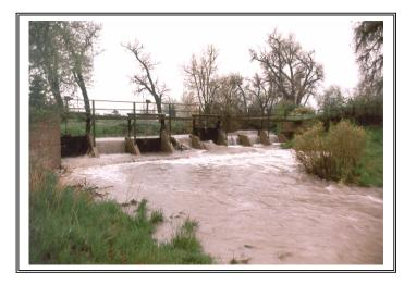
In evaluating the interaction irrigation ditches with а major drainageway for purpose of basin delineation, the ditch should not be utilized as a basin boundary due to the limited flow capacity of the ditch. The ditches will generally be flowing full or near full during major
