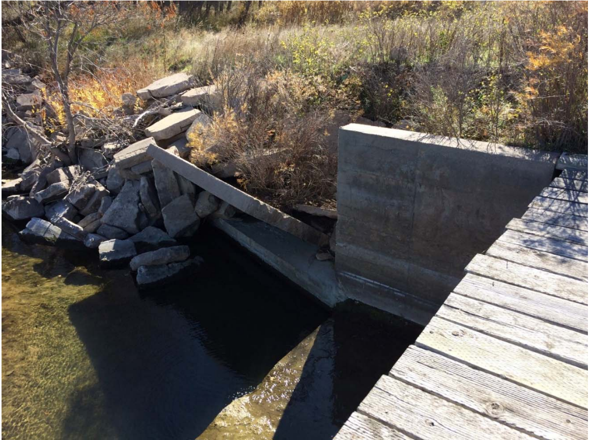
PHOTO 3 - RIGHT (SOUTH) ABUTMENT BLOWOUT
