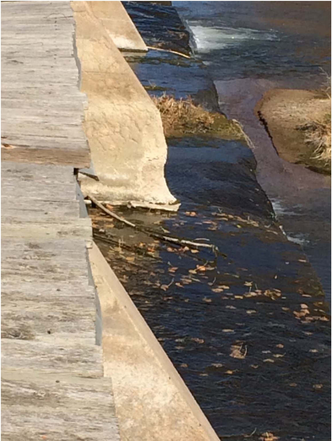
PHOTO 4 – DIVERSION STRUCTURE DETERIORATED CONCRETE
