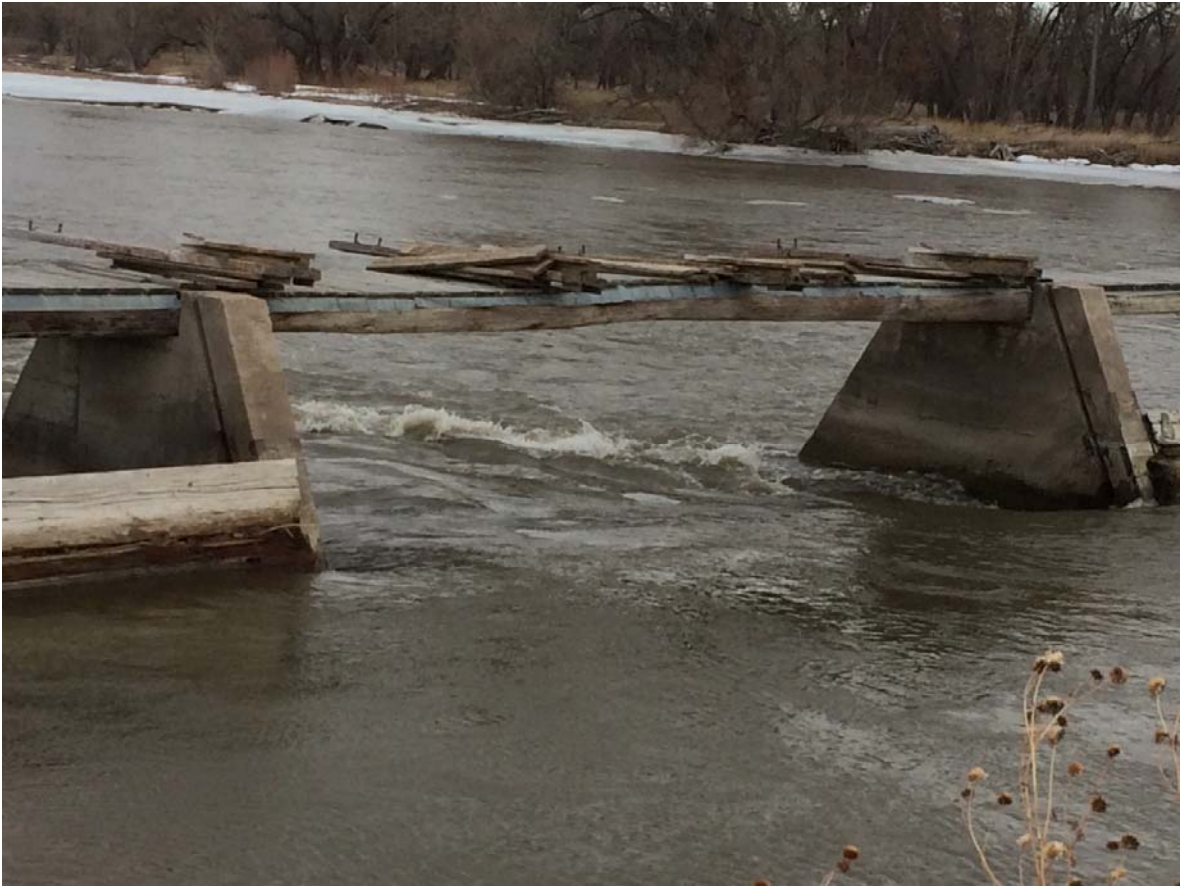
PHOTO 5 – DIVERSION STRUCTURE DURING WINTER OPERATIONS (CHECK BOARD REMOVED)
