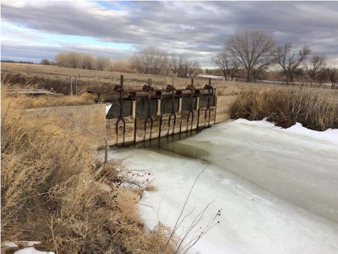
PHOTO 6 DITCH GATE STRUCTURE DURING WINTER OPERATIONS
