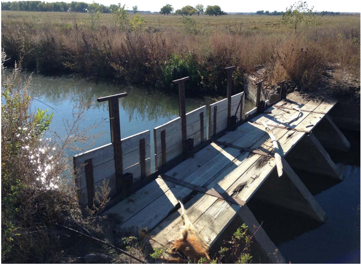
Fig. 5: Head gate structure, looking west.
