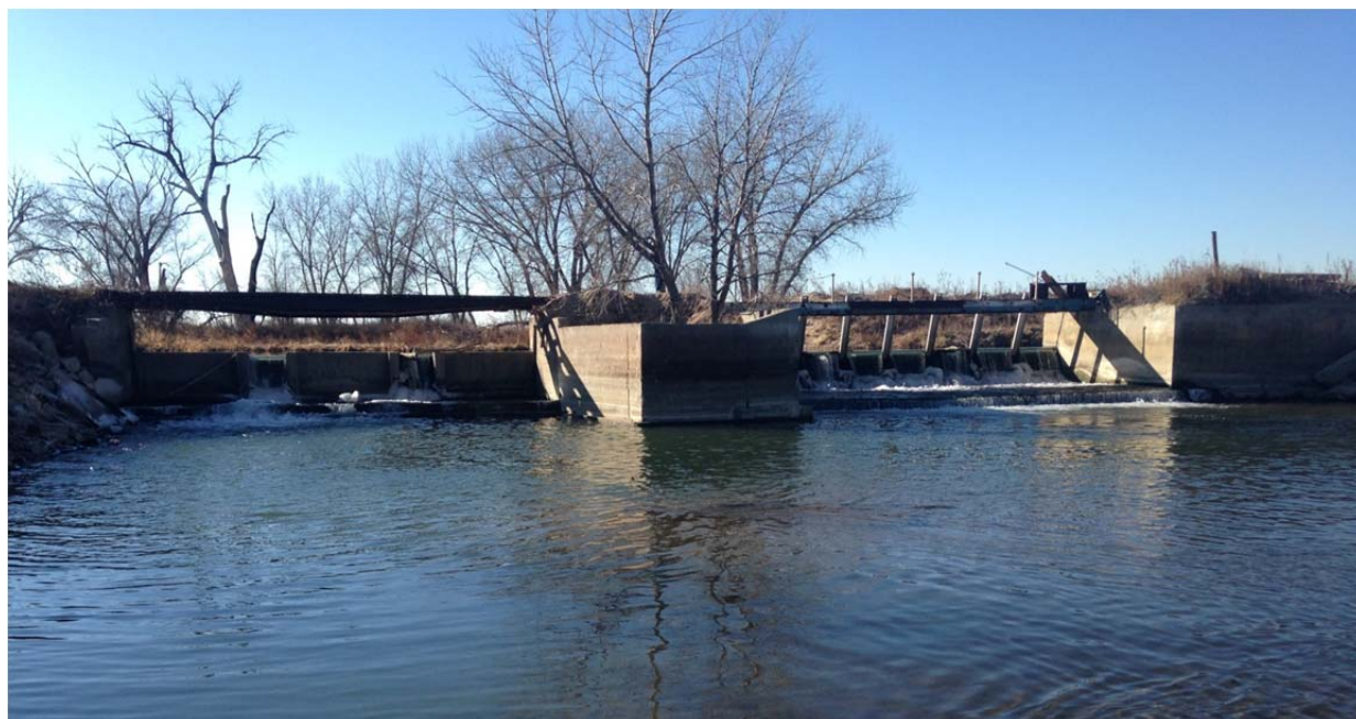
Fig. 1: Diversion structure, looking upstream.
