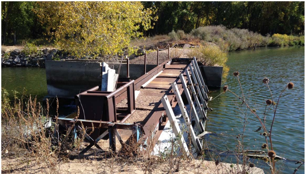
Fig. 4: North gated sand chutes, looking south.
