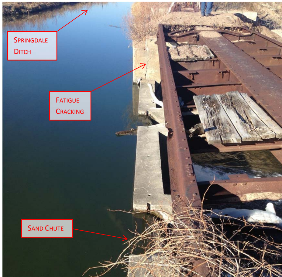
Fig. 3: South flash boarded sand chutes, looking north.
