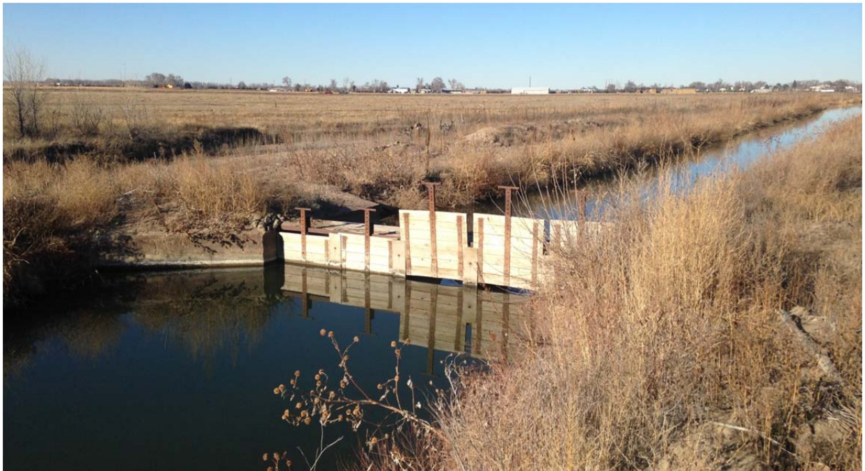
Fig. 6: Head gate structure, looking north.
