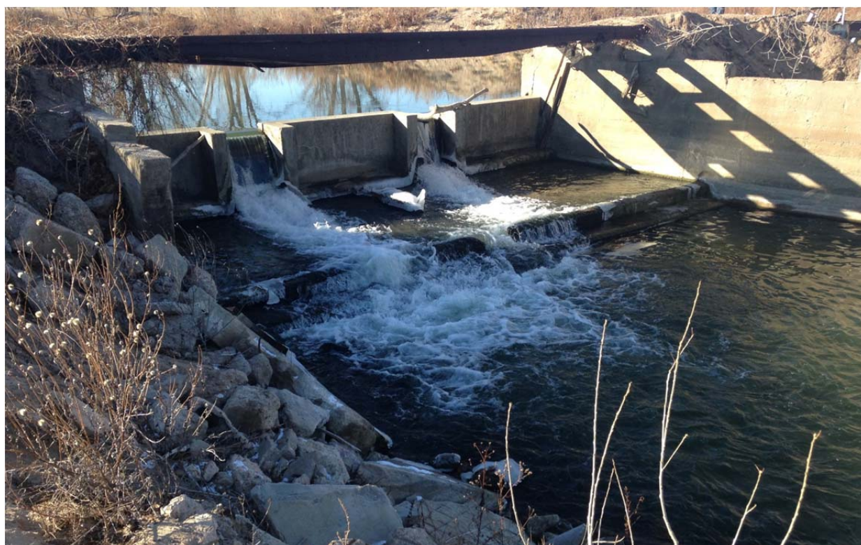
Fig. 2: South sand chutes, looking upstream.
