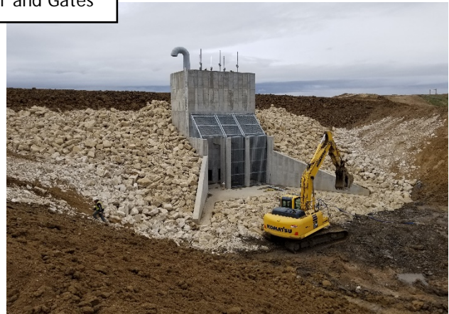
Outlet Tower and Gates
