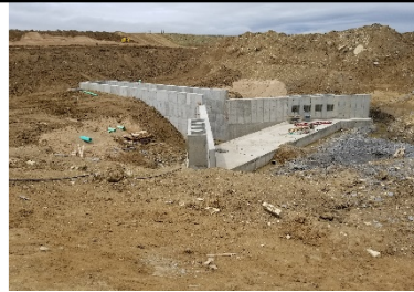
Construction of Mud Mat and Outlet Terminal Structure
