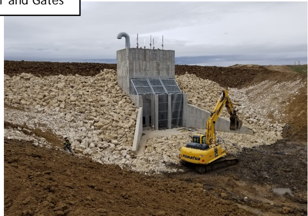
Outlet Tower and Gates
