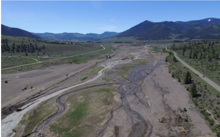
Figure a. June 12, 2019 Aerial photo depicting impacts from snowmelt runoff. Please note return of creek from engineered single channel to braided stream.
