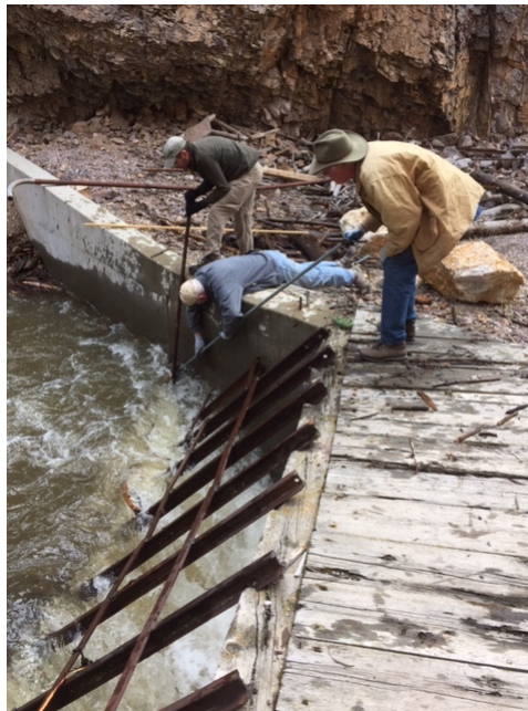
Figure c. June 5, 2019 Grizzly at the Amethyst mine before and after debris cleanup by Headwaters Alliance and WCRC volunteers just prior to runoff event.
