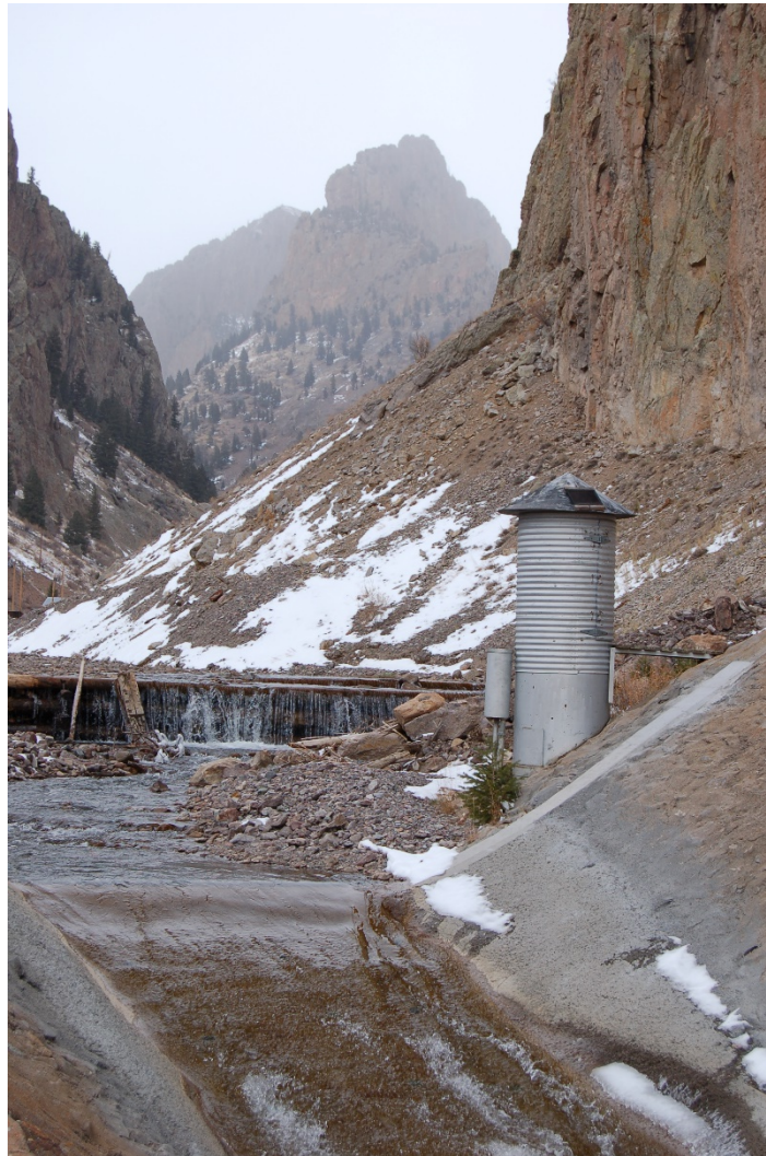
Figure h. Water Gage at the top of the flume. The gage has been inactive since 1987. Without accurate reading of cfs flow volumes during high water events, concern of impacts during high water events cause uncoordinated response actions due to the lack of accurate data. Additionally, the lack of data on Willow Creek has made the floodplain map revision process long and arduous.
