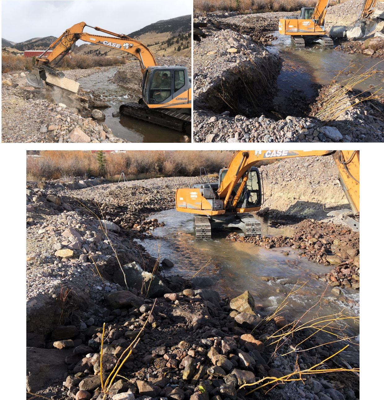
Removal of debris and concrete (upper left) during initial structure installation followed by excavation and willow cutting installation (upper right). Bottom middle photo shows final product including 5 large boulders and over 30 cuttings.
