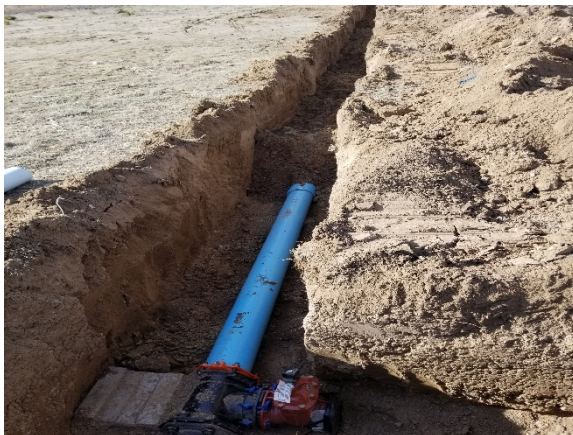
Completed well field piping for Well Nos. 12 and 13.
