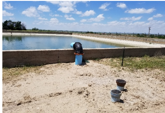
Completed installation of bypass piping for the open water reservoir used as a source of irrigation water for the piped distribution system.
