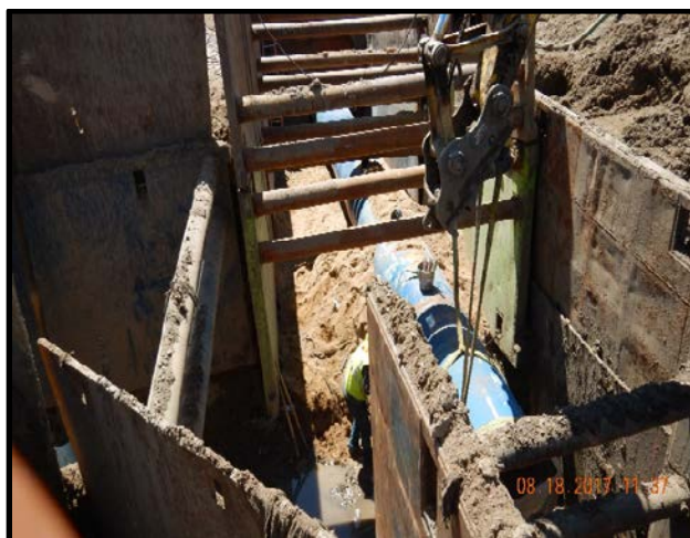
Photos show installation and welding of the new pipeline near Rueter-Hess Reservoir. The pipeline extends from Chambers Road and E-470 to the Parker Water Treatment Plant south of Rueter-Hess Reservoir.
