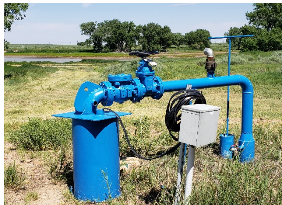
Completed pump installation for Well No. 47.
