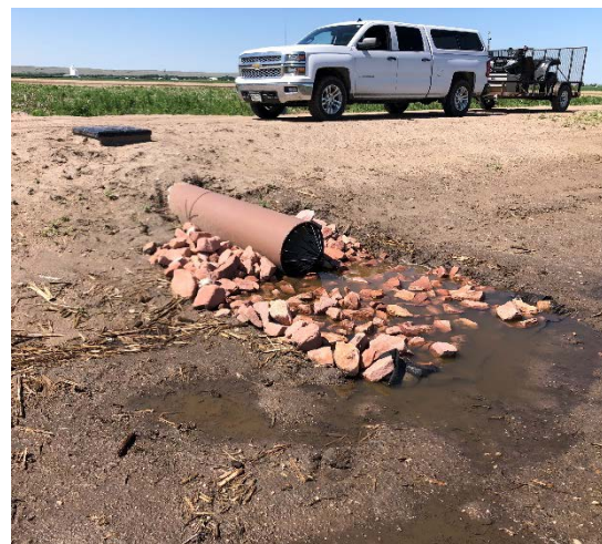
Picture 2- Agri-Drain installed in East Pond embankment
