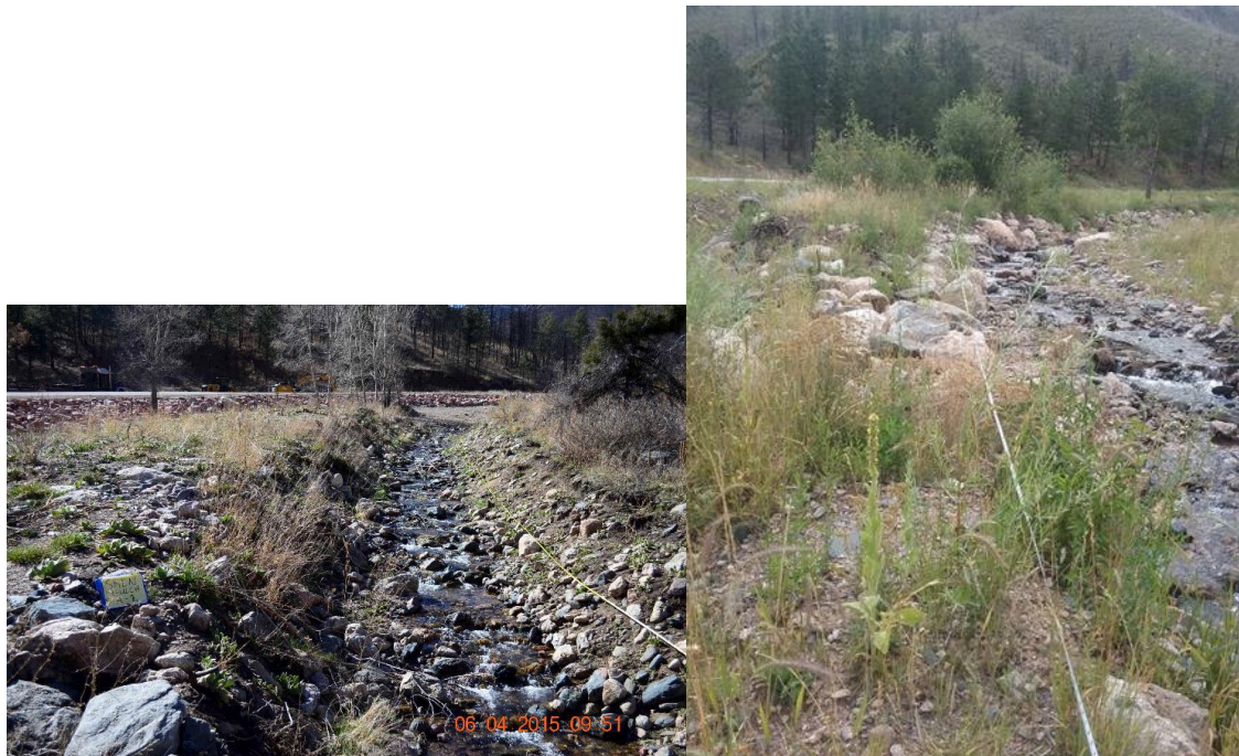
Figure 6. Reach A, middle section. Left: pre-restoration; 2) post-restoration August 2016
