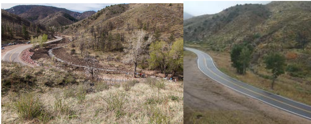
Figure 7. Skin Gulch Reach A, viewed from downstream end. Photo on the left - channel construction complete, prior to first volunteer planting day, spring 2015. On the right: after all construction and planting complete, fall 2016.
