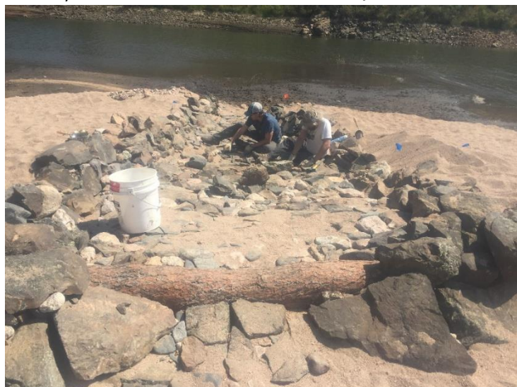
Figure 4. Installation of rock structures & log weirs in delta channel to stabilize the channel at Seaman Reservoir
