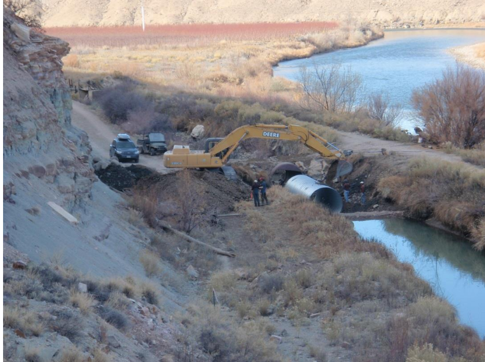
Replacing old culvert/crossing
