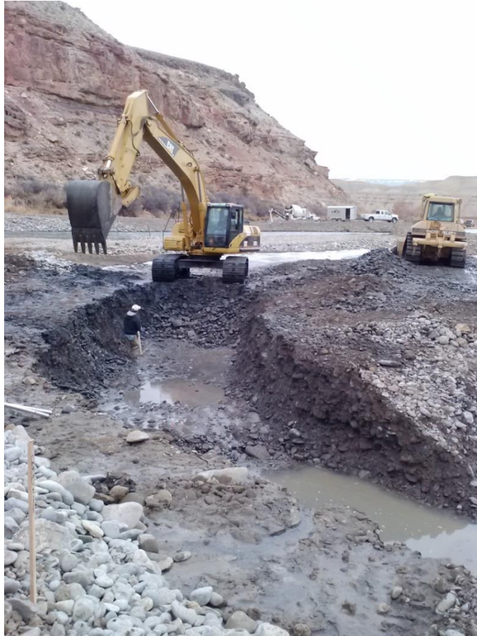
Excavation for weir foundation
