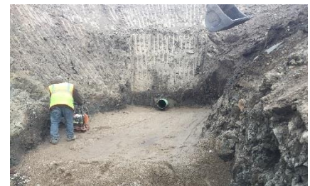
FIGURE 3 FOUNDATION DRAIN CONSTRUCTION
