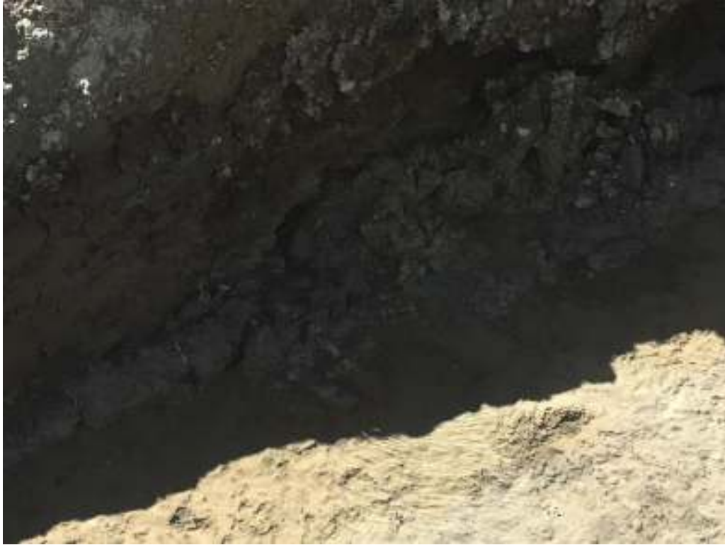
Photo 3 Seepage from sides of Excavation
