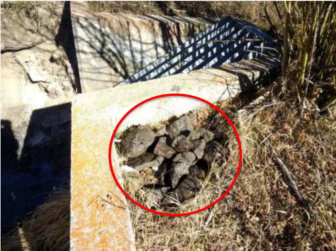
Figure 6: Rocks Removed from 30" CMP
