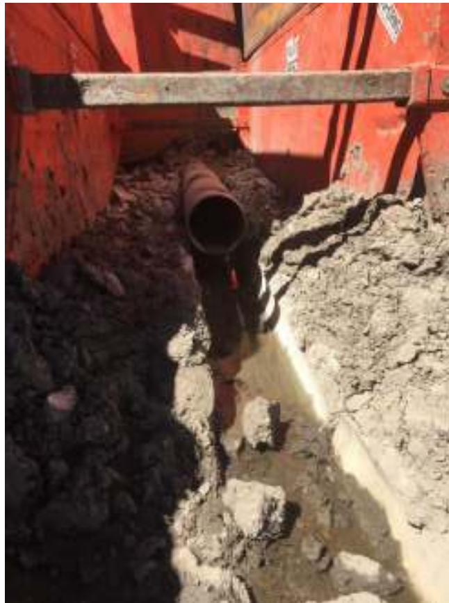
Photo 6 Trench sta 1+14 to 1+44, one stick of pipe remains to be removed
