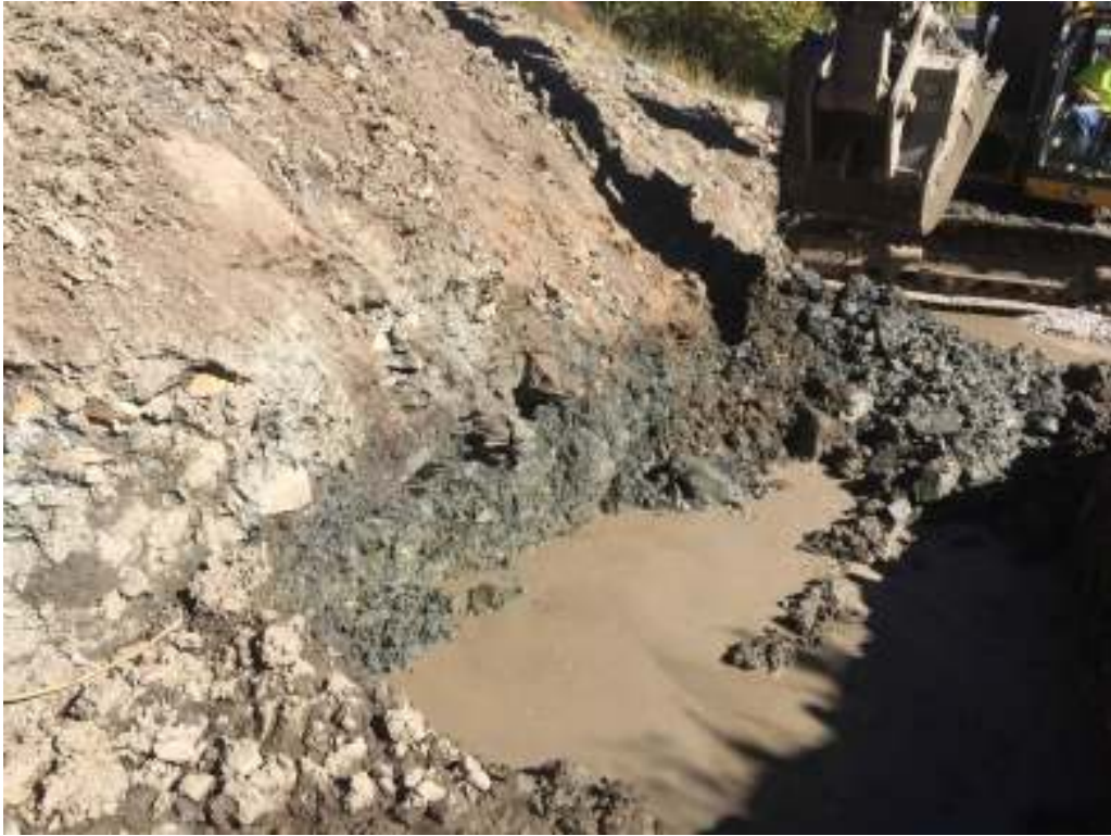
Photo 5 Cleaning trench stat 1+44 to 1+66, collapsing on sides, lots of water
