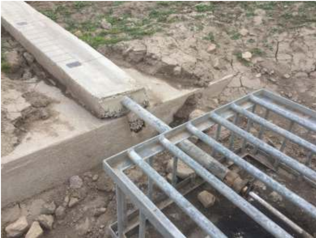
Photo 1 Grade beam/inlet structure overlap
