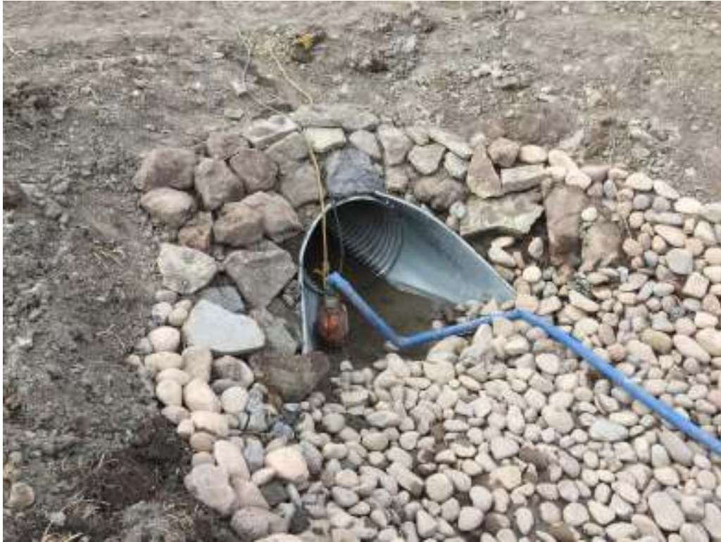
Photo 1 Outlet riprap/Cobble
