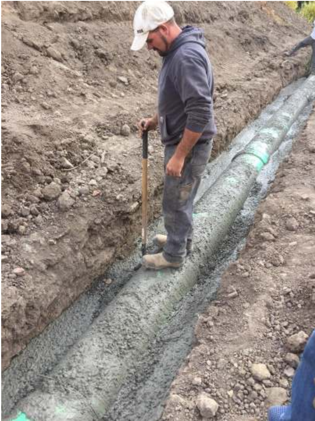
Photo 2 Shovel slicing flowfill under pipe
