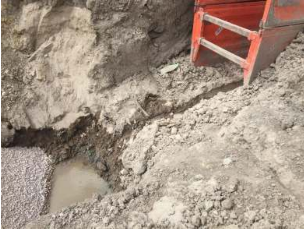
Photo 3 Gravel Placement near sta 1+44 - note lack of seepage from trench box area
