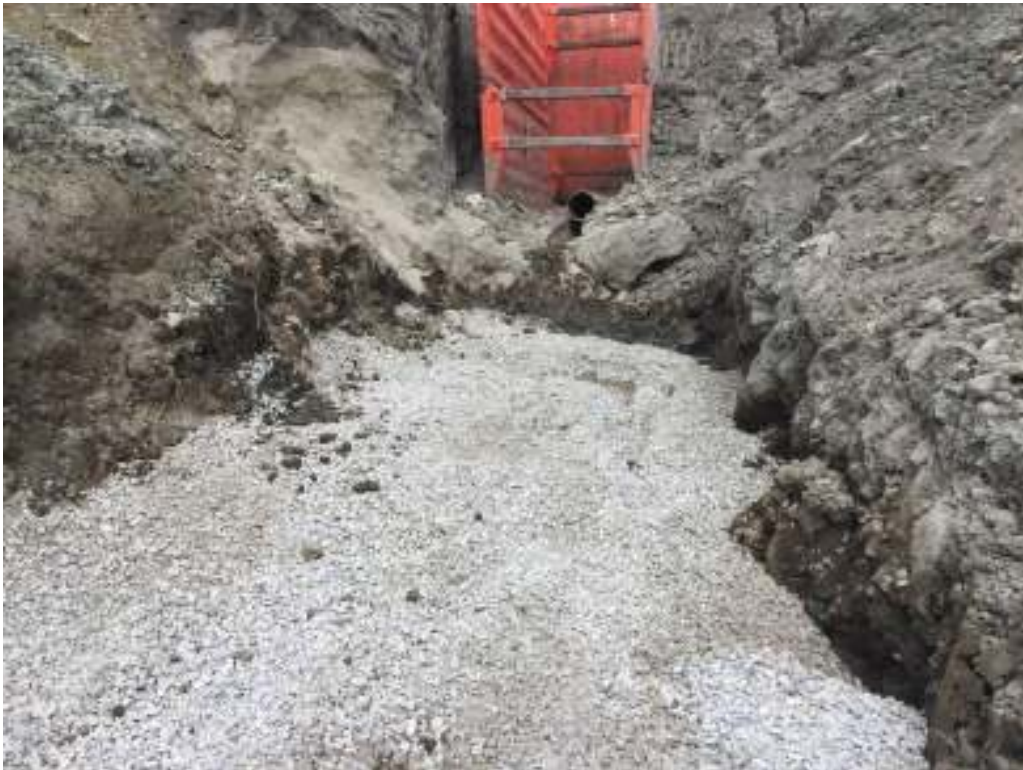
Photo 4 completed gravel placement sta 1+44 to 1+66
