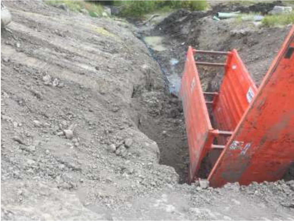
Photo 5 Trench boxes and near vertical adjacent slopes
