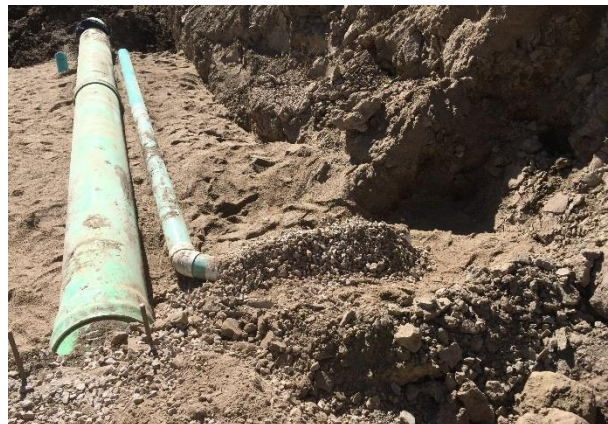
FIGURE 4 FILTER COLLAR DRAIN CONSTRUCTION
