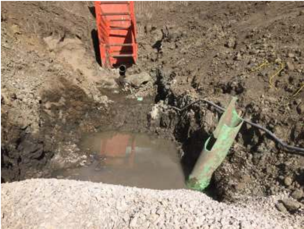
Photo 1 Dewatering Sump Install
