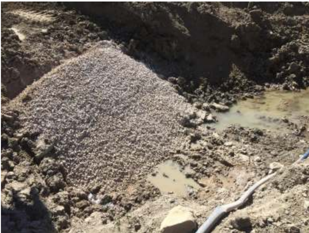
Photo 4 Initial Gravel placement near sta 1+66 (manhole)
