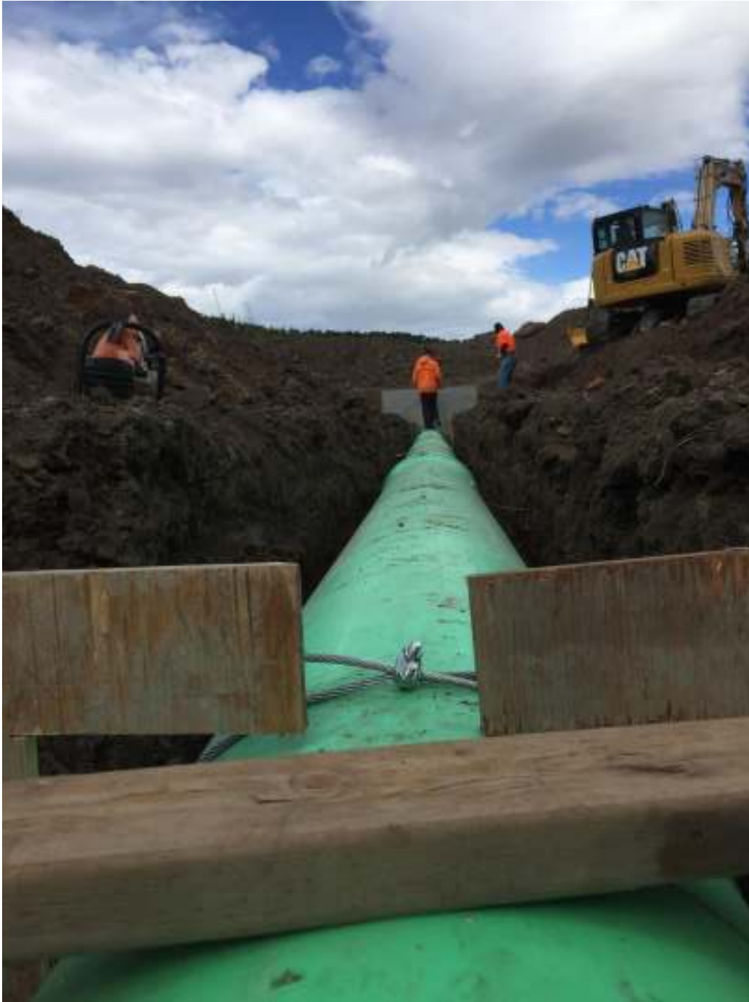
Photo 1 Pipe Ready for flowfill
