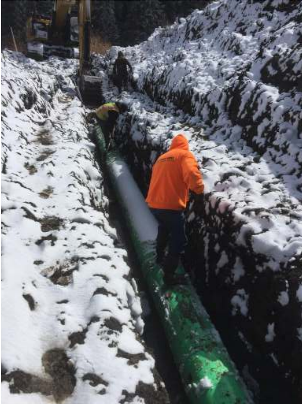
Photo 1 removing snow from pipe and trench
