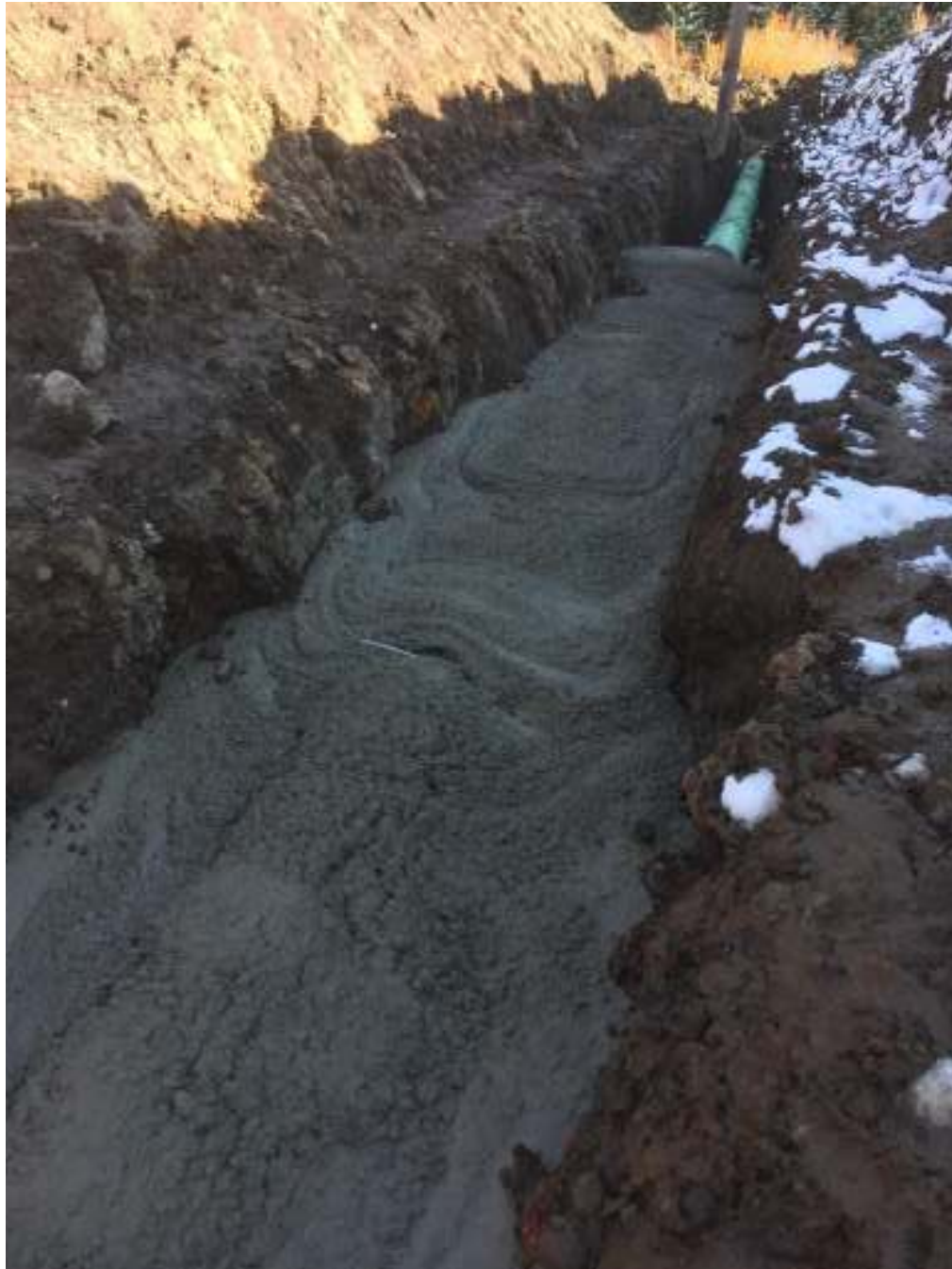
Photo 2 Flowfill Placement – looking downstream
