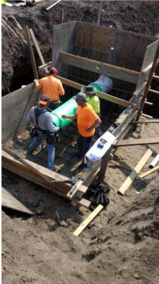
Photo 1 Inlet Structure Formwork
