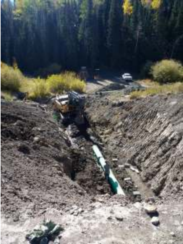
Fig 1: Crews setting pipe grade
