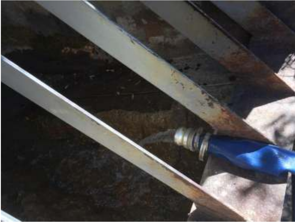
Photo 3 Dewatering Pump Discharge
