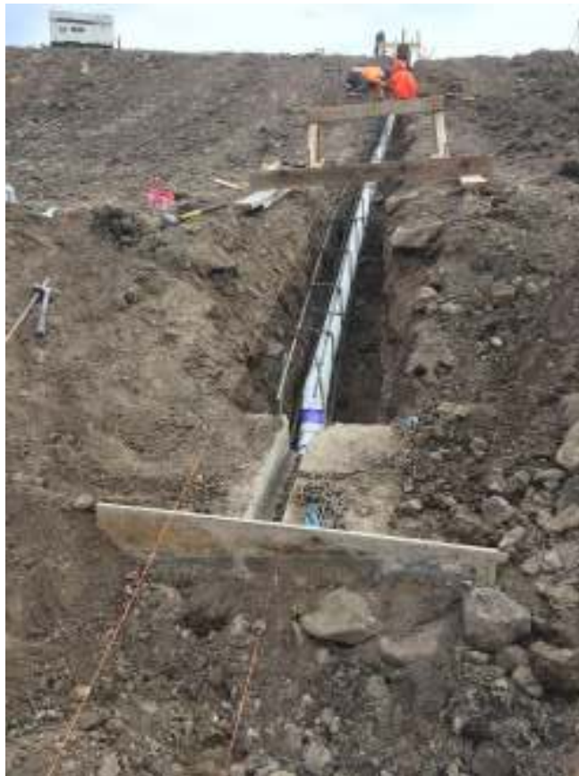
Photo 4 Starting Grade Beam formwork
