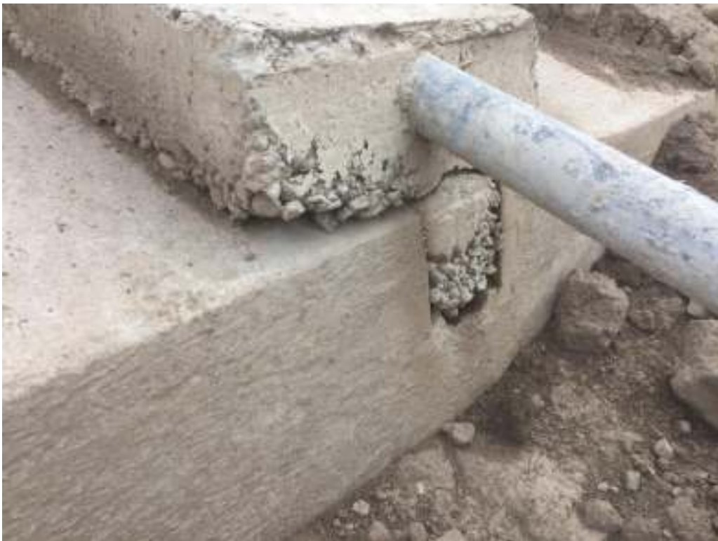
Photo 2 Grade beam/inlet structure overlap
