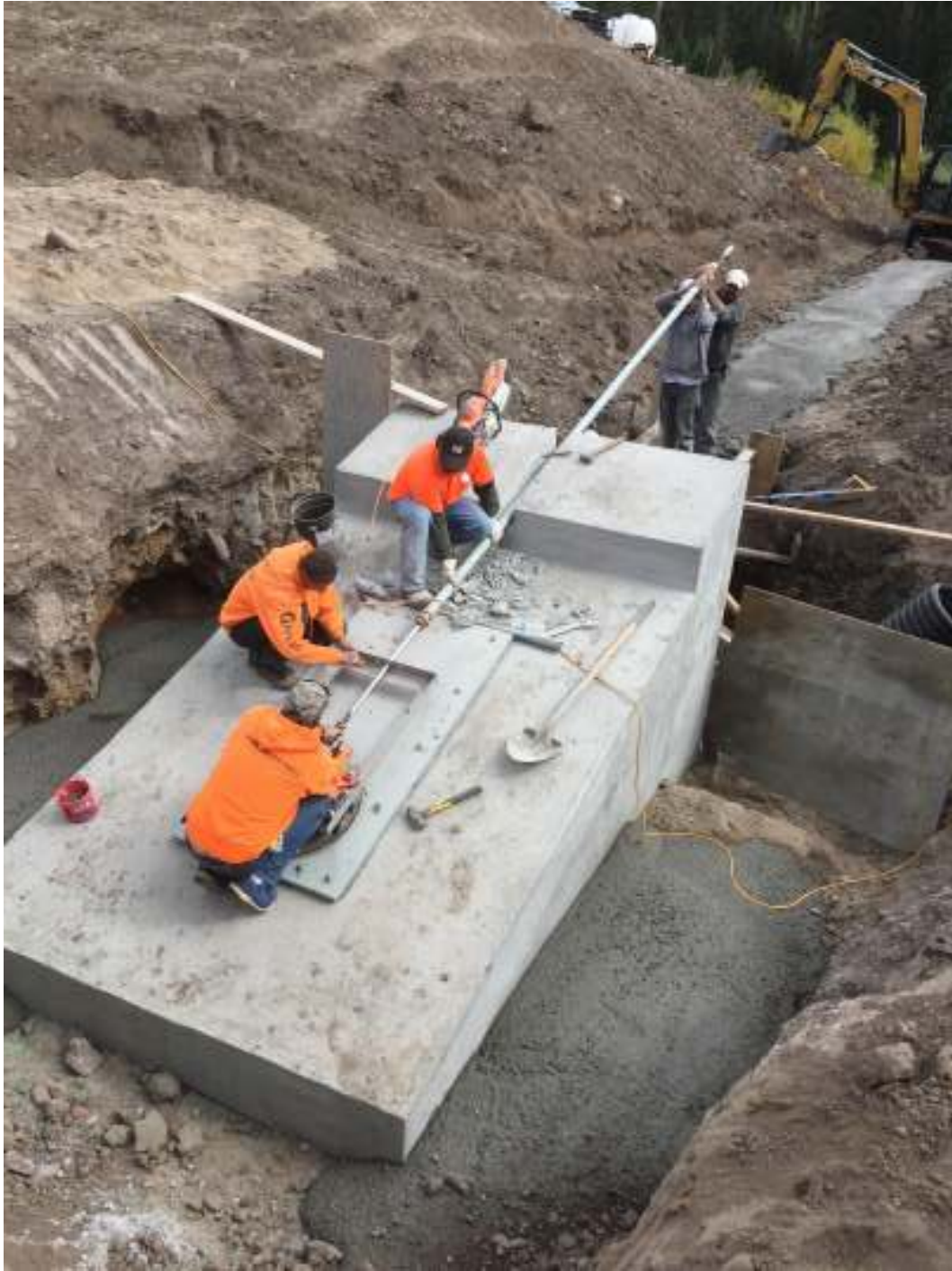
Photo 4 resetting gate stem
