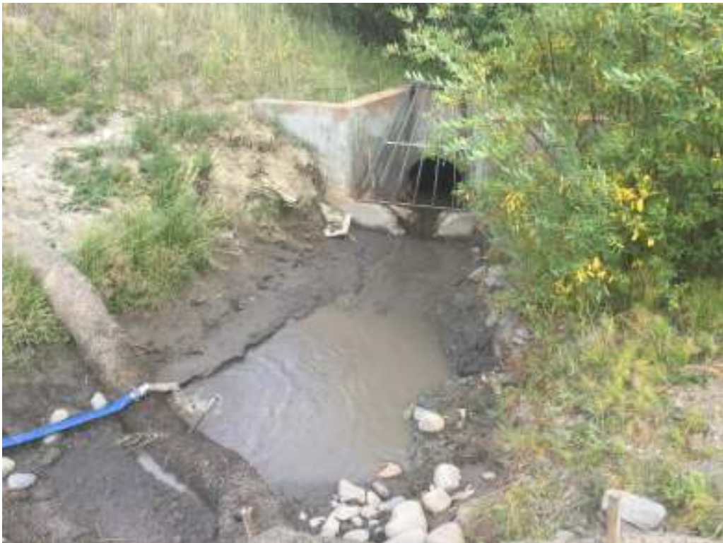
Photo 4 Dewatering pump discharge
