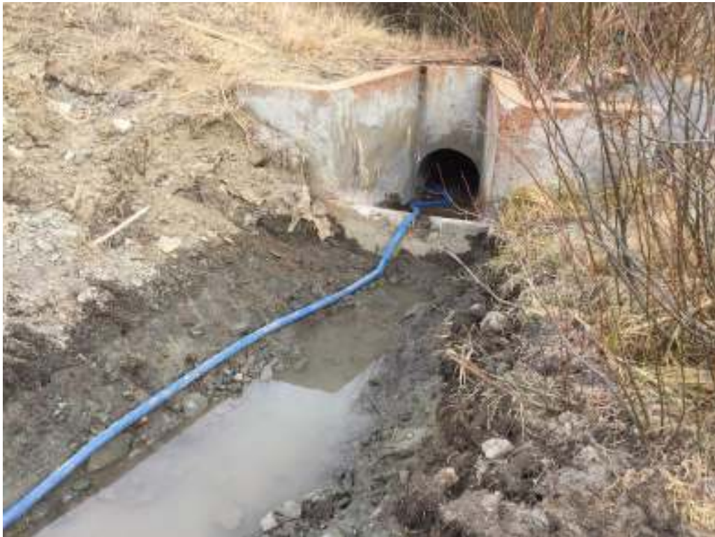
Photo 2 Existing 30" CMP Downstream, note concrete lip in front of pipe.
