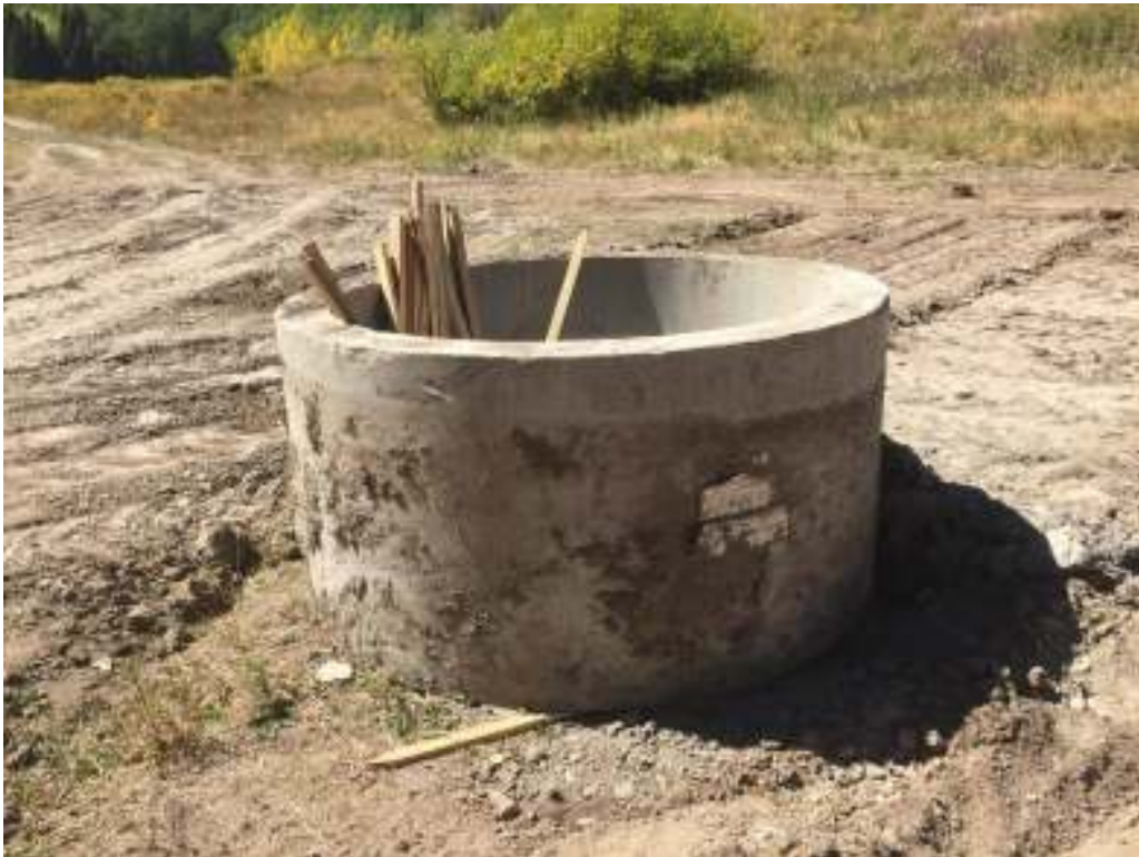
Photo 1 Upper Manhole section
