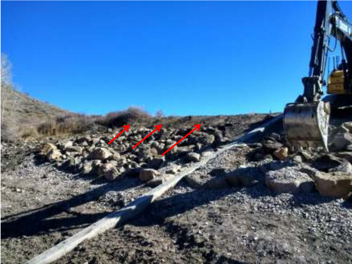
Figure 5: Crews Spreading Riprap Toward Crest
