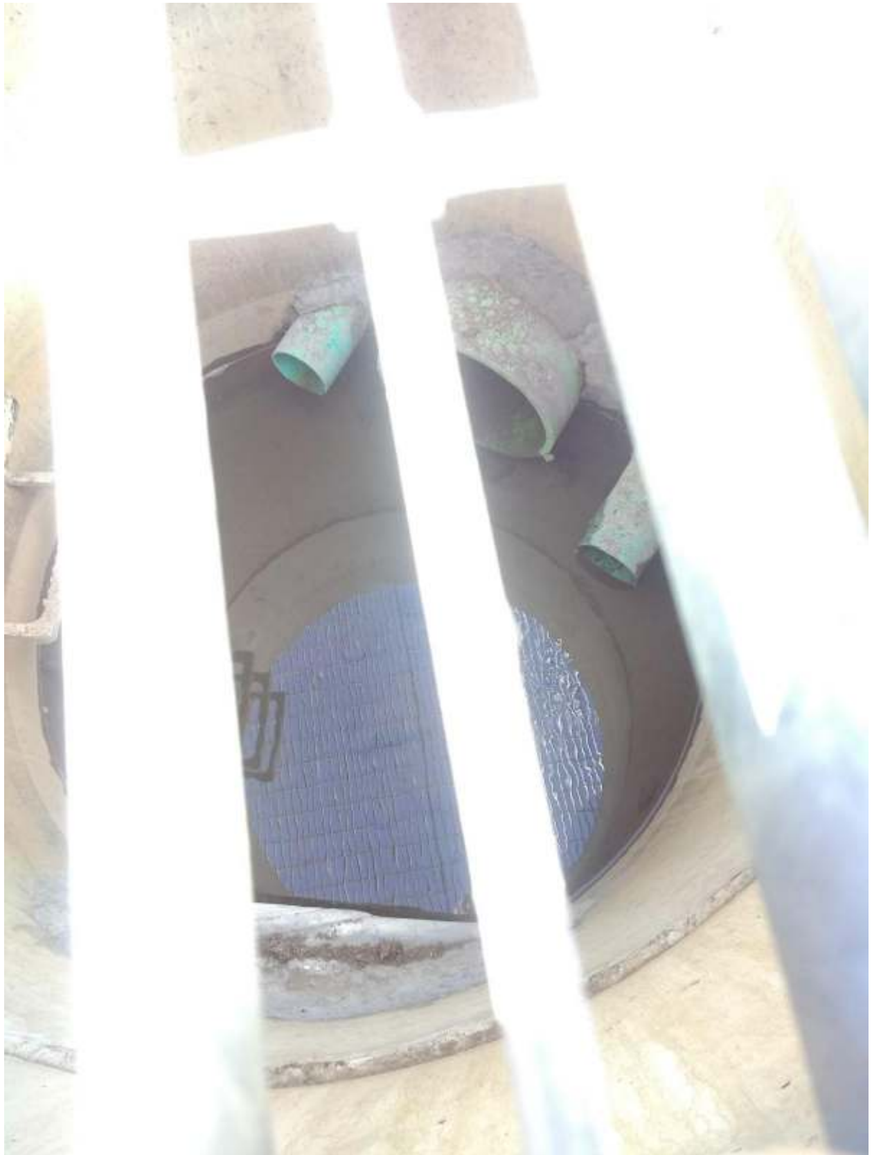
Figure 4: View Inside Downstream Manhole, Notice Water Levels Inside Pipes
