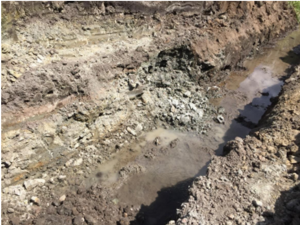
Photo 4 Seepage/Slump in Excavation
