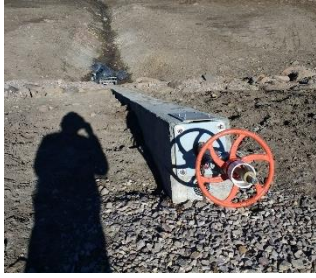
FIGURE 6 GRADE BEAM The concrete grade beam was poured in November of 2017. Due to the incorrect angle of the inlet structure concrete, discussed above, the lower end of the grade beam was poured overlapping a section of the inlet structure. This thin layer of concrete did not serve any purpose as the structural connection between the grade beam and the inlet structure was achieved through rebar on the back face of the inlet structure. This thin layer did not bond well to the inlet structure and in 2018 it was noted that this concrete had cracked near the back edge of the inlet structure. Since this section did not serve any purposed it was sawcut near the back edge of the inlet structure and removed. The staff gage was then marked below this point with a demo saw.
