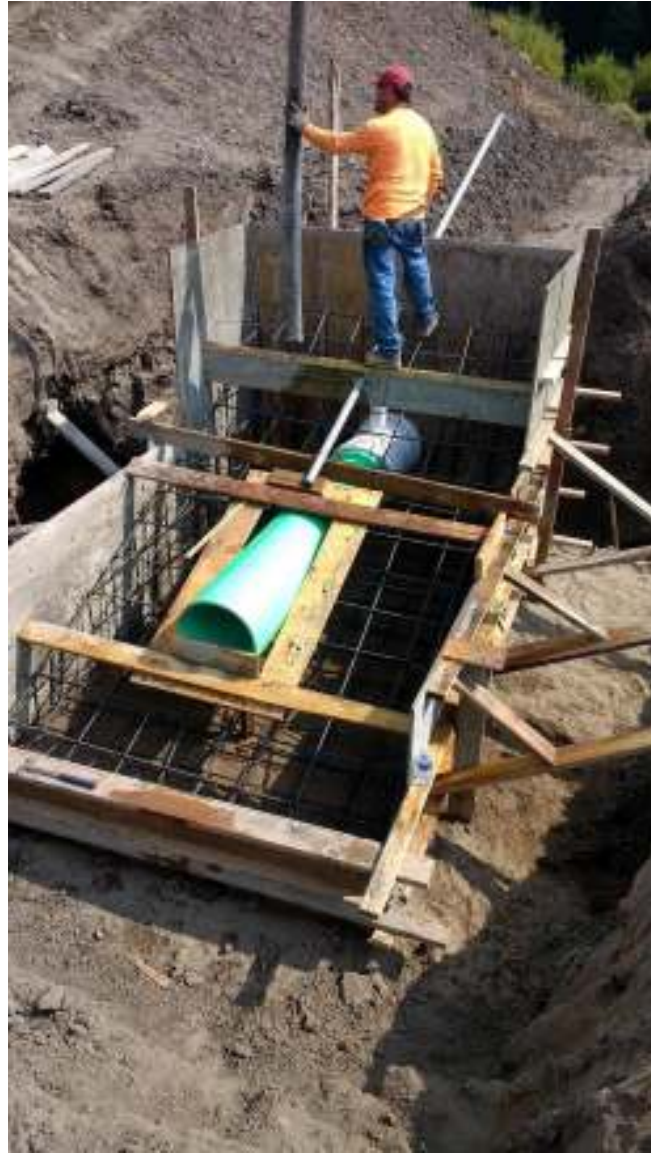
Photo 2 Beginning Concrete Placement
