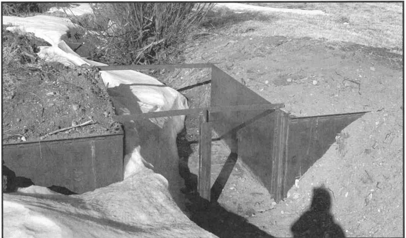
Photos of backfilled structure. 1/4" steel walls and floor with 1/4" x 2" x 2" angle iron reinforcement and check board slots. Dimensions and elevations are as designed. Welds and construction are good. Compaction is present and installation is good. Anodes are in place - (2) 32lb.
