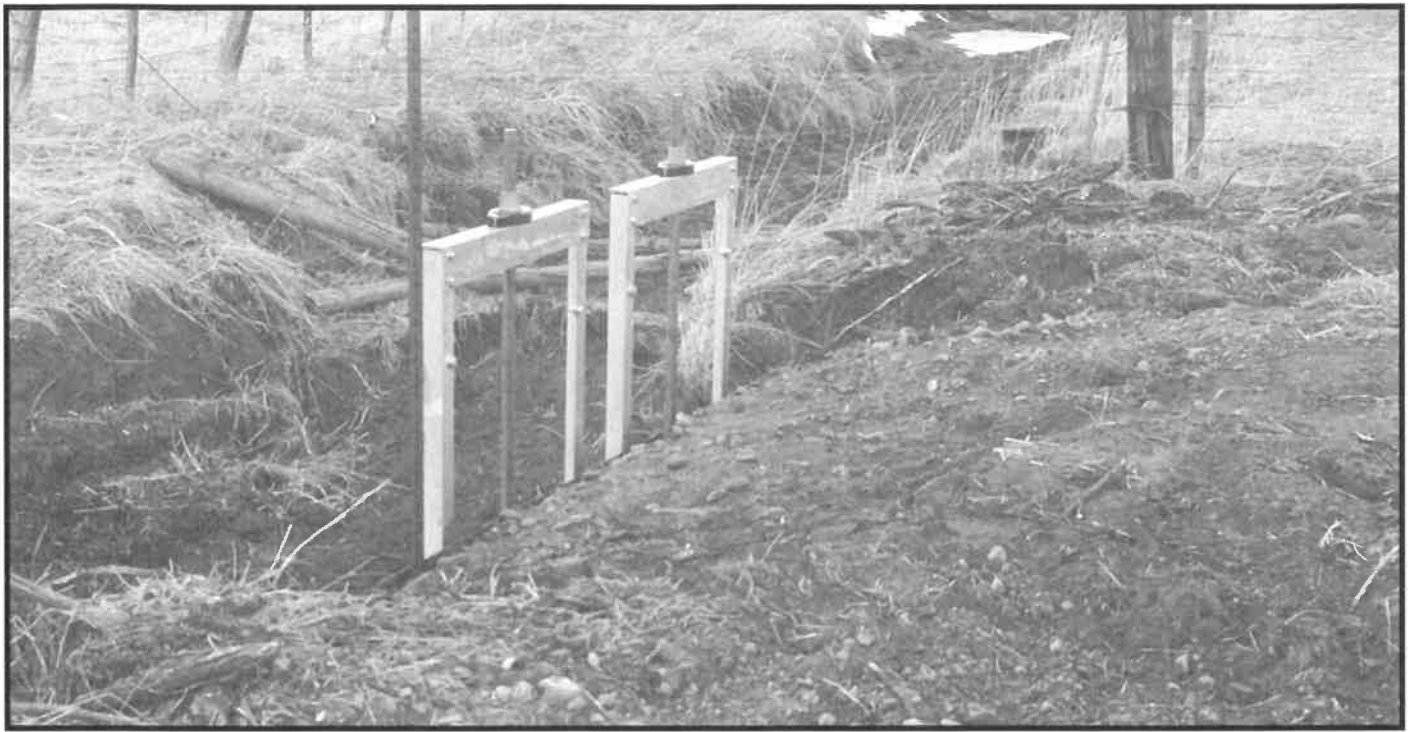
Photos of backfilled structure. Each pipe is 30" x 20' ADS N12 pipe. Gates are Fresno, flat back 30" cast iron slide gates with 5' frames. Compaction is present and installation is good. Compacted material along pipes, under top fill material is 3/4" crushed road base.
