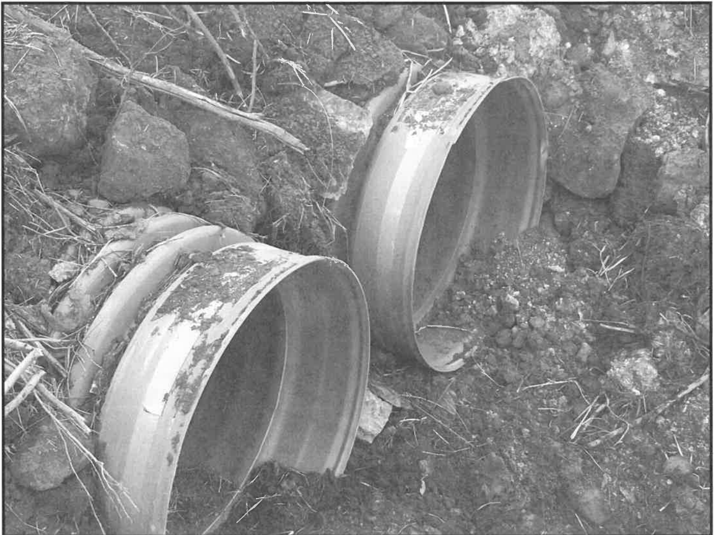
Photos of backfilled structure. Each pipe is 30" x 20' ADS N12 pipe. Gates are Fresno, flat back 30" cast iron slide gates with 5' frames. Compaction is present and installation is good. Compacted material along pipes, under top fill material is 3/4" crushed road base.
