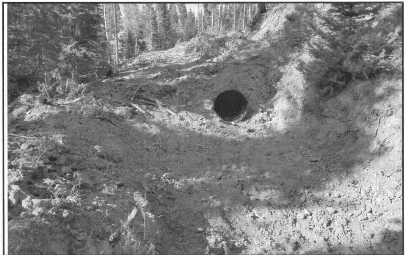
Completed Length = 440 feet of 30" diameter ADS N12 Pipe with adequate cover.
